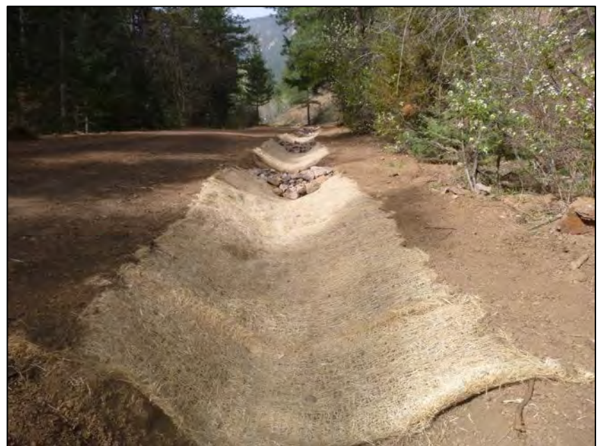
Figure 4. Images of check dam installation and erosion control matting.
