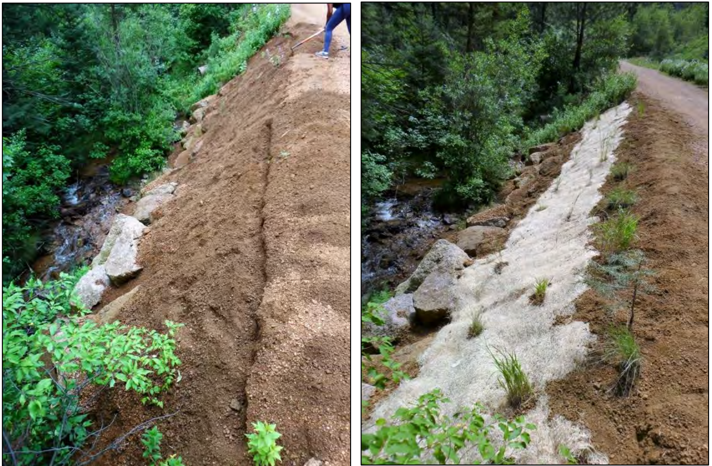
Figure 2. Before and after images of erosion control matting installation and native vegetation transplants.
