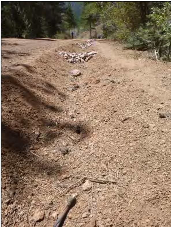
Figure 4. Images of check dam installation and erosion control matting.
