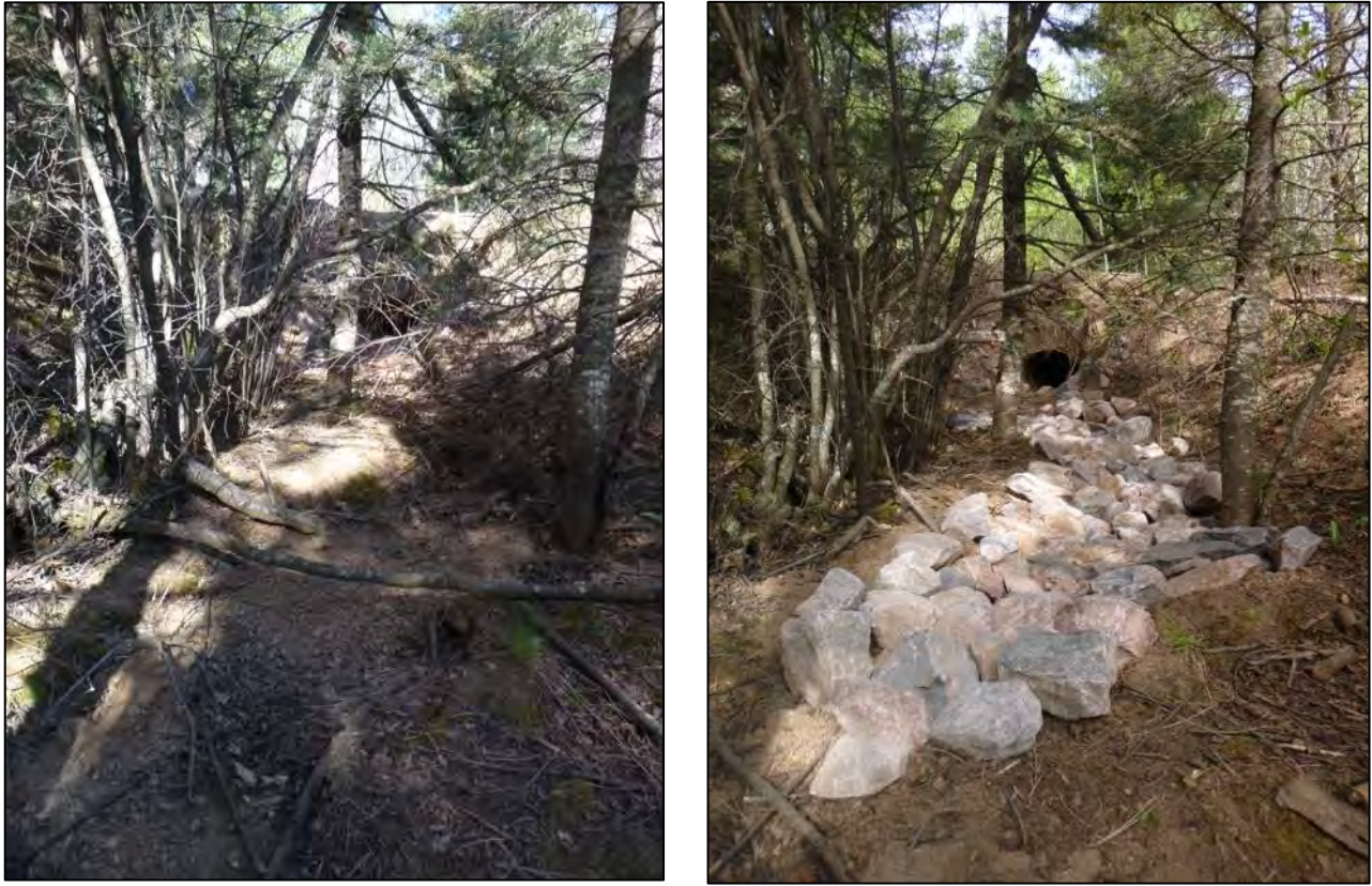
Figure 5. Before and after images of drain installation below culvert.
