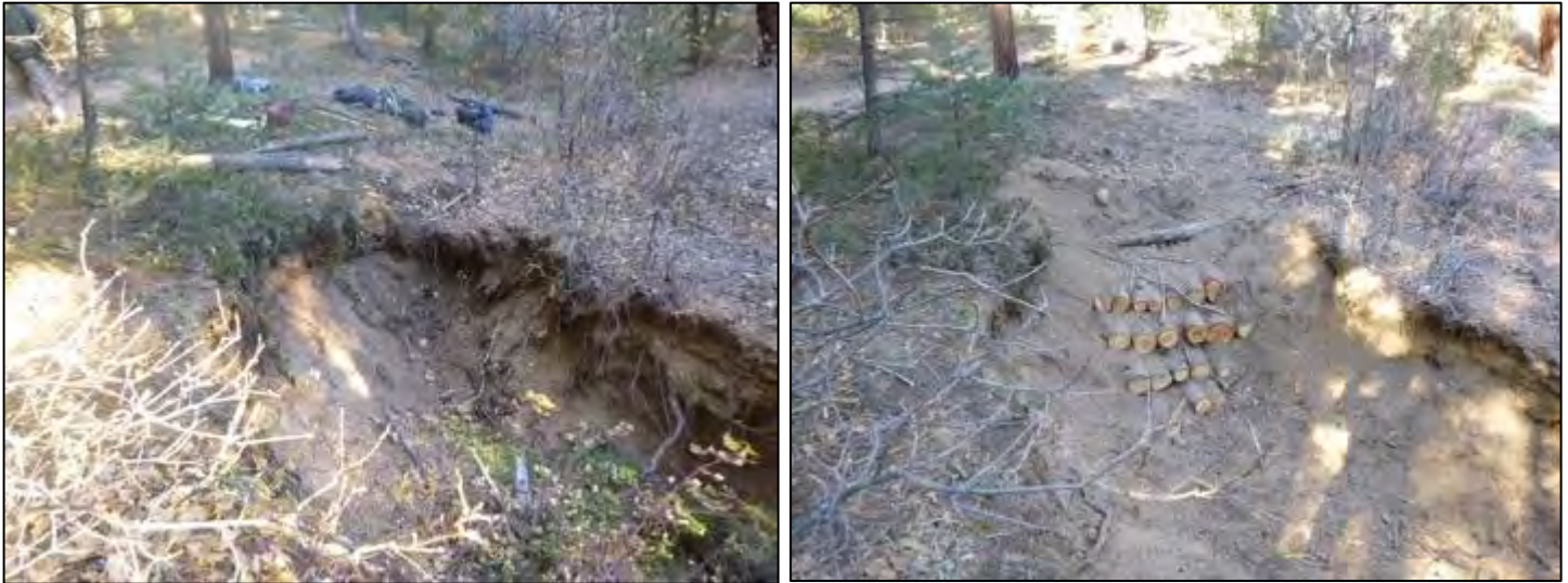
Figure 1 (above). Before and after images of a headcut treated with log stepfall structure.
