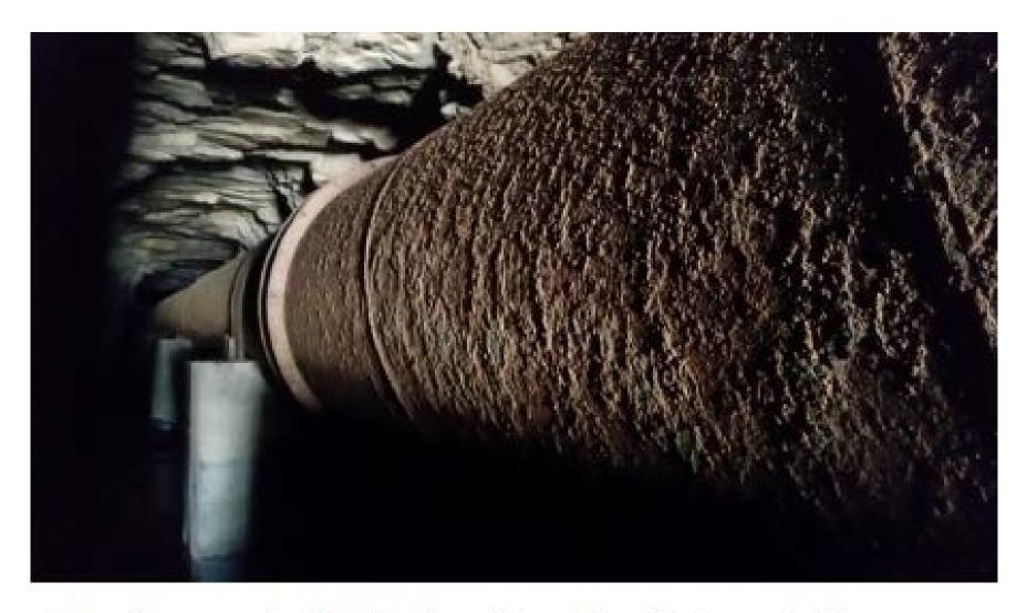
Heavily corroded/pitted section of outlet conduit.
