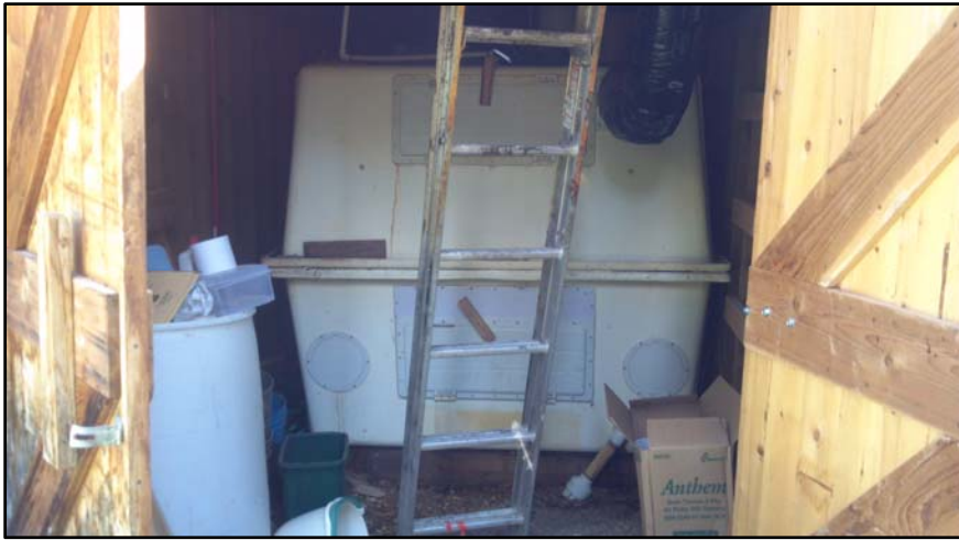
FIGURE 5. THIS IS A PHOTO OF THE FULL VAULT. EVEN THE BLACK VENT PIPE IN PHOTO RIGHT IS FULL OF HUMAN WASTE THAT HAS NOT DECOMPOSED.
