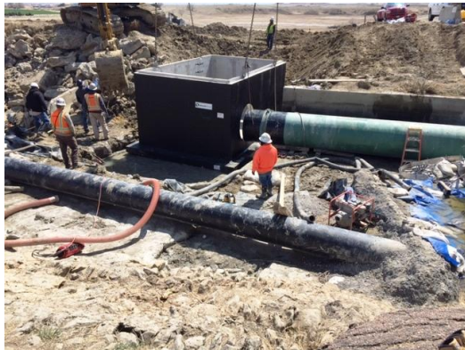
Placement of large vault in the Outlet Canal used to house the valves that divert water to Pump Station No. 1.
