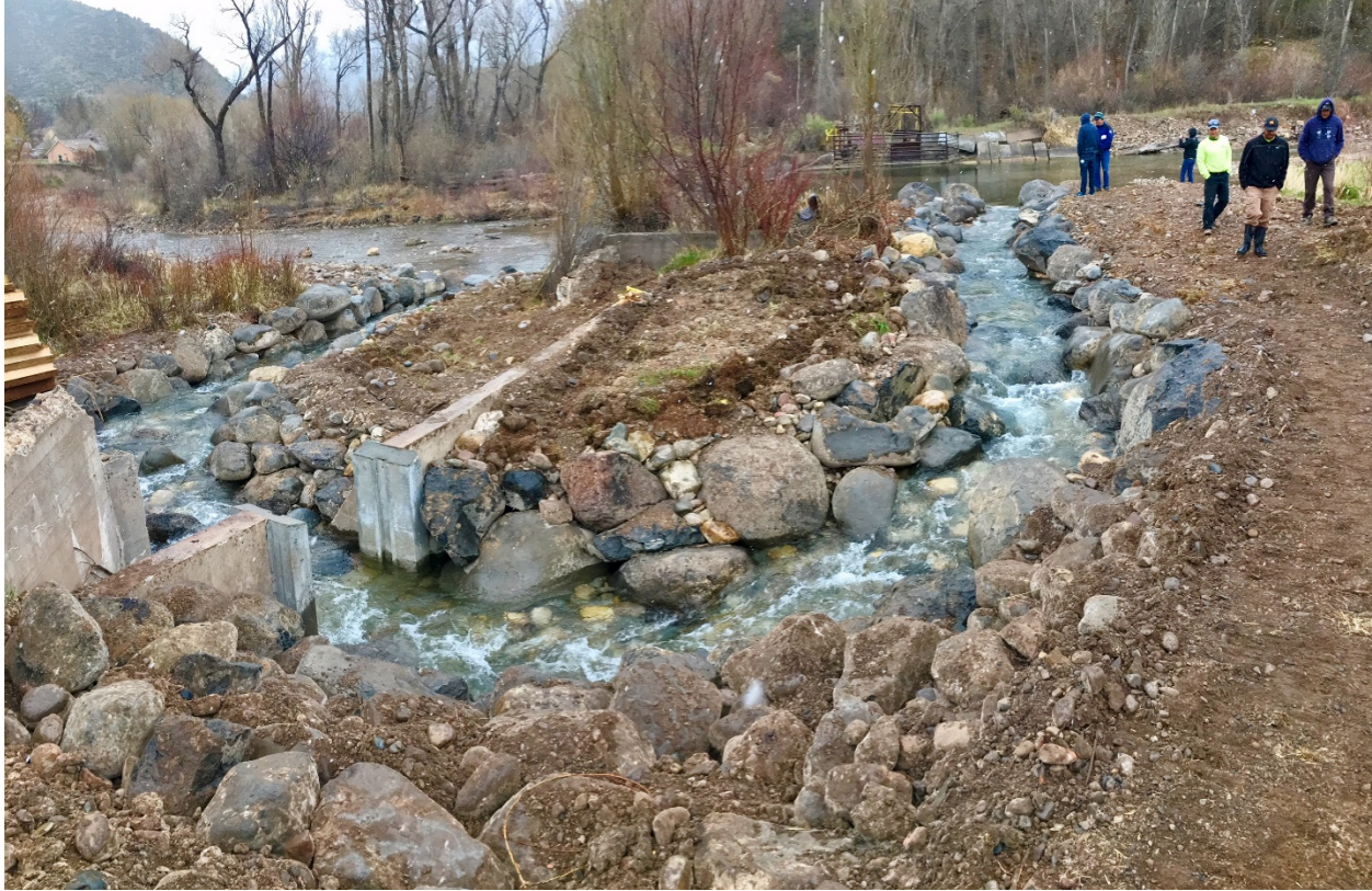
Final inspection of the Ware and Hinds Fish Bypass channel by TU and CPW personnel.
