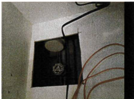
METER BEHIND WALL – Required access panel
