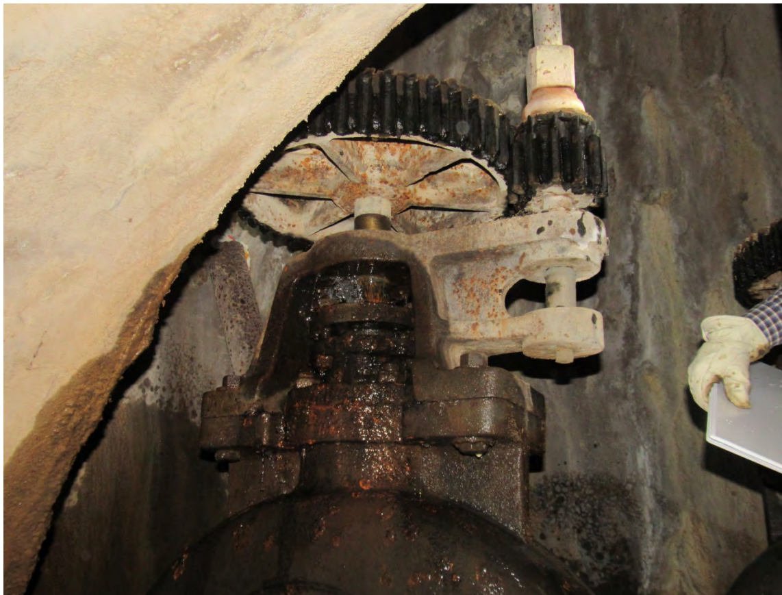
Water leaking from top of gate valve No. 1. Taken 3/13/17
