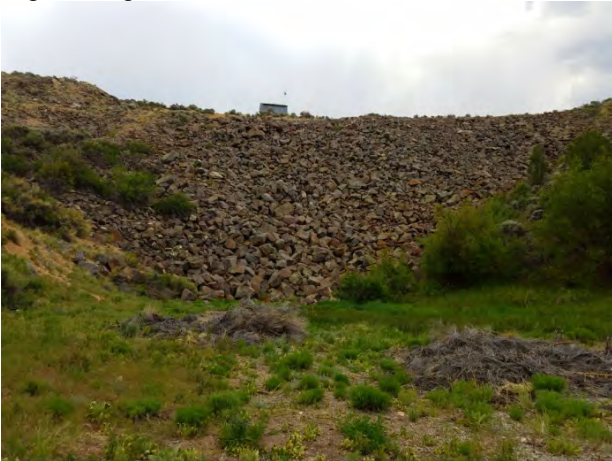
Photo 4 – Overview of downstream slope and toe. NOTE: slash piles from clearing brush from the downstream toe last year.
