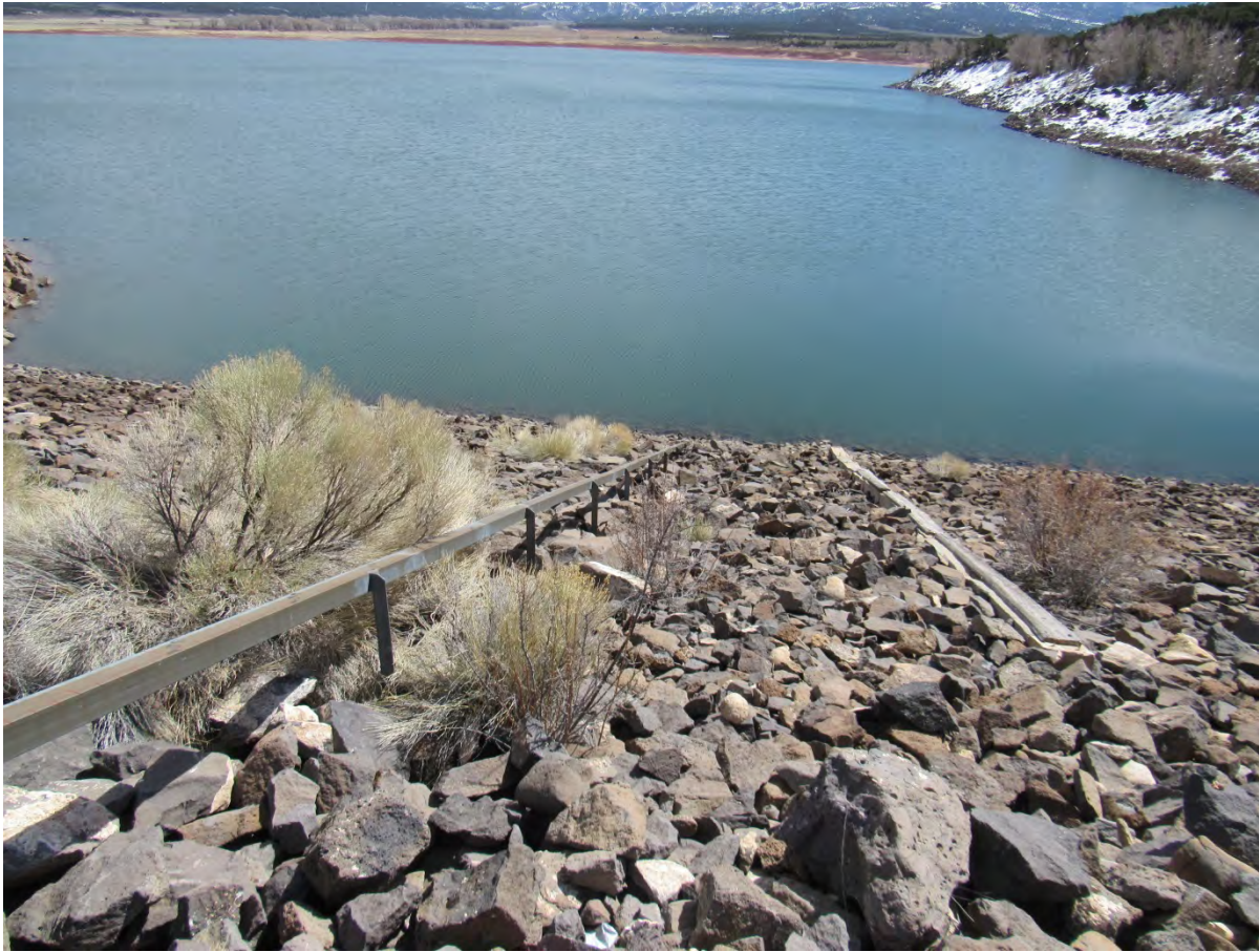
Upstream slope of dam and reservoir elevation staff gauge(s). View taken looking east. Taken 3/13/17
