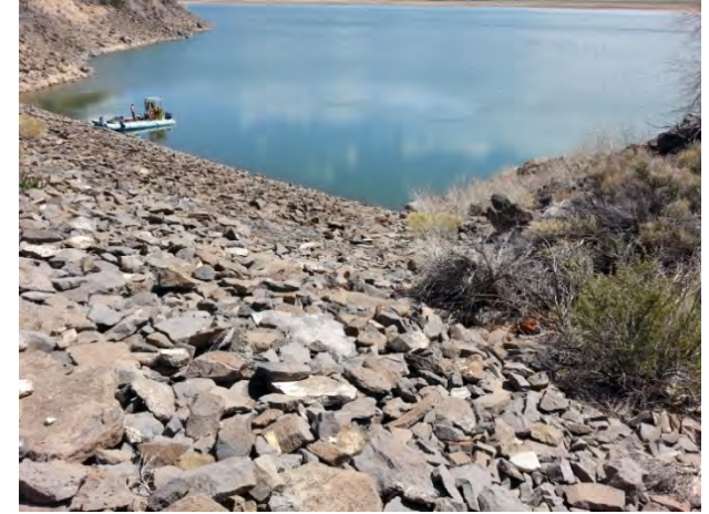
Photo 3 – Looking down the upstream, left groin/abutment contact. No signs of distress observed. Would aid visual inspection to remove brush from the dam's groins.
