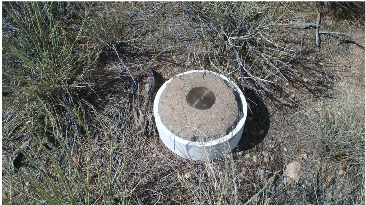
Typical concrete survey benchmark location. Taken 3/13/17
