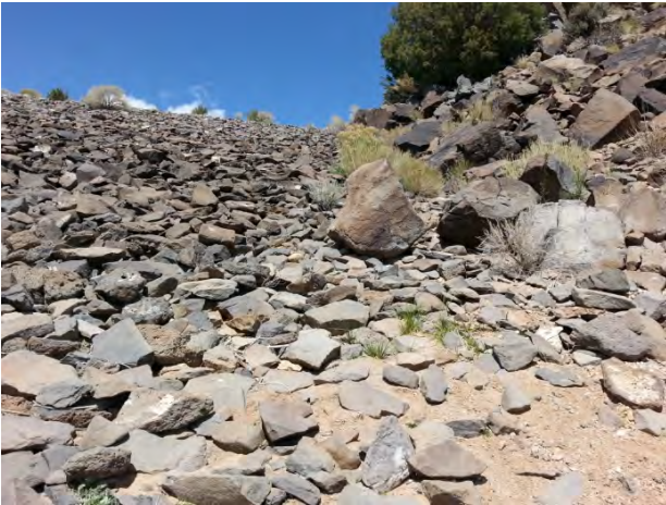
Photo 4 – Looking up the upstream, right groin/abutment contact. No signs of distress observed.
