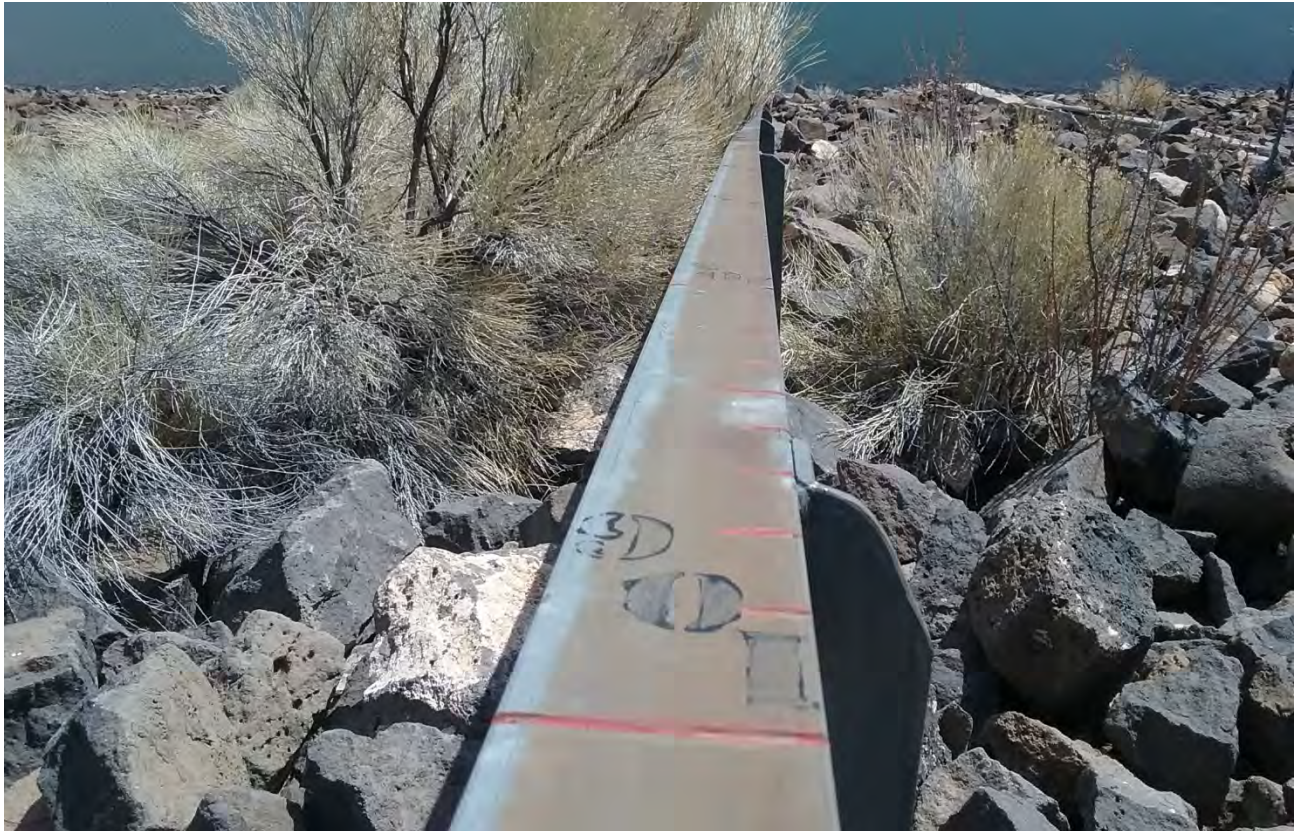
Concrete staff gauge on upstream slope of dam. View taken looking east. Taken 3/13/17
