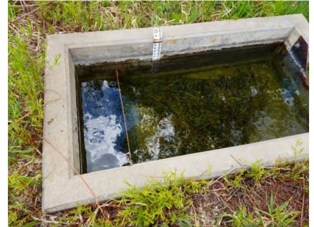
Photo 6 – Toe drain weir box. .
