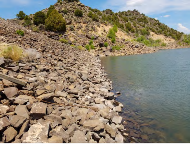
Photo 1- Upstream slope, slightly left to right along the water line at GH 65.8 ft.
