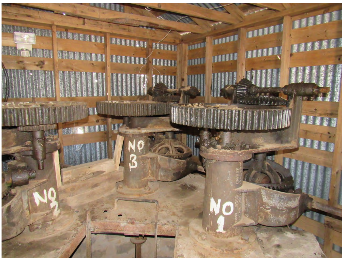
Outlet works gate valve controls inside control house. Taken 3/13/17
