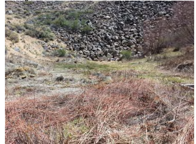
Photo 6 – Downstream toe of the dam after owner cleared brush.
