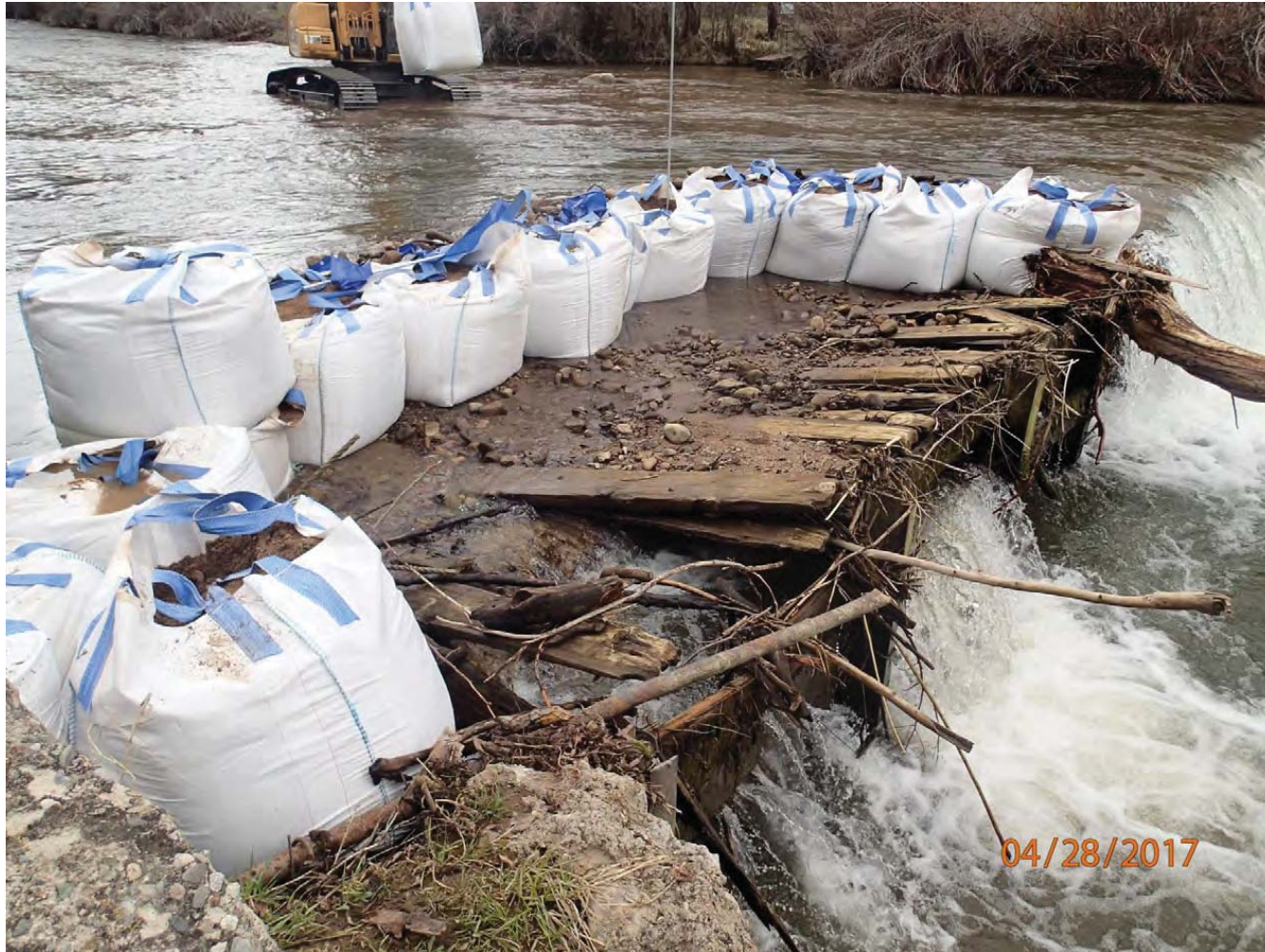
Photo 2: Florida Canal Diversion Structure - Emergency Repair
