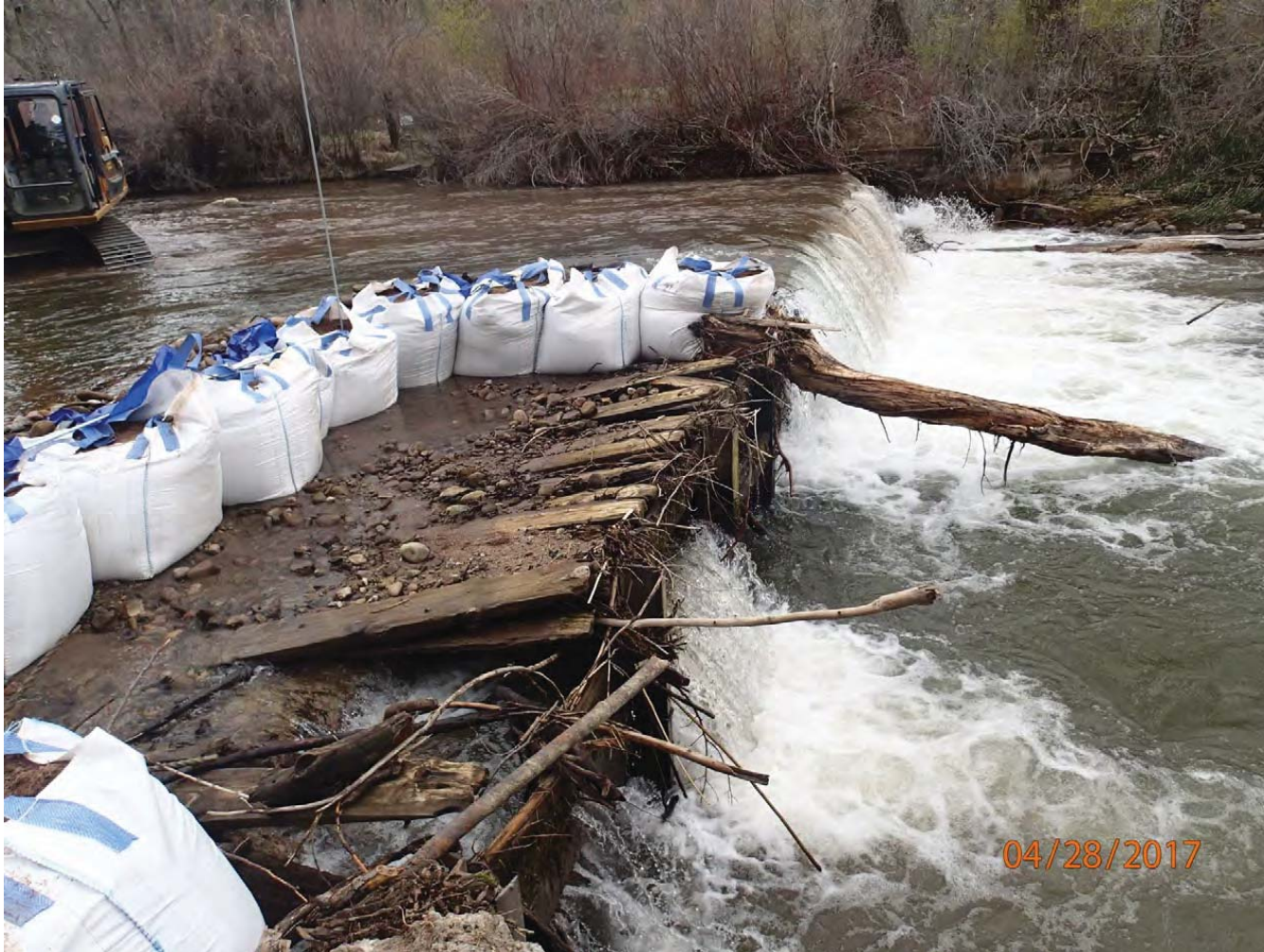
Photo 3: Florida Canal Diversion Structure - Emergency Repair 2
