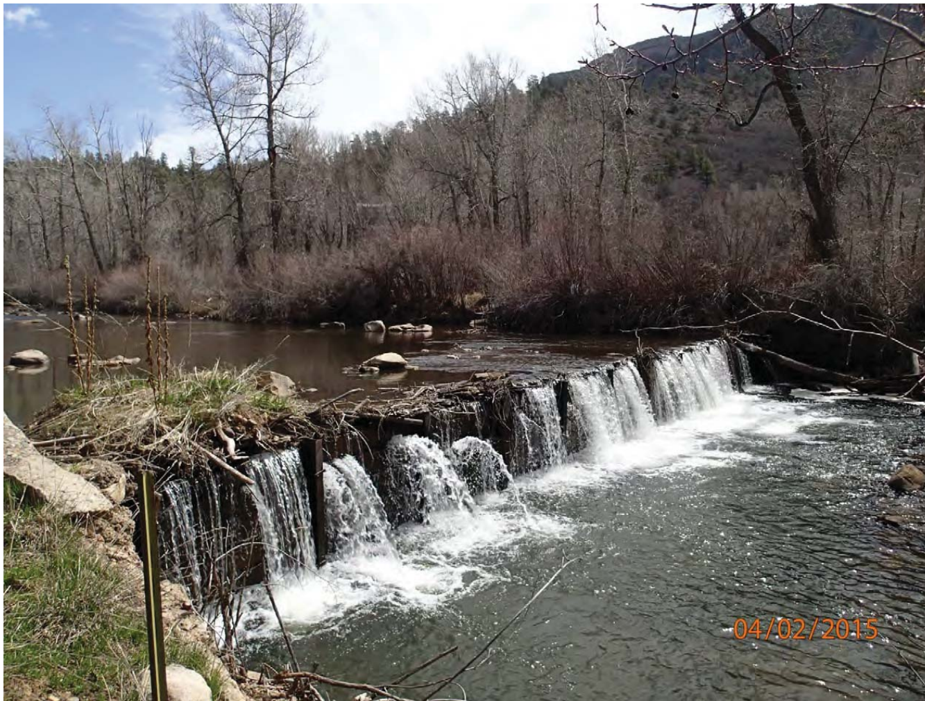
Photo 1: Florida Canal Diversion Structure - Pre-Failure
