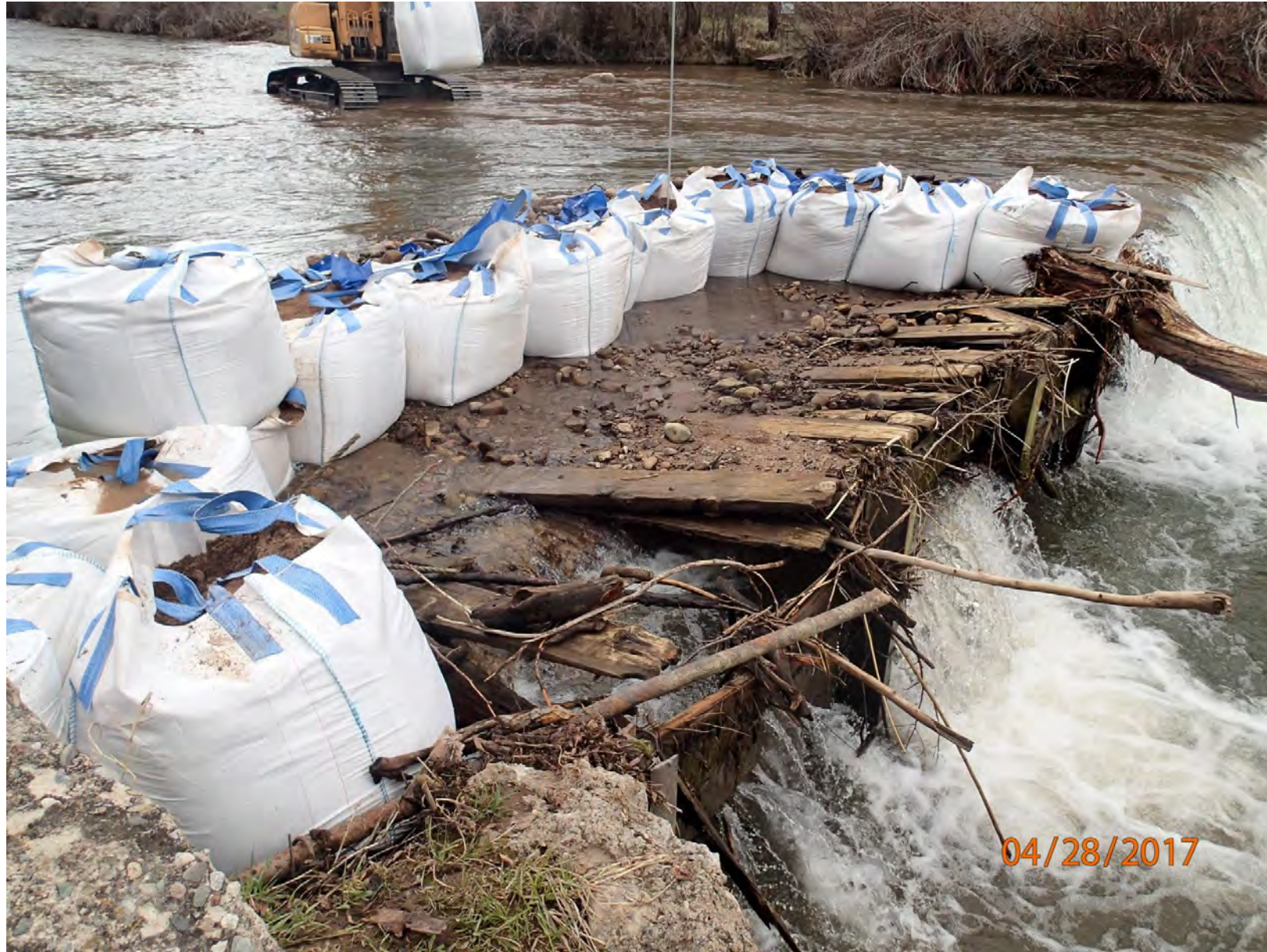
Photo 2: Florida Canal Diversion Structure - Emergency Repair
