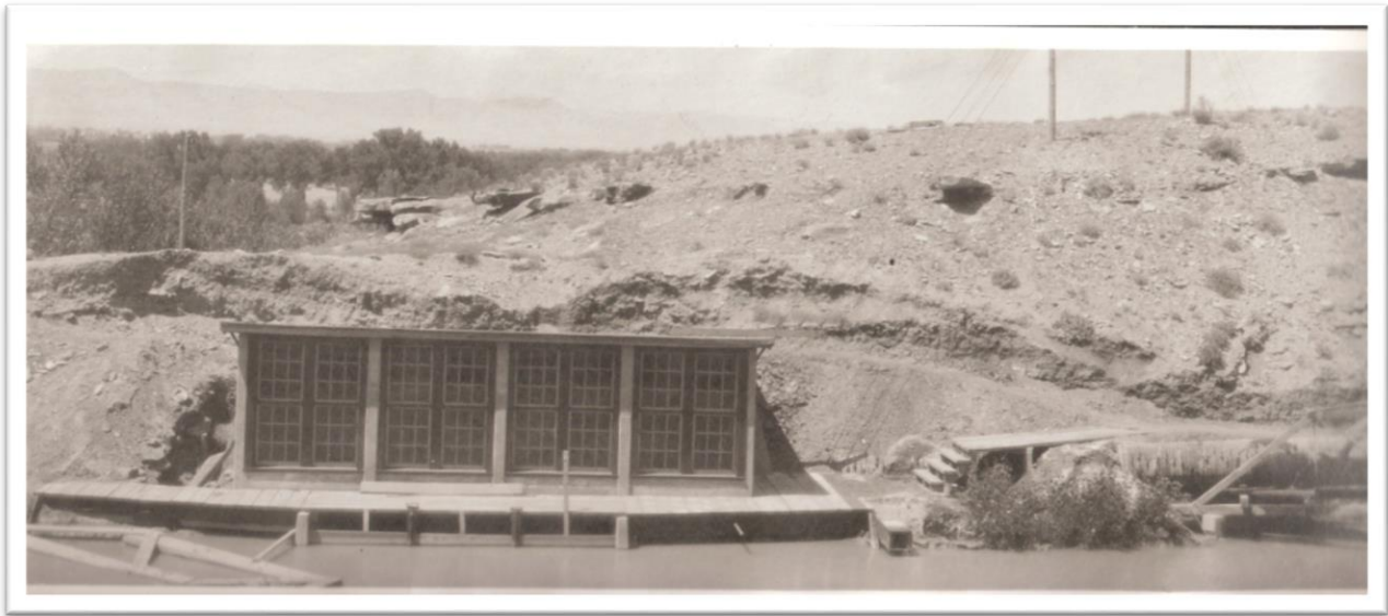
Pumping Plant Intake - Early Completion
