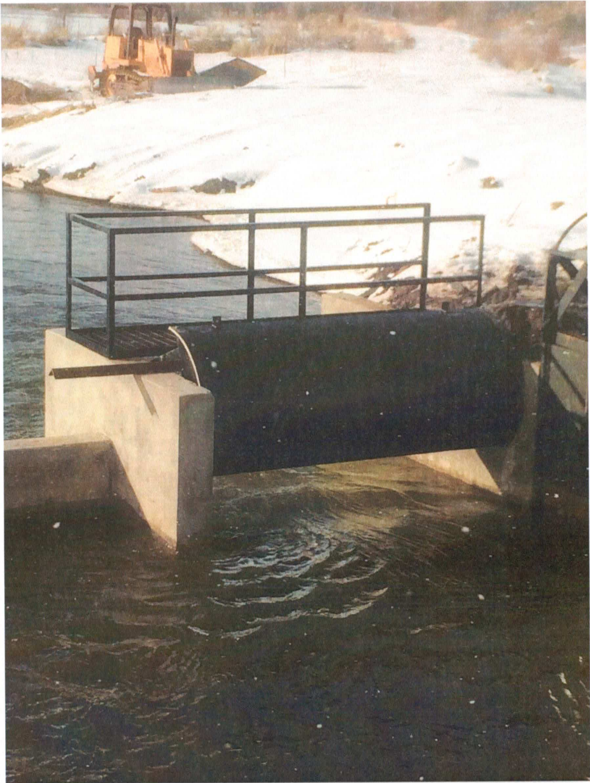
Eastbend radial gate installation
