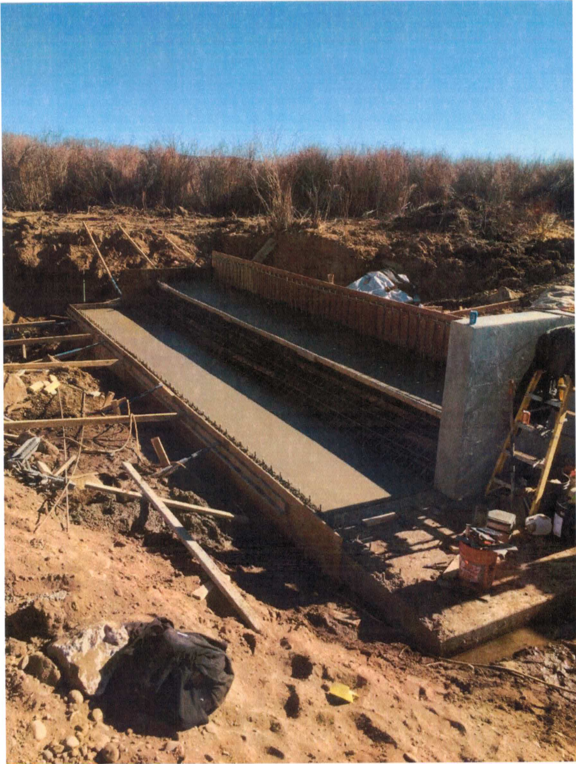
3/4/2016- Mr. Watters has completed all of the necessary concrete work at the confluence location. The final pours were for the Ephraim's core. He is in the process of installing the metal sheet piling for the wings of the Ephraim, building and installing the radial gate for the Sanford, and rehabilitating the superstructure of the Sanford diversion gate to accept automation.
