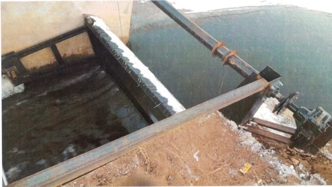
Radial gate with winch mechanism at the Sanford site.
