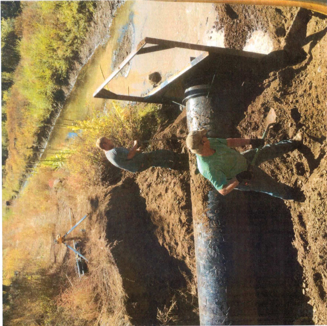
Workers install the channel Sluice structure near the Sanford Diversion
