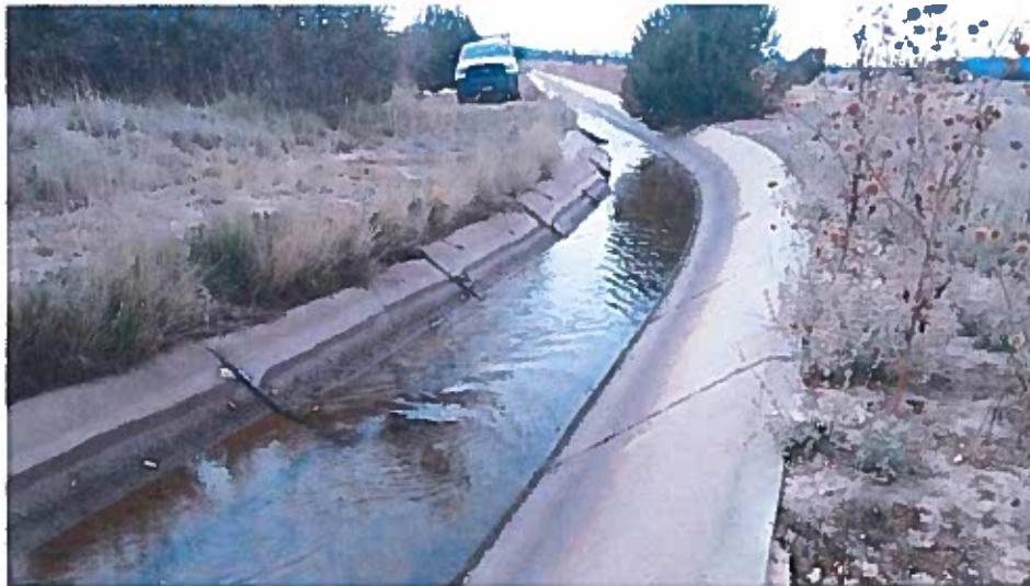
Left side of canal section fractured at base and slumping into canal bottom. Right side of canal lining remains in good condition.
