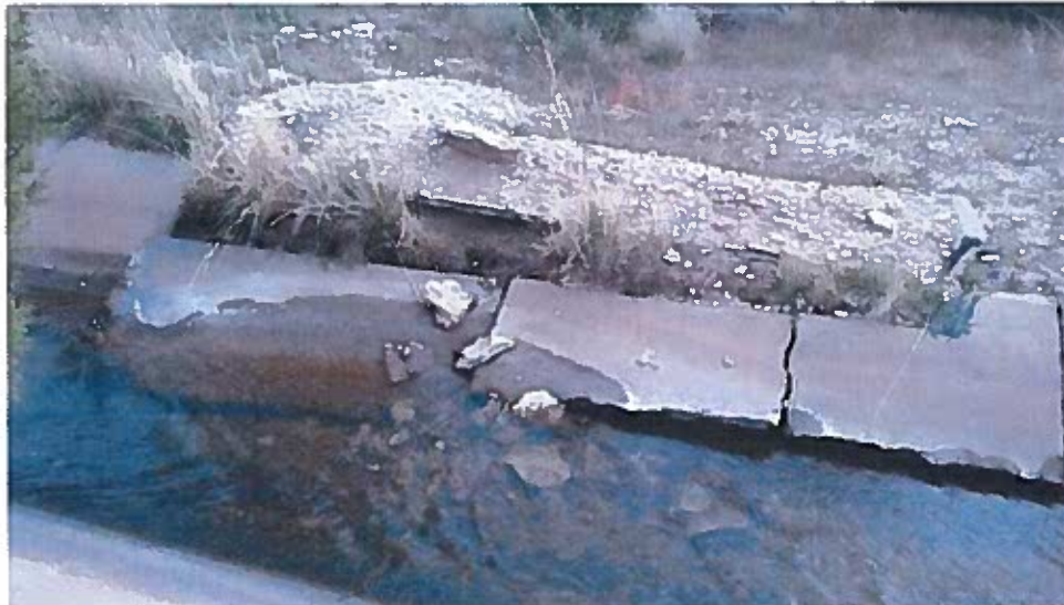
Individual canal concrete lining sections fully separated from the bottom of the canal. Increasing ditch transit losses and sediment load while also reducing canal capacity.
