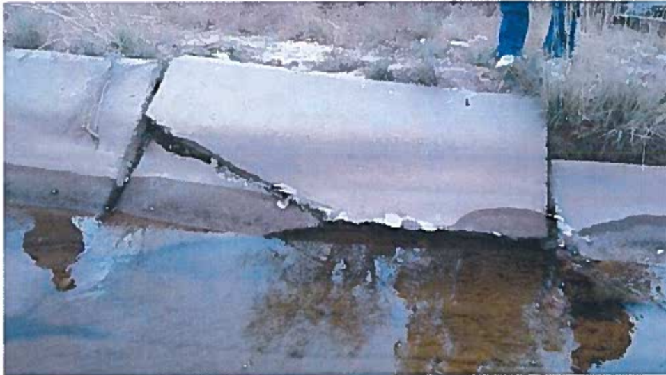
Fully failed canal lining section.
