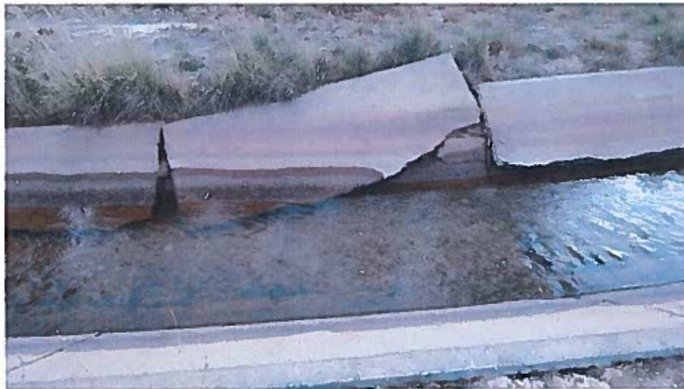
Fully failed canal lining section.
