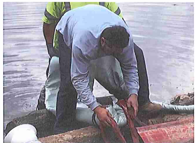
Starting Liner Installation at Inlet
