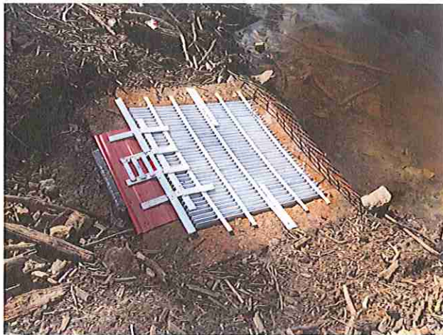
New Trashrack After Installation
