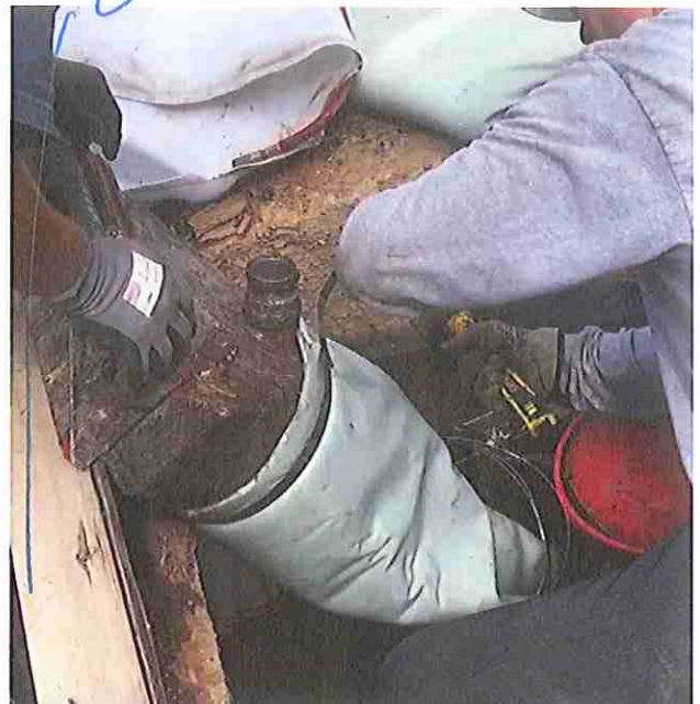
Connecting Steam Applicator Into Upstream End of Outlet Liner – Note New Headgate
