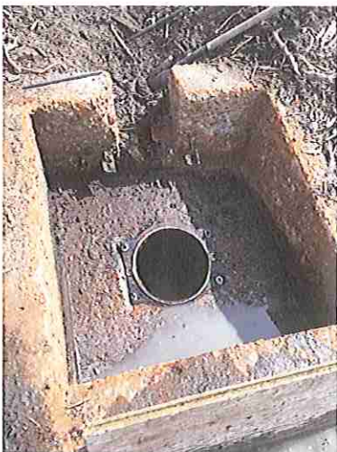
Inlet Basin After Removal of Old Headgate
