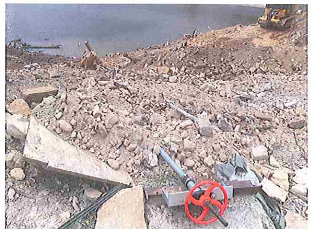
Backfilling New Gate Stem
