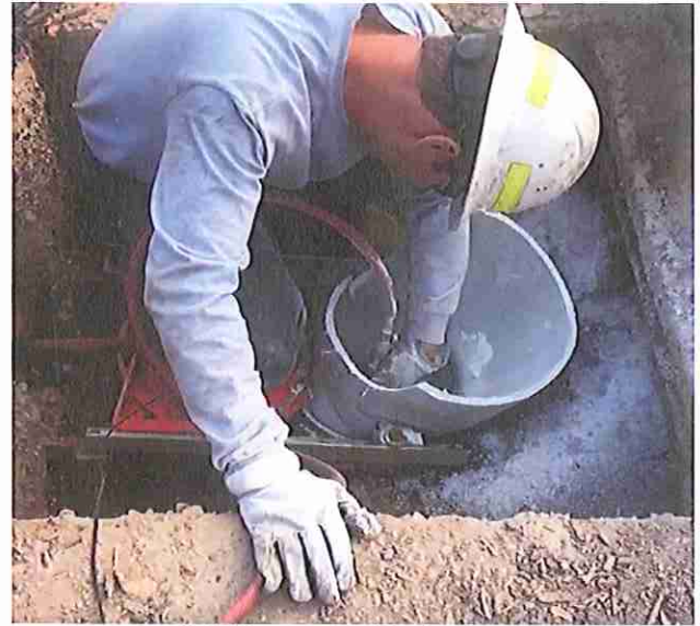
Cutting Off Upstream End of Outlet Liner
