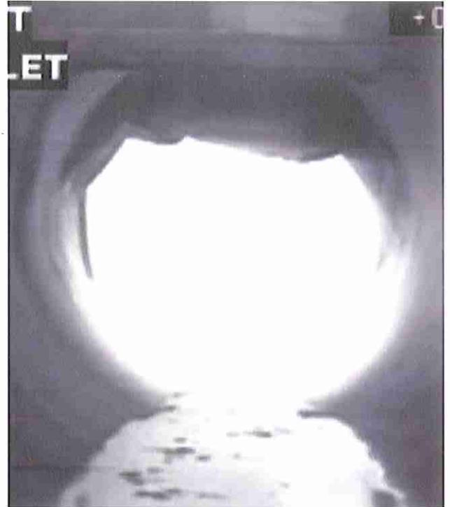
Upstream End of Lined Outlet
