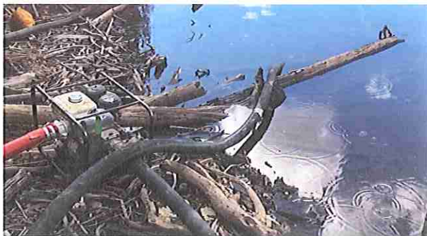
Pumping Reservoir Down Prior to Liner Install
