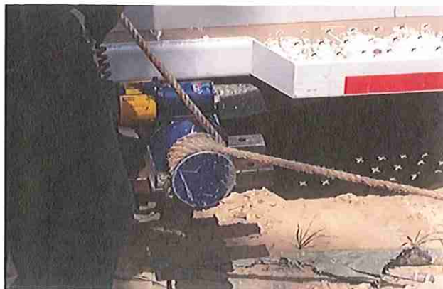
Cathead Winch Used To Pull Liner
