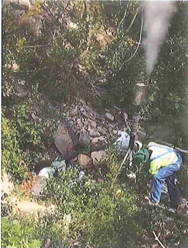
Releasing Steam From Downstream End of Outlet Liner and Verifying Temperature Has Reached 180 degrees F
