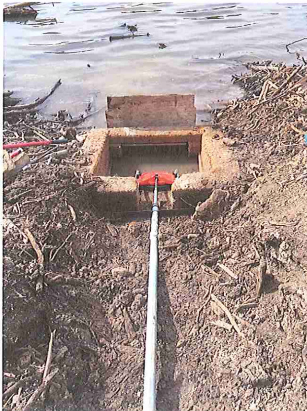
New Gate Stem and Headgate After Installation
