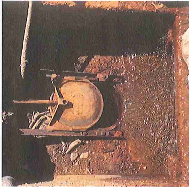
Old Headgate Prior to Removal
