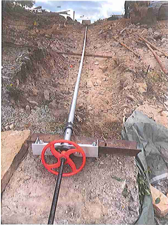
New Gate Stem and Wheel After Installation
