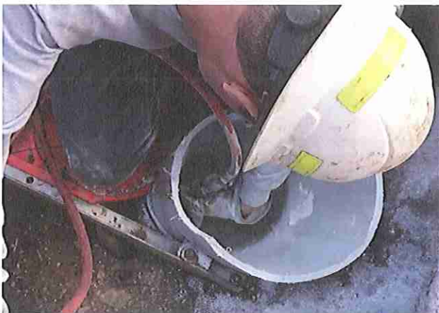
Cutting Off Upstream End of Outlet Liner
