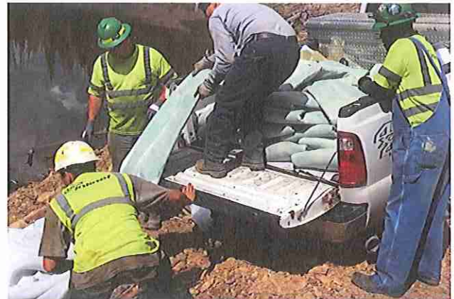
Unloading Liner Materials
