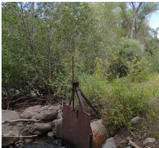
McKinley Ditch Primary Head Gate and Turnback Structures
