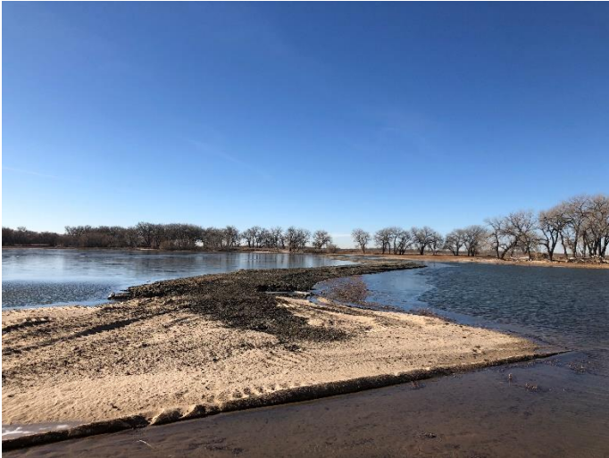
Figure 10. Completed embankment for one of the cells at Prewitt State Wildlife Reservoir Enhancement Project near Merino, Colorado. The picture shows the shallow water wetlands that will be exposed under normal drawdowns of the reservoir. This picture was taken following the annual fill of Prewitt Reservoir in late December.
