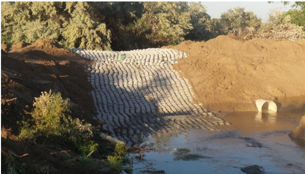
Figure 6. Installation of Agri Drain inline stoplog water control structure for the Prewitt State Wildlife Area wetland enhancement project. This structure enhanced approximately 20 acres of shallow water wetlands.
