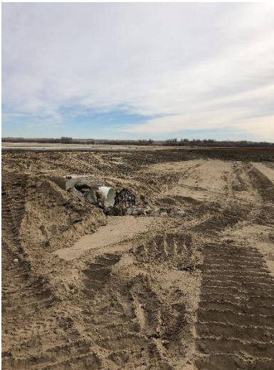
Figure 9. One of the embankments and Agri Drain inline stoplog water control structures installed as part of the Prewitt State Wildlife Reservoir Enhancement Project near Merino, Colorado. The embankment will help retain water during normal operation of the reservoir thereby providing suitable habitat to migratory birds.
