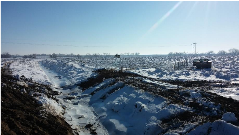
Figure 3. Phase I ditch rehabilitation after completion of the DPG Prewitt project near Merino, Colorado.
