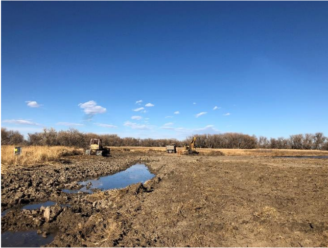
Figure 5. Construction of small embankment on cell 4 of the Prewitt Ranch and Prewitt State Wildlife Area project near Merino, Colorado. The embankment is designed to hold back water creating shallow water wetlands in portions of the reservoir that are normally dry.
