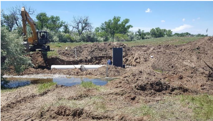
Figure 6. Installation of Agri Drain inline stoplog water control structure for the Prewitt State Wildlife Area wetland enhancement project. This structure enhanced approximately 20 acres of shallow water wetlands.
