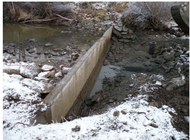
Figure 7. New Diversion Structure Dam prior to Installing Gravel Pack
