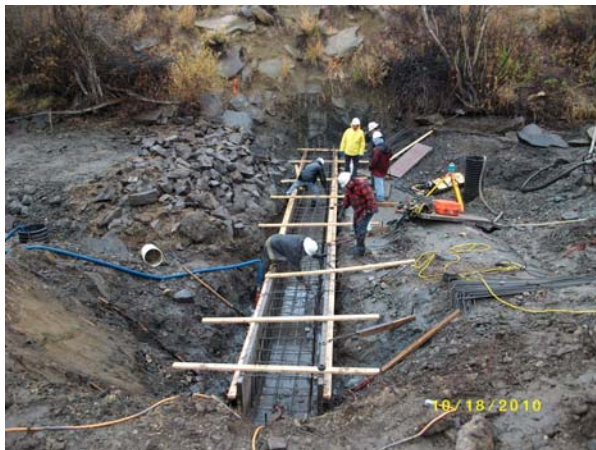
Figure 6. Constructing Footing for New Diversion Structure
