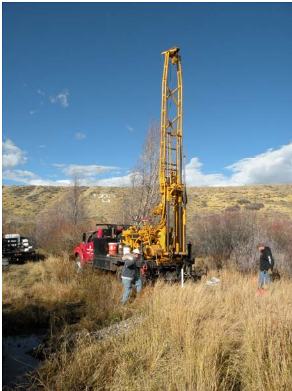
Figure 2. Drilling Test Holes
