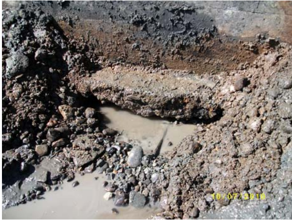
Figure 5. Piping Under the Existing Diversion Structure
