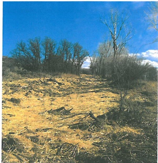
Final grading and shaping, seeding and mulching of pipeline in steep rocky section.
