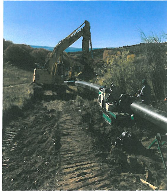
Welding HDPE pipe in the steeper and rockier terrain.
