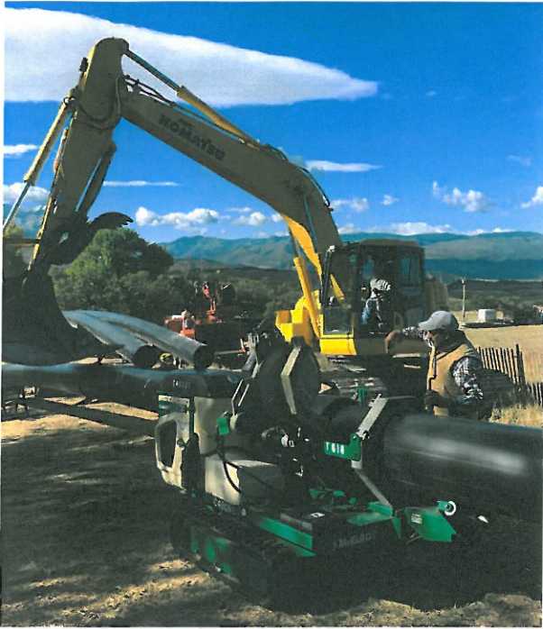
Welding sections of HDPE pipe together prior to pulling it into trench for covering.
