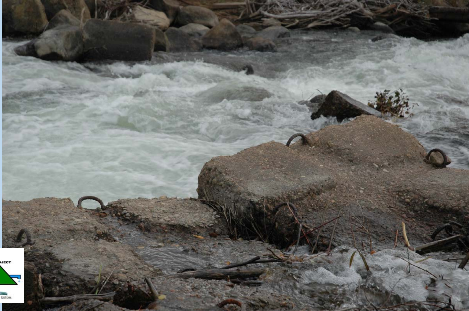
Existing Conditions, detail of articulated concrete slabs used for armoring the rockfill diversion structure.
