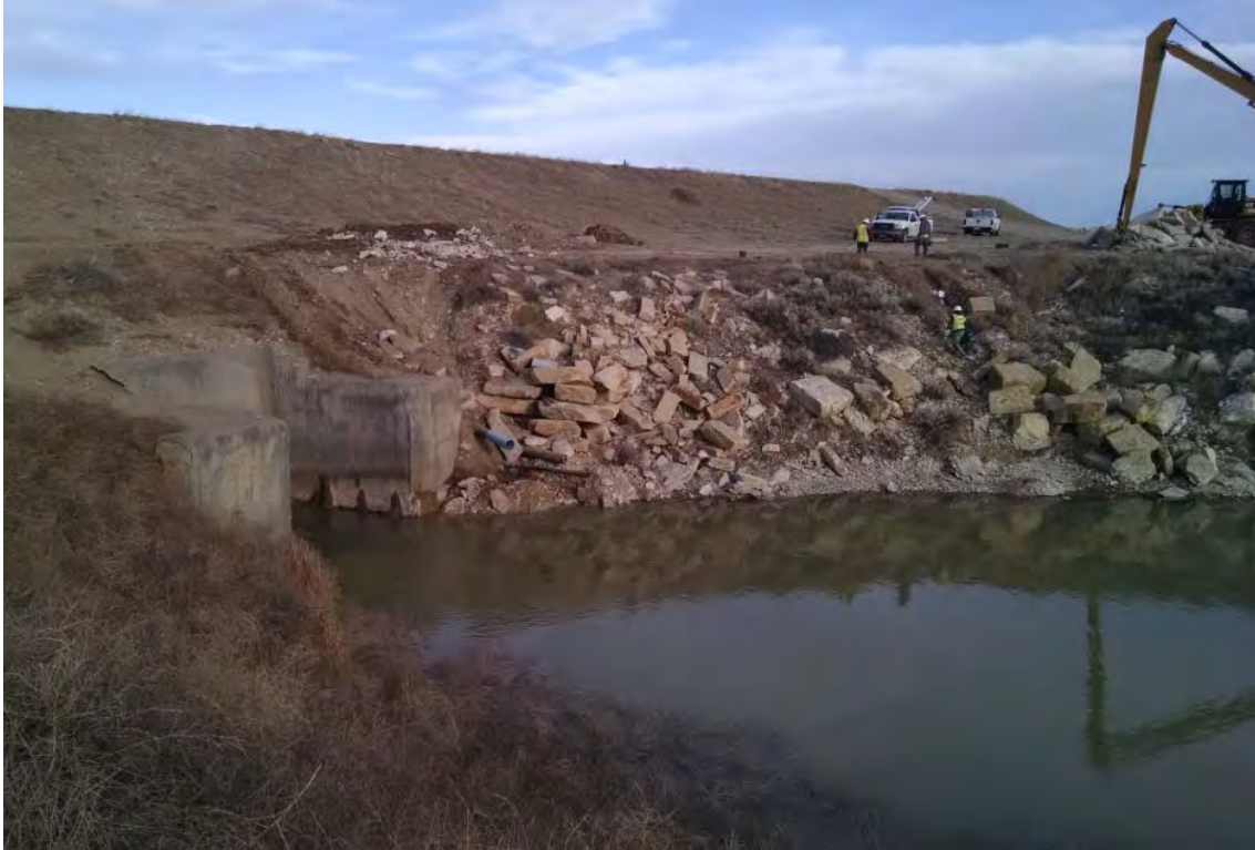
Photo 14: View of the repair area after completion of work. Note the additional riprap placed below the toe drains. Further riprap to be placed above the drain pipes at a later date. March 25, 2016.
