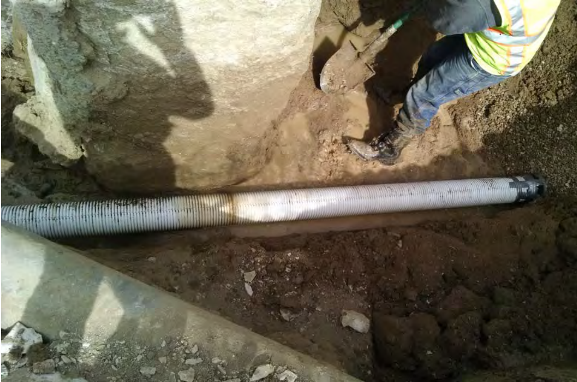
Photo 9: View of the new 6-inch-diameter slotted drain pipe bedded in the ASTM C-33 concrete sand. March 25, 2016.
