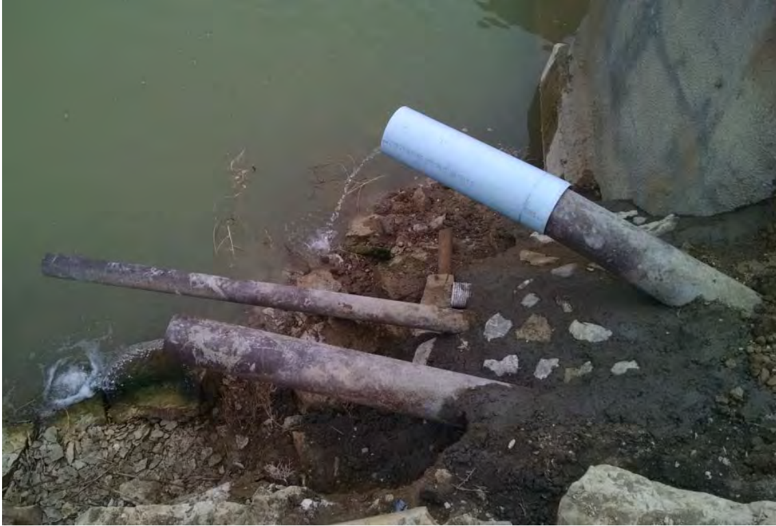
Photo 13: View of left abutment seepage drain pipes after concrete cap placement on new drain. The blue pipe on the far right pipe in the picture is a temporary sleeve to prevent water flow on uncured concrete. March 25, 2016.
