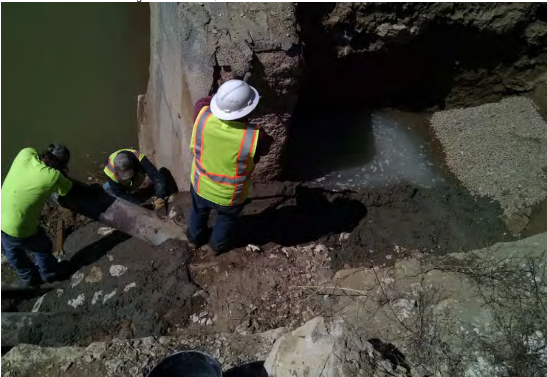
Photo 12: View of completed concrete placement over ASTM C-33 concrete sand. FLCC is performing finishing work of concrete. Note the seepage water ponded behind the concrete. March 25, 2016.
