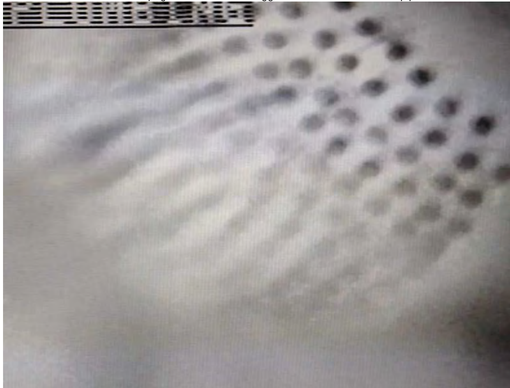
Screenshot 4: 1996 Left Seepage Drain: Unclogged perforations on upstream end cap of drain pipe. March 23, 2016.
