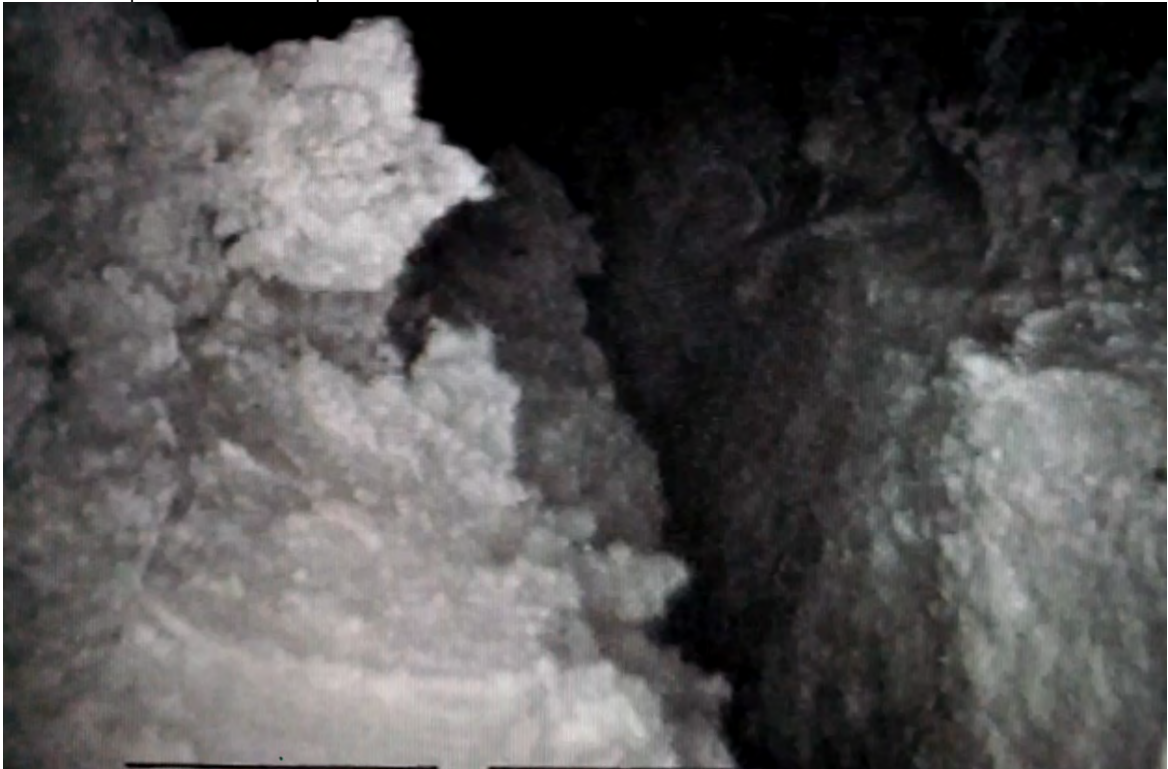
Screenshot 2: Uncontrolled Seepage Exit: View of interior of seepage channel at approximately three feet upstream of the exit point. March 23, 2016.
