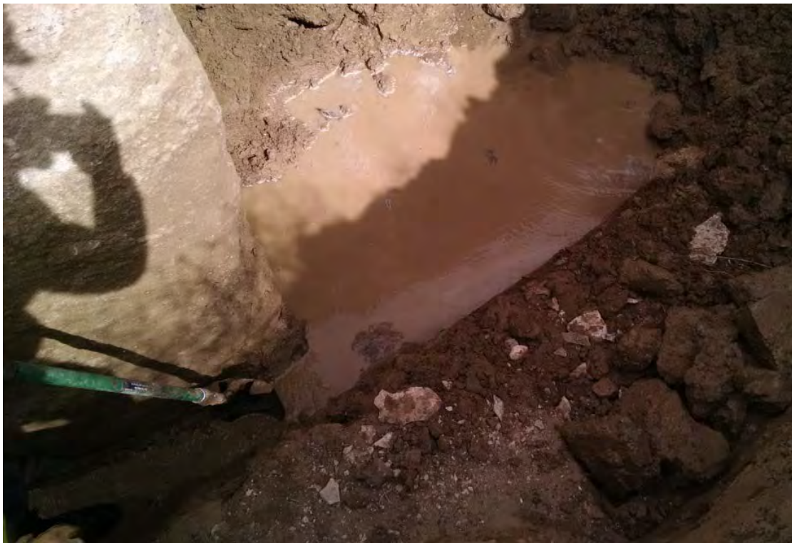
Photo 6: The excavation has reached the uncontrolled seepage path in this view. March 25, 2016.
