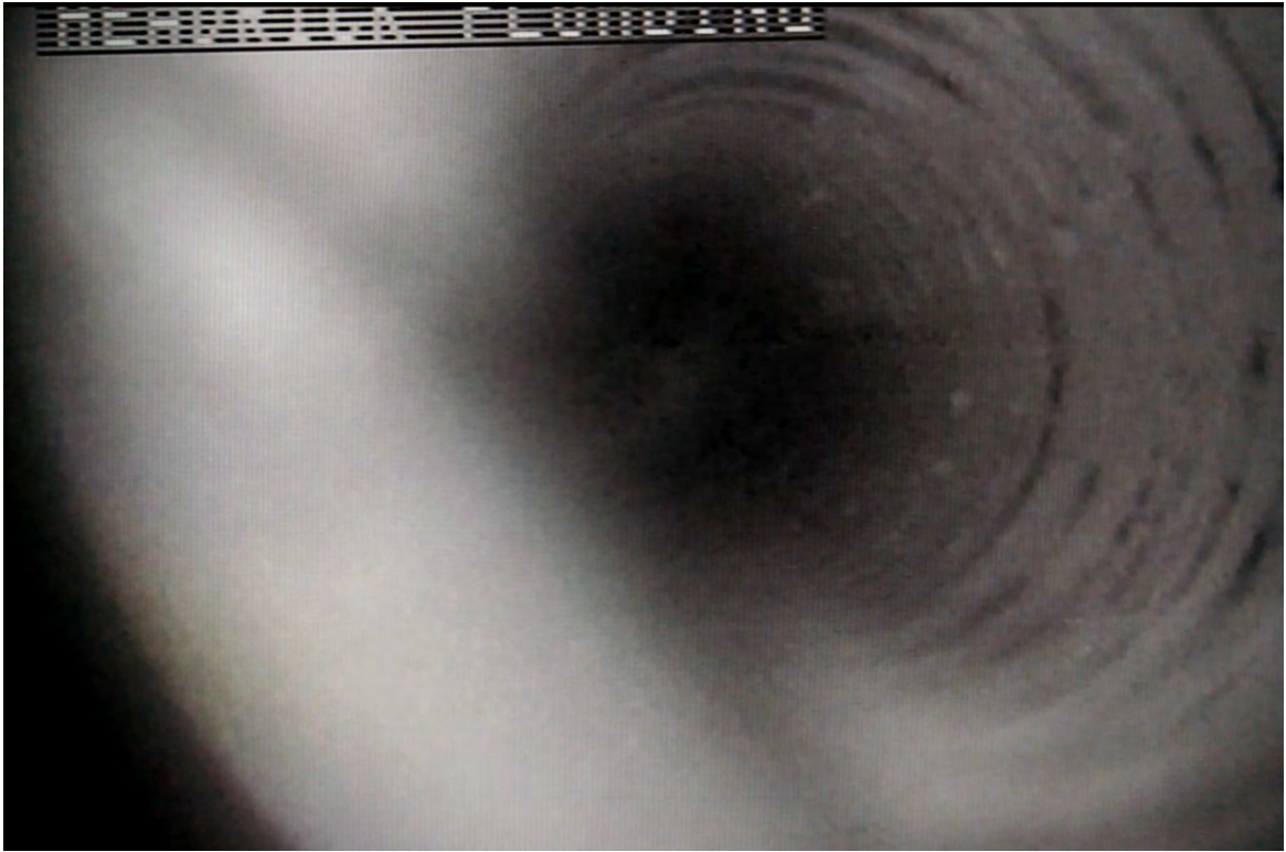
Screenshot 5: 1996 Left Seepage Drain: Unclogged slots in drain pipe. March 25, 2016.
