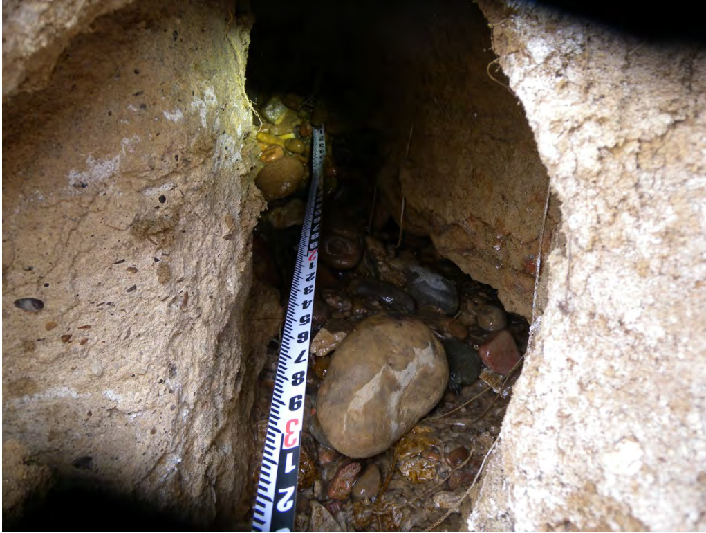
Photo 3: View looking up the uncontrolled seepage path left of the outlet works. March 22, 2016.
