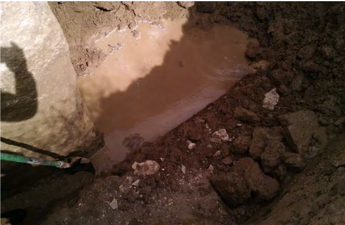
Photo 10: View of the new drain excavation with ASTM C33 concrete sand cover over the new slotted pipe and gravel upstream. Note the seepage water ponded behind a temporary sand dam. March 25, 2016.
