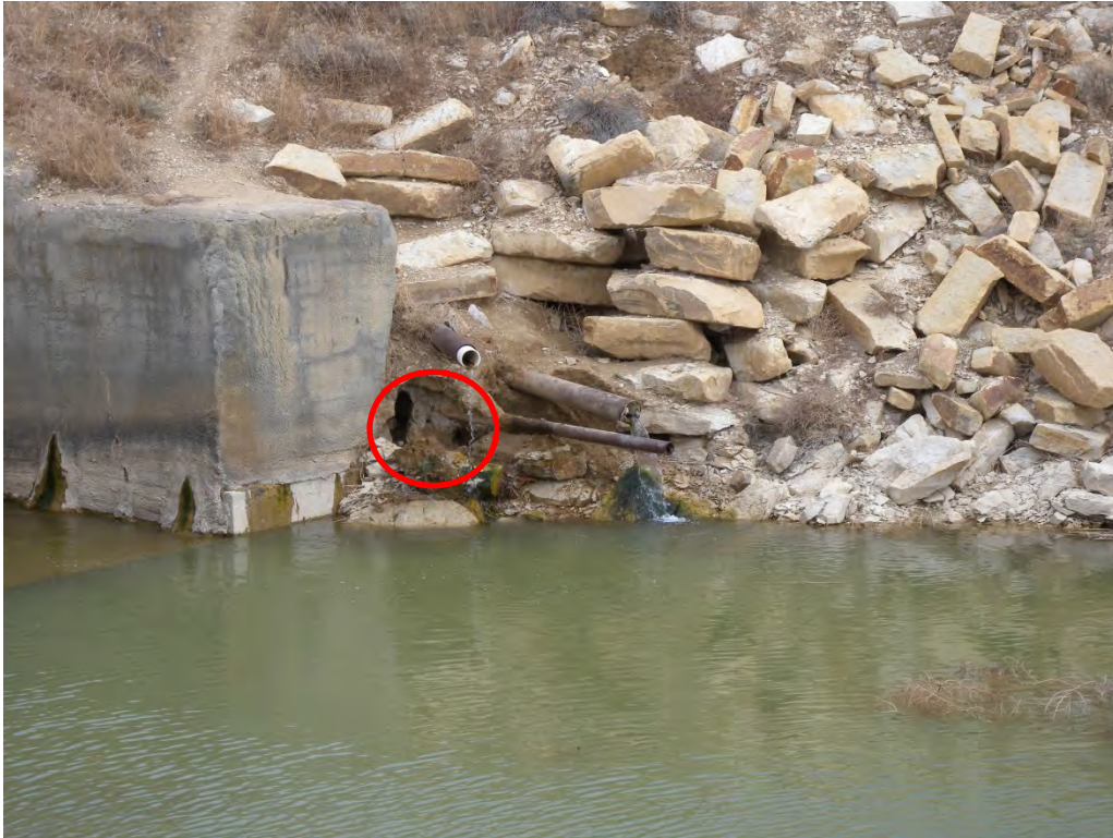
Photo 1: View of left abutment seepage drains and uncontrolled seepage path exit point left of the outlet works. March 22, 2016.
