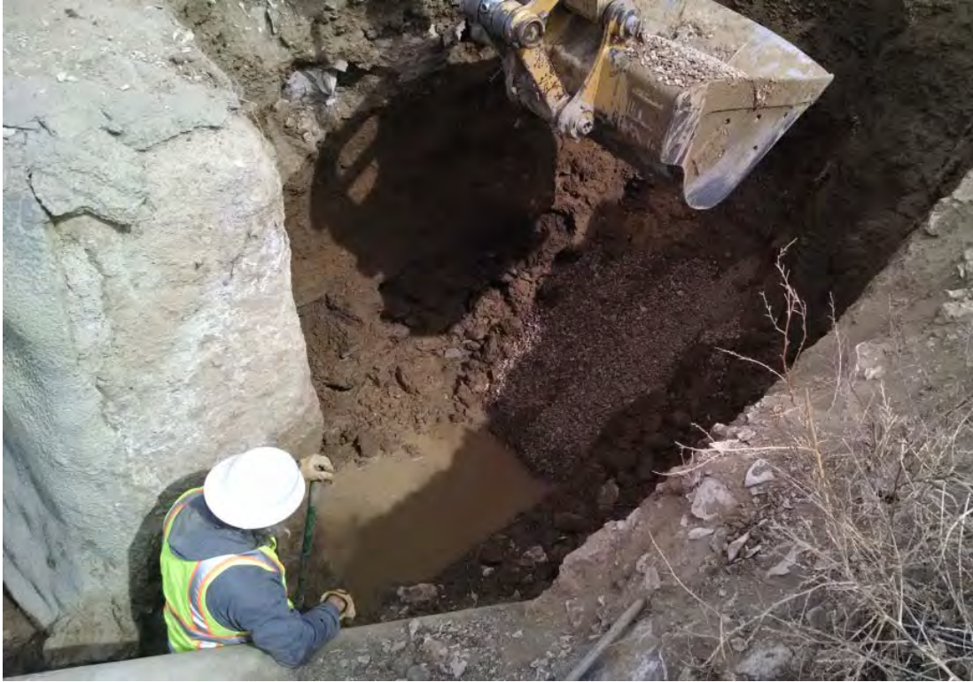
Photo 7: View of excavation during initial placement of gravel along upstream excavation slope. March 25, 2016.
