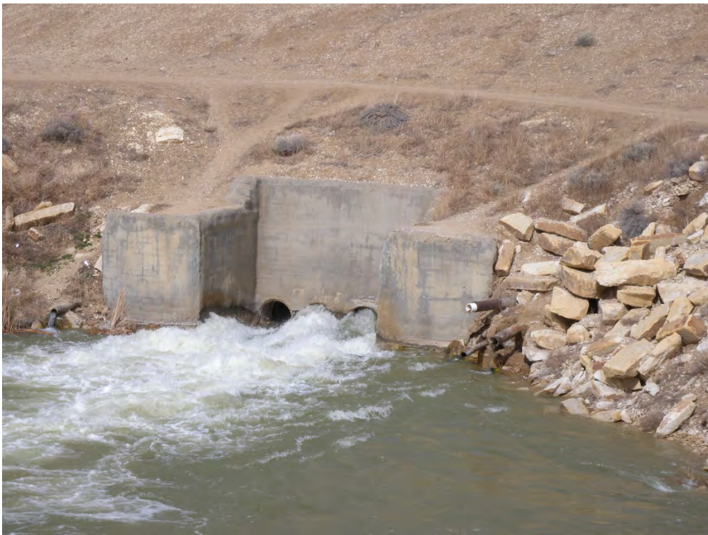
Photo 4: View of the outlet works and seepage drain pipes looking upstream. The center two outlet pipes were discharging approximately 300 cfs when the photo was taken. March 22, 2016.
