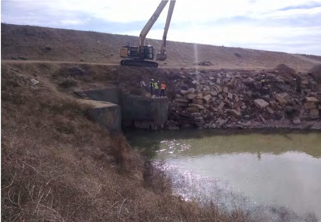
Photo 5: Commencement of initial excavation and riprap removal from slope above seepage drains left of the outlet works. March 25, 2016.
