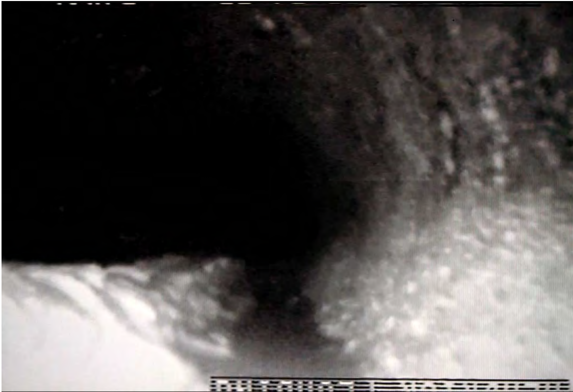
Screenshot 3: 2008 Left Seepage Drain: View of clogged slots on bottom half of pipe. March 23, 2016.
