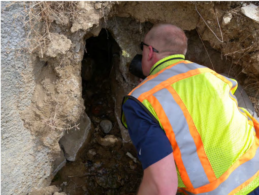
Photo 2: View of Trevor Mugele observing the uncontrolled seepage path exit point left of the outlet works. March 22, 2016.
