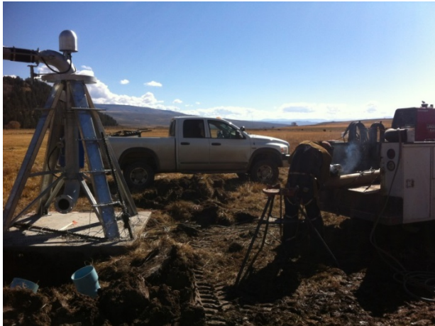
Welding Z pipe, which connects 8in PVC to the Pivot
