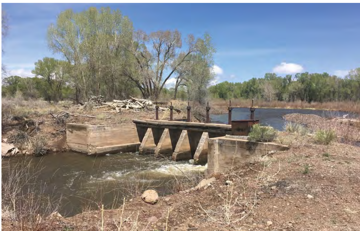
Figure 8: Consolidated Slough Headgate
