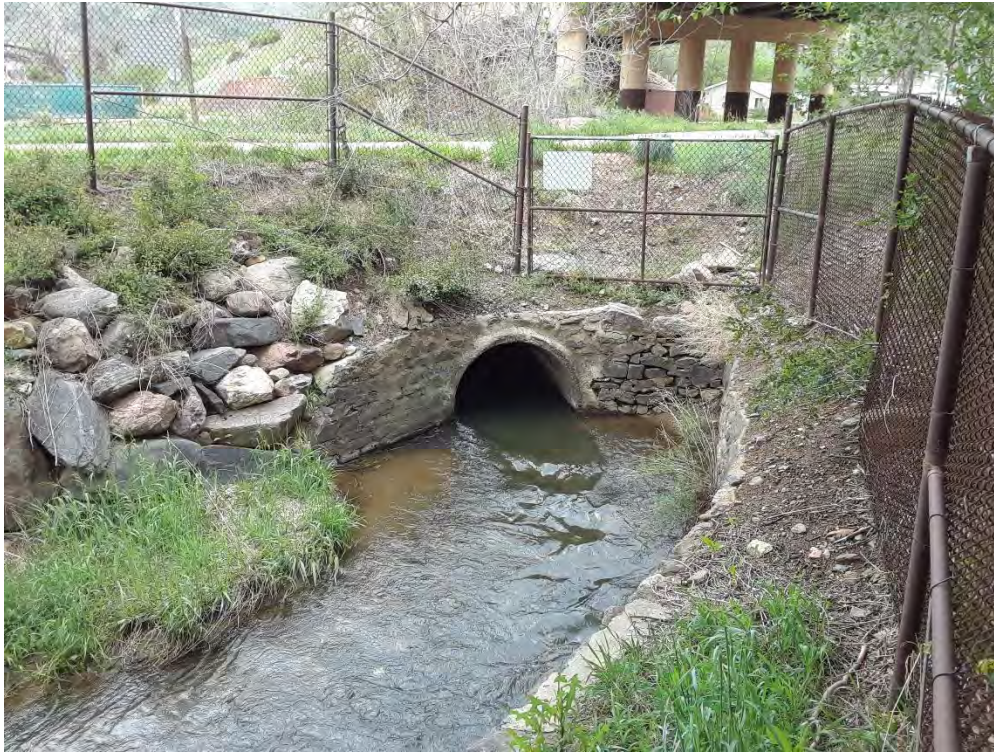
Figure 1.12. Ford Street Siphon Outlet
