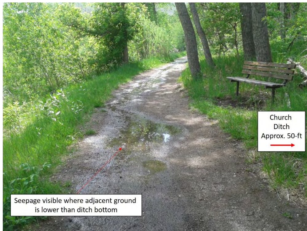
Figure 1.9. Seepage 50-ft South of Church Ditch in Area 15 (Facing West near W. 46 th Ave)
