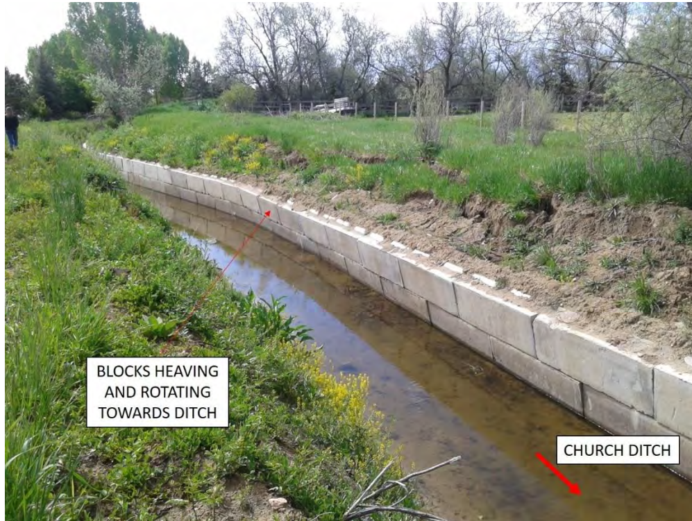
Figure 1.6. Headgate 53 Retaining Wall (Facing Upstream Along Church Ditch)
