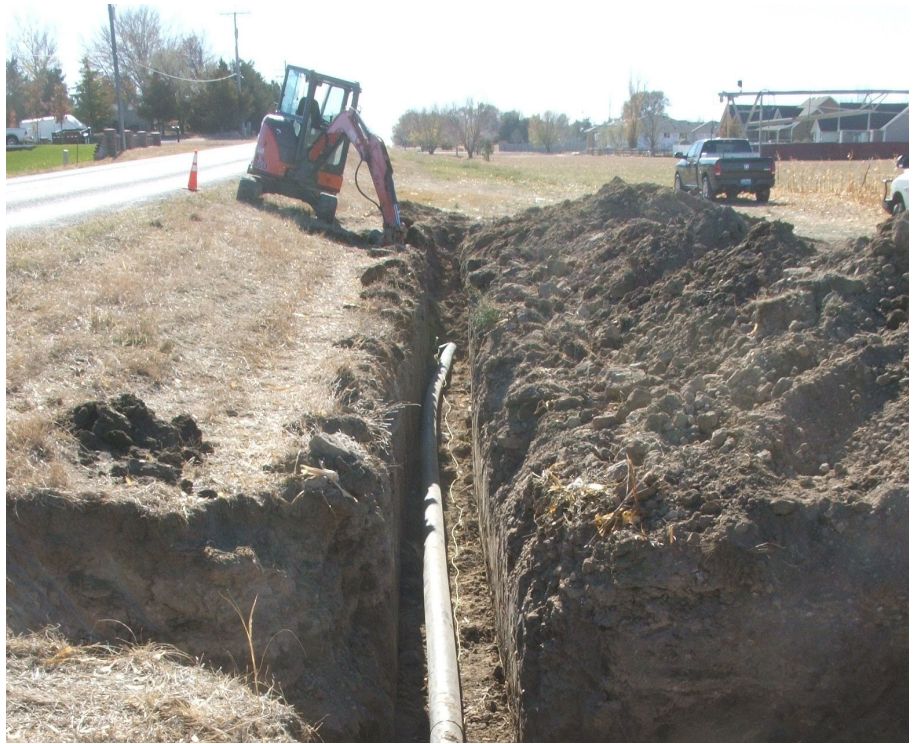
Open trench installation of 6" pipeline running north along the west side of County Road 37.
