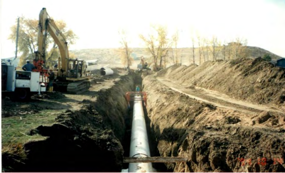
Photograph 2. Example of construction of the original SWSP in 1995, near Woodland Road.
