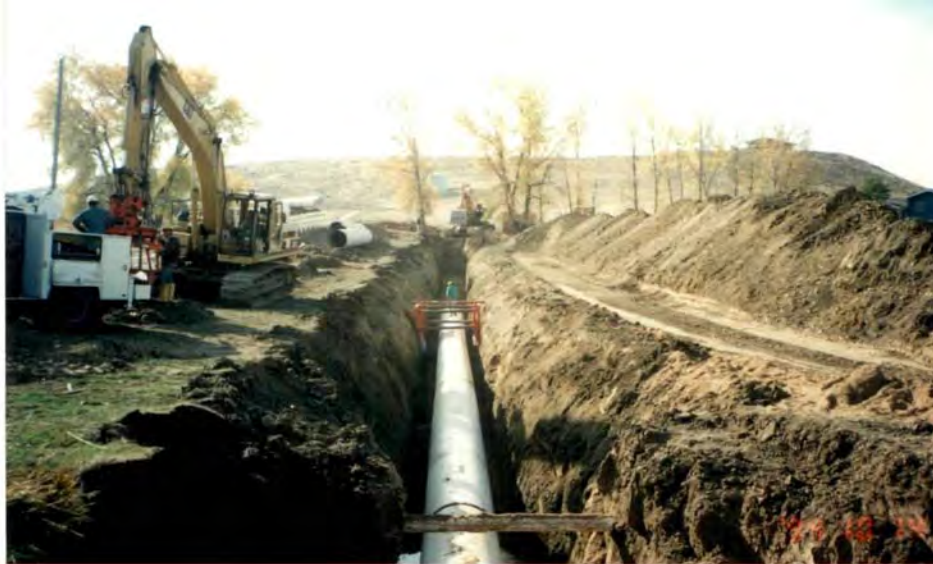
Photograph 2. Example of construction of the original SWSP, near Woodland Road.
