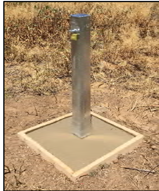
Figure 8. Monitoring well completion picture
