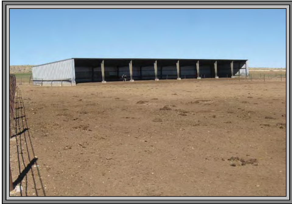
Compost Cattle Barn / Loafing Shed
