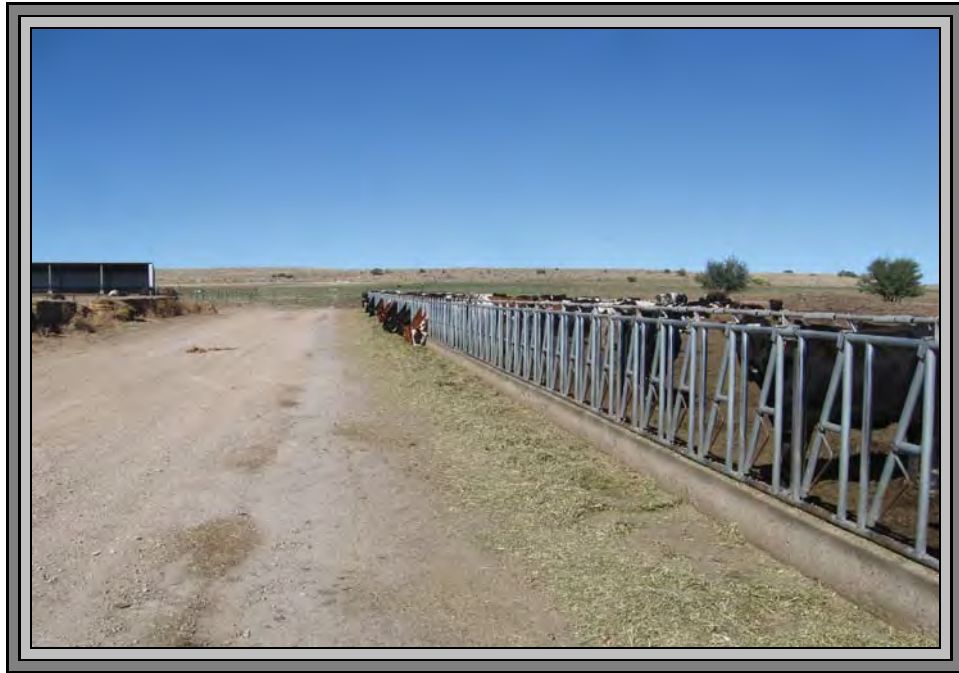
Open Concrete Feed Lane and Attached Confinement Pens
