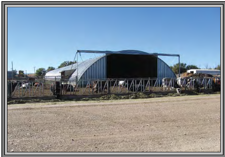
Quonset Cattle Barn / Loafing Shed
