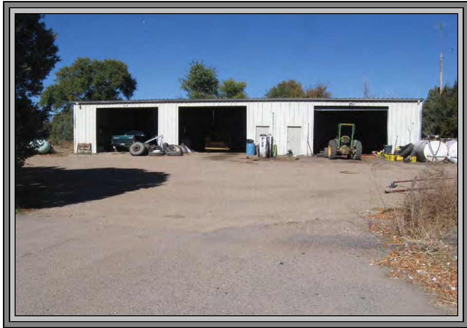
Machine Shed / Shop Building
