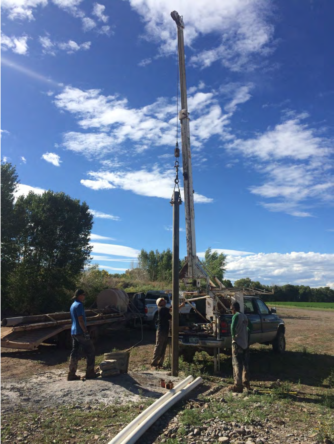
Figure 2: Installing 6" steel casing at Conejos West shallow piezometer. September, 2014.
