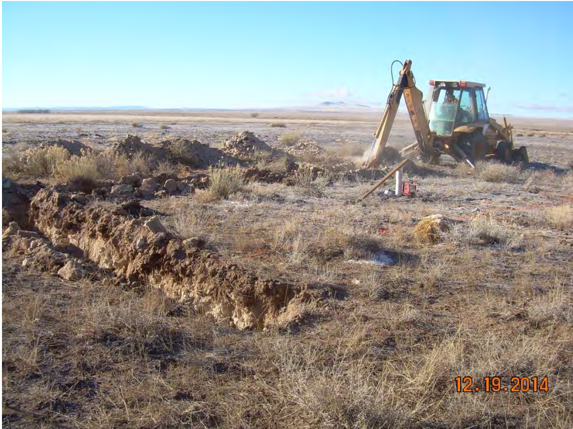
Figure 10: Digging test trenches for recharge test at Bountiful West site. December, 2014.
