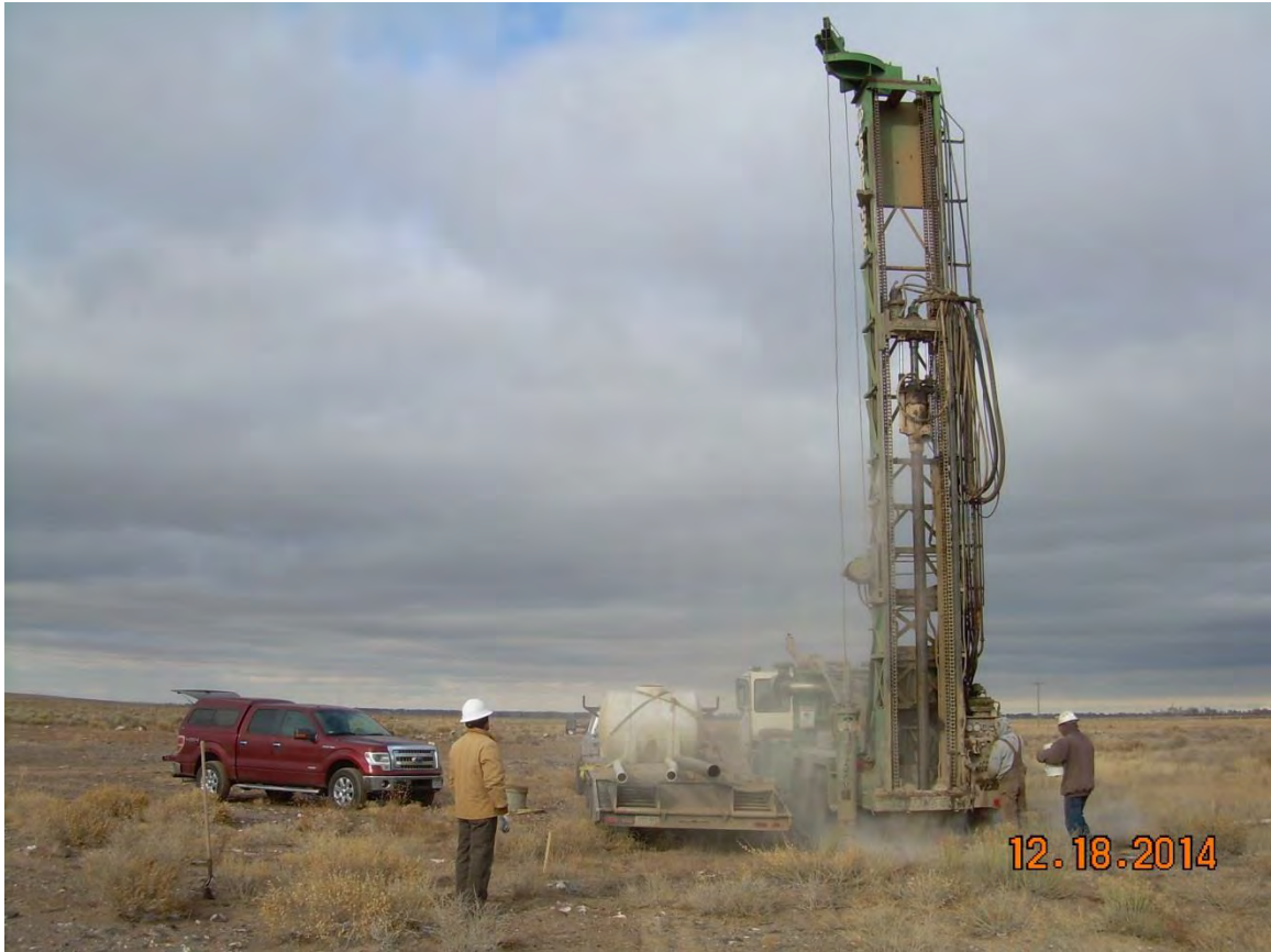
Figure 3: Drilling shallow piezometer at Bountiful West test site. December, 2014.
