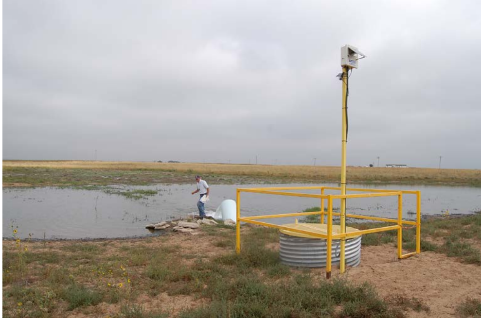
Figure 5: Recharge pond at Orcharge Project. Deliveries can be sustained at rates of approximately 3 cfs per surface acre because of the sandy geologic conditions.
