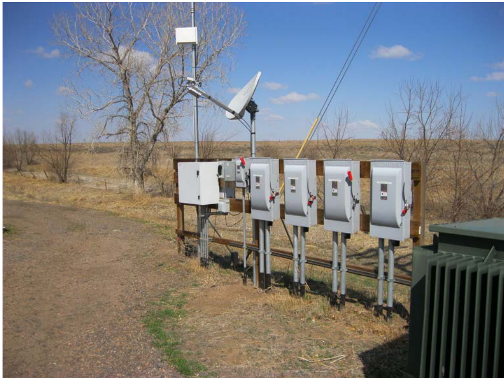
Figure 6: All wells at Central's adjacent Orchard Project have been equipped with SCADA to allow remote control of facilities and optimization of well pumping/recharge operations.
