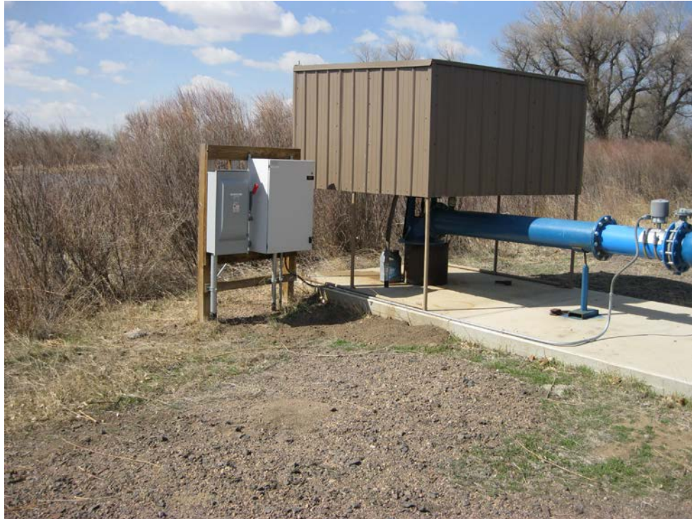
Figure 3: Headgate well at Central's adjacent Orchard Project. Six wells divert from north bank of South Platte River for delivery to recharge ponds.
