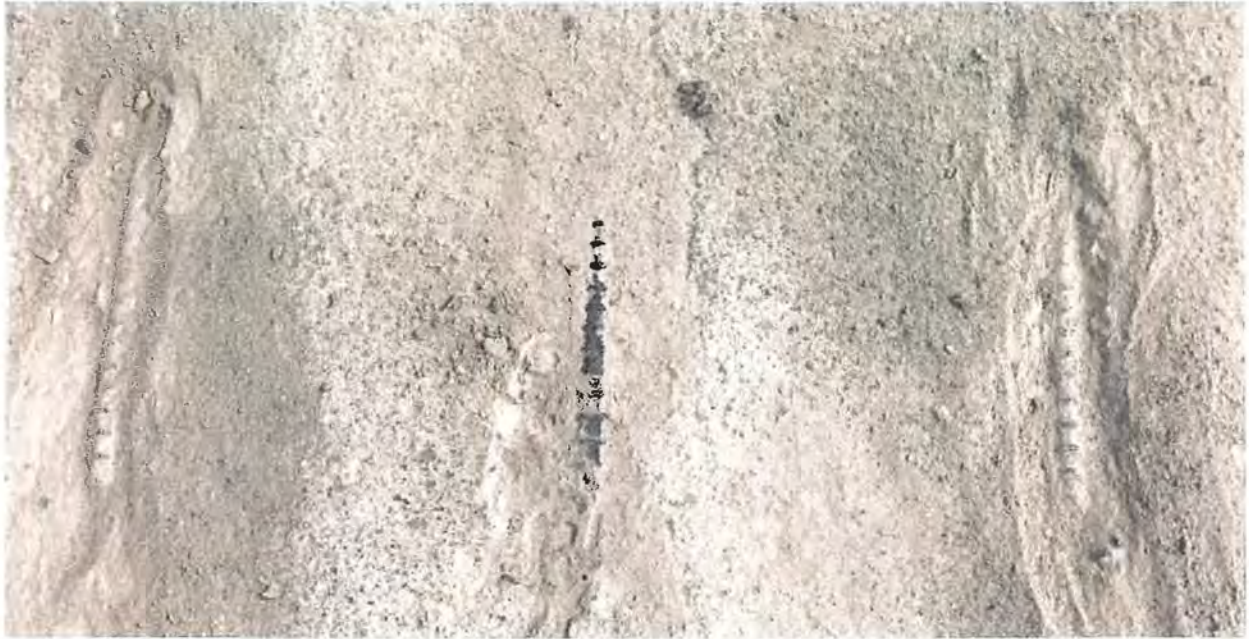
Figure 69: Exposed rebar on the invert of the Persigo Wash flume is typical. Grand Valley Project, Colorado 3/13/2017
