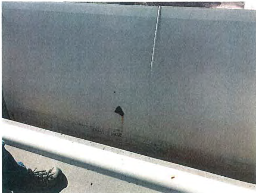
Figure 43: Coating on the Lewis Wash radial gate is started to peel. Grand Valley Project, 3/1/2017
