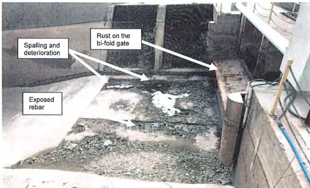
Figure 10: Looking at the upstream end of the Langemann gate at the tunnel 3 outlet. Photo was taken from the right bank looking towards the left bank. Note the cracking and section loss in the concrete invert as well as the spalling below the intake screen. Grand Valley Project, Colorado 2/21/2017.
