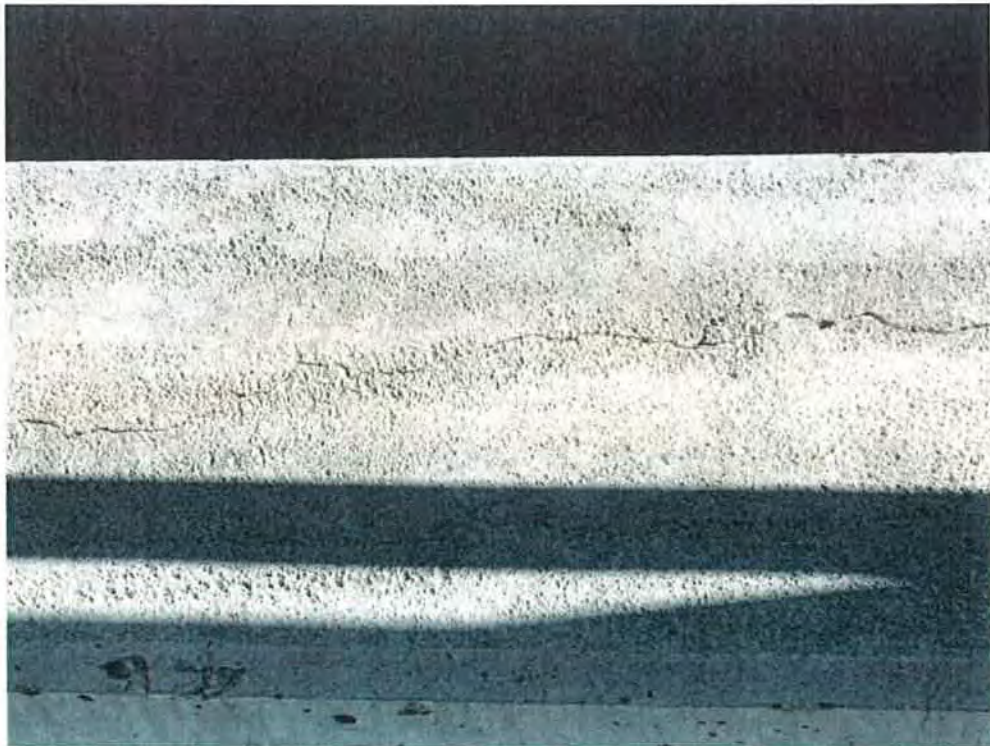
Figure 52: Longitudinal cracking on check A7. Grand Valley Project, Colorado 3/2/2017
