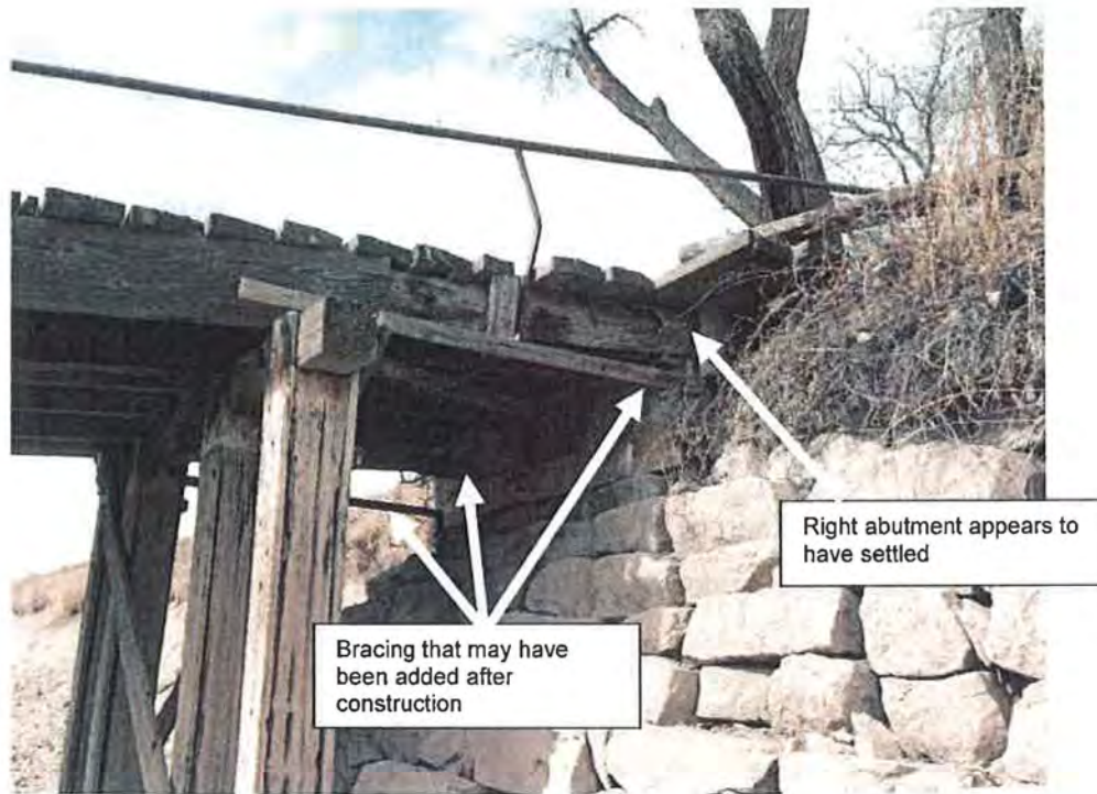
Figure 22: Right abutment and bent of the timber bridge. Grand Valley Project, Colorado 2/21/2017
