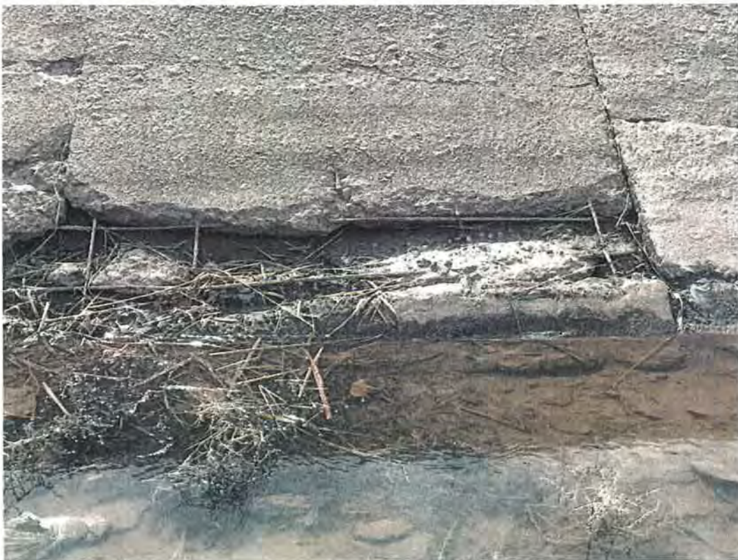
Figure 39: Exposed rebar in concrete lining. Grand Valley Project, Colorado 2/21/2017
