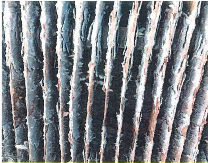
Figure 15: The intake screen for the Stub Pump Plant has significant corrosion and section loss. Grand Valley Project, Colorado 3/1/2017
