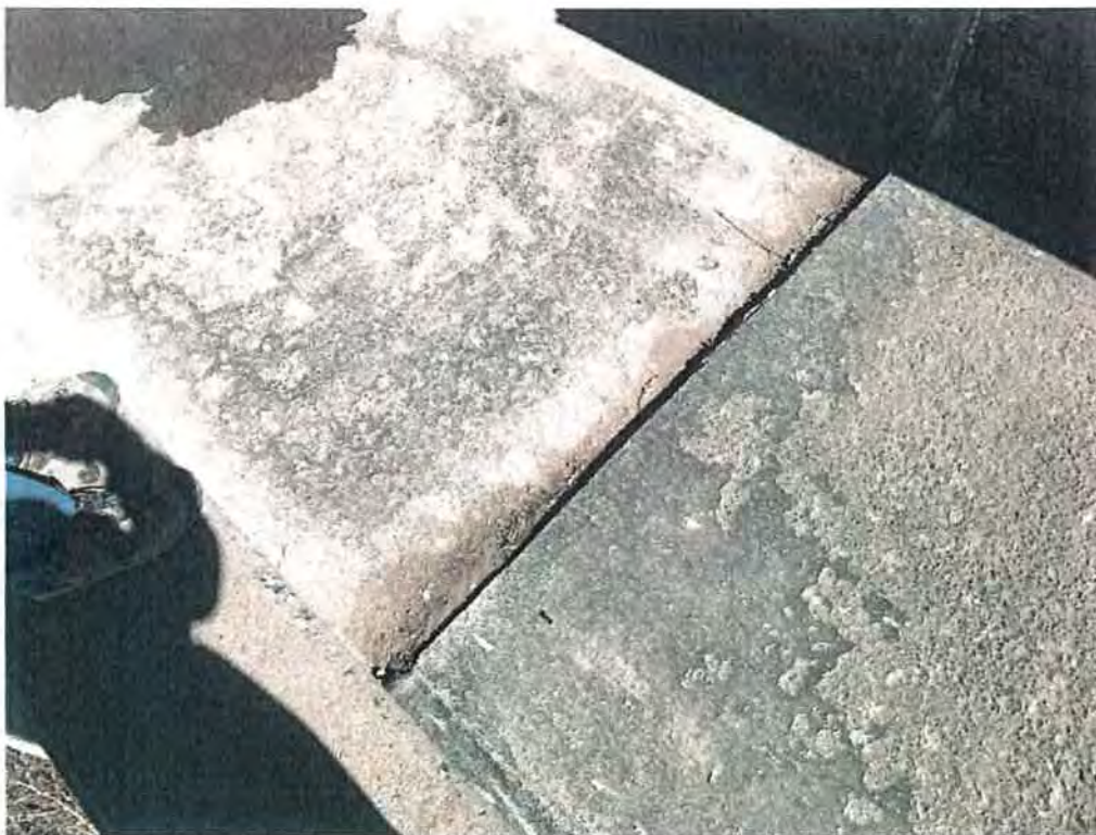
Figure 64: Offset in the flume invert at the expansion joint. Grand Valley Project, Colorado 3/2/2017
