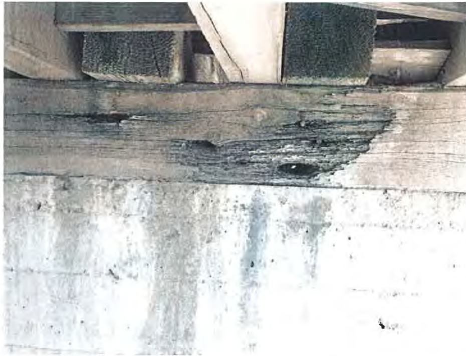
Figure 97: Decay was observed at several locations on the Little Salt Wash O&M bridge. Grand Valley Project, Colorado 3/13/2017
