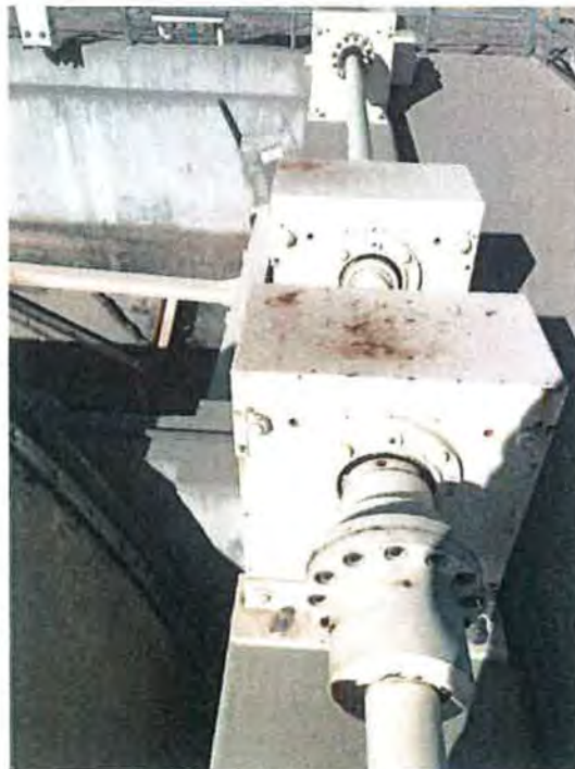
Figure 48: Rusting on some of the mechanical portions of check A 1 1/4. Grand Valley Project, Colorado 3/1/2017
