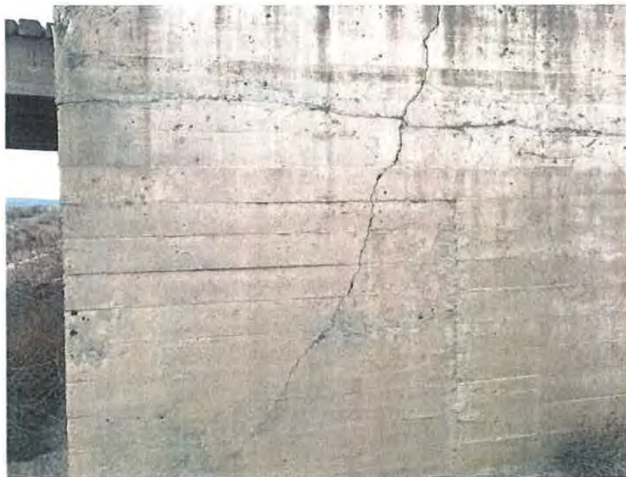
Figure 84: Significant cracking along the abutment of the Adobe Wash O&M road. Grand Valley Project, Colorado 3/13/2017
