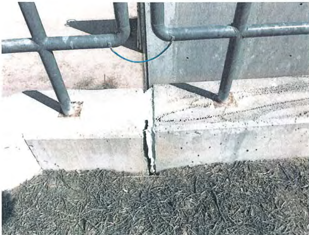
Figure 100: Possible movement of the wing walls of the A32 check structure. Grand Valley Project, Colorado 3/13/2017
