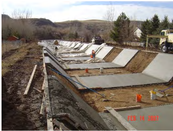
Figure 4.3.2. Installation of Reinforced Concrete Canal Liner
