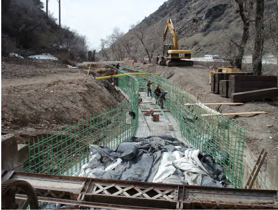
Figure 4.5.1. Construction of Concrete Forms for Cast-In-Place Concrete Box Culvert
