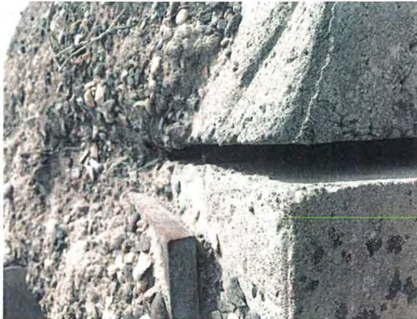
Figure 77: Possible differential settlement on the outlet wall for the Persigo Wash wasteway. Grand Valley Project, Colorado 3/13/2017
