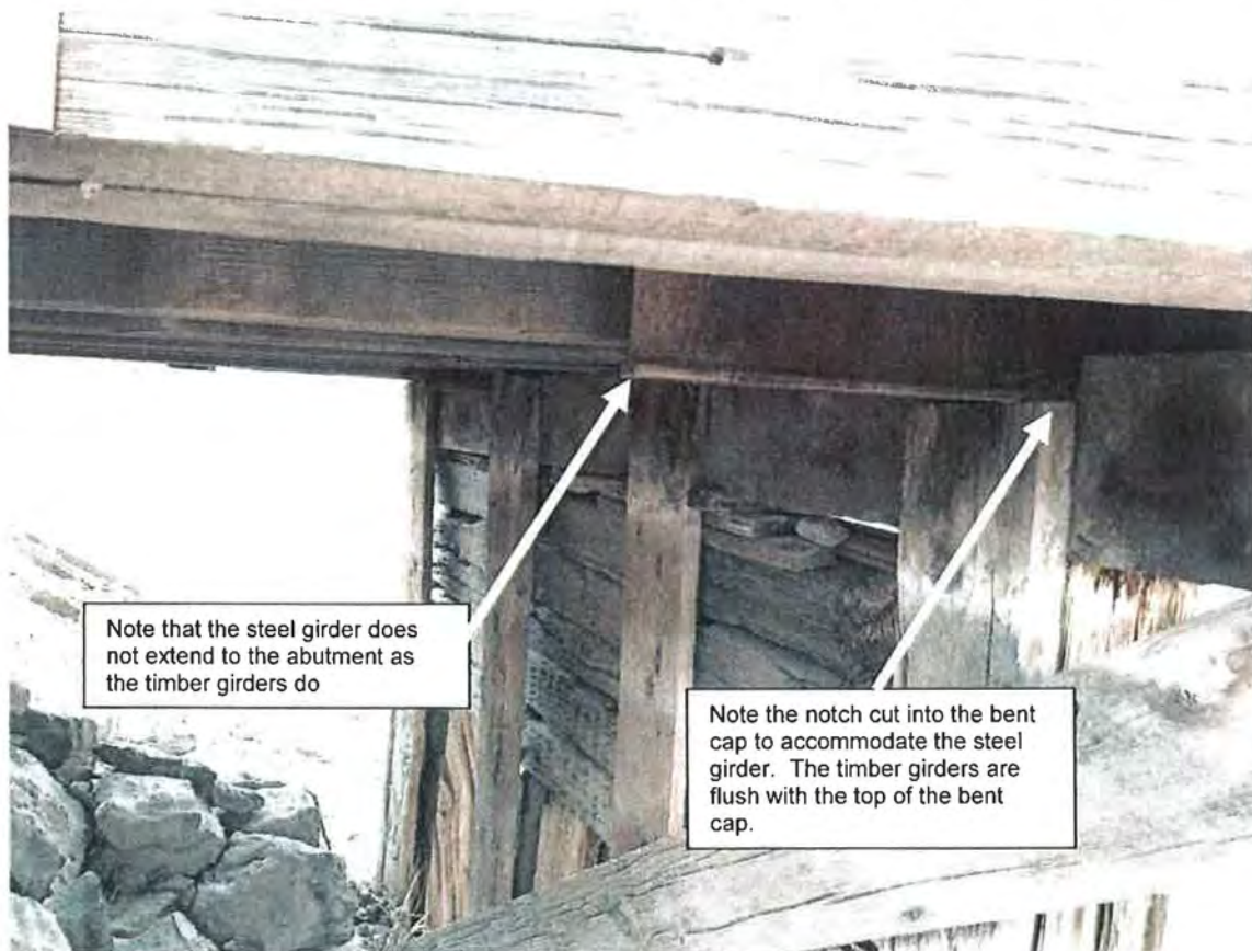
Figure 27: Close up of the left bent and bent cap. Grand Valley Project, Colorado 2/21/2017
