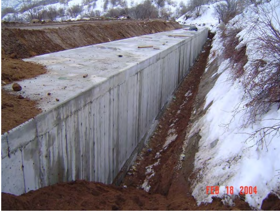
Figure 4.5.3. Completed Cast-In-Place Concrete Box Culvert
