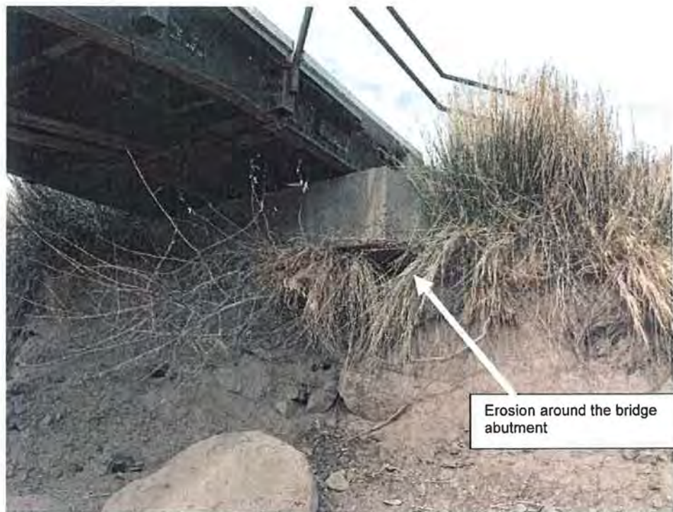
Figure 17: Erosion around the bridge abutment at station 1343+77. Grand Valley Project, Colorado 2/21/2017
