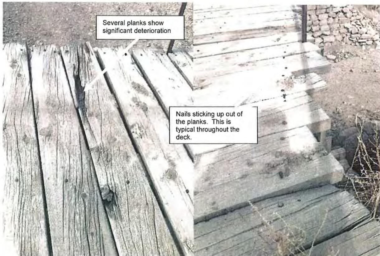
Figures 29 and 30: Close up of timber deck deficiencies. Grand Valley Project, Colorado 2/21/2017
