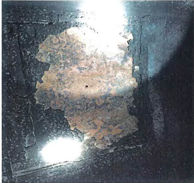
Figure 7: The coating on an access panel used during the tunnel realignment is showing significant peeling and flaking. The underlying metal has substantial corrosion as a result. The hole in the center of the access door should be noted. Grand Valley Project, Colorado 3/1/2017.
