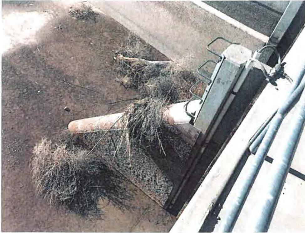
Figure 49: Rusting on some of check A 7. Grand Valley Project, Colorado 3/2/2017
