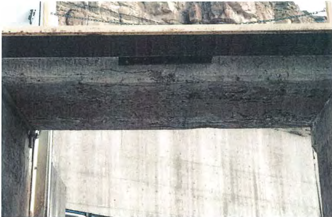
Figure 11: The underside of one of three bays for the Price Stub check at the Tunnel 3 outlet. Note the cracking and efflorescence. This is typical of all three bays. Grand Valley Project, Colorado 2/21/2017.
