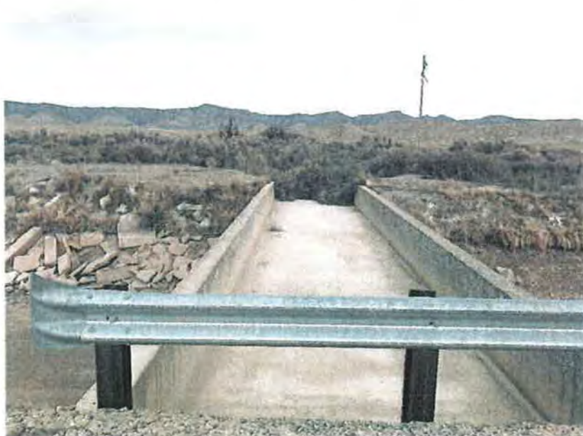
Figure 68: Persigo Wash overshoot flume. Grand Valley Project, Colorado 3/13/2017
