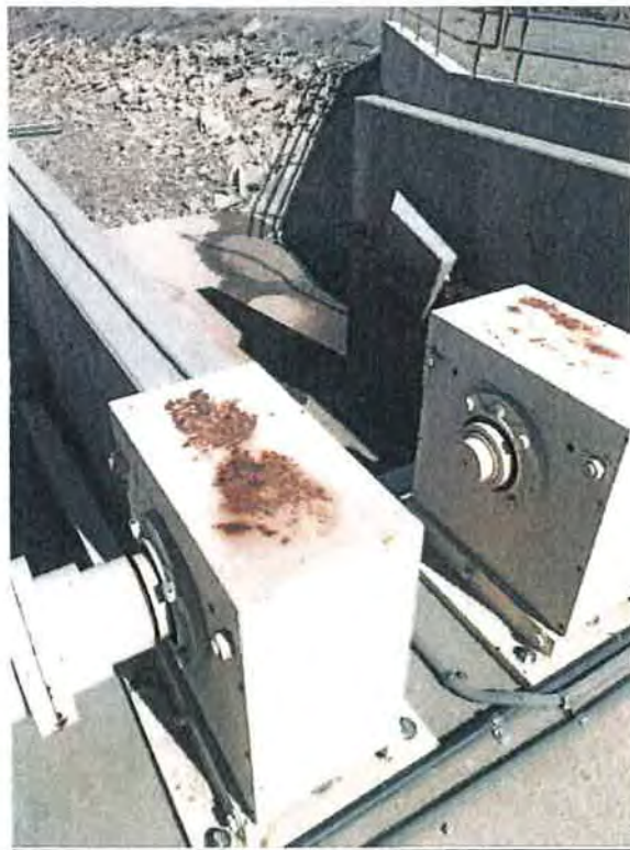
Figure 82: Rust on the mechanical portions of the A 21 ½ check structure. Grand Valley Project, Colorado 3/2/2017
