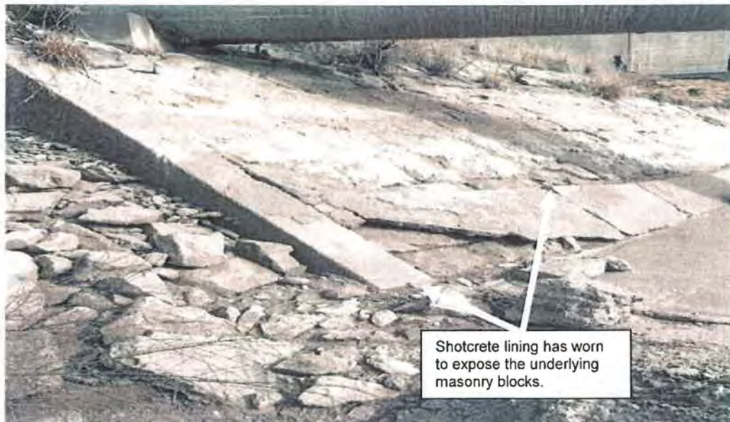
Figure 13: The right bank downstream of the Langemann gate at the tunnel 3 outlet. Note the deterioration of the shotcrete lining that covered the masonry along the bank. Grand Valley Project, Colorado 2/21/2017
