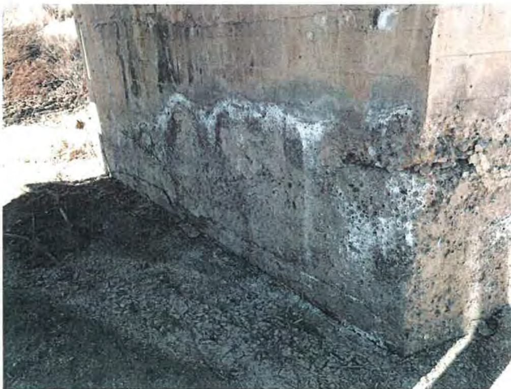
Figure 56: Cracking, spalling, and apparent efflorescence along the abutment of the 1220 flume O&M bridge. Grand Valley Project, Colorado 3/2/2017
