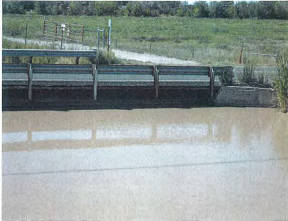
Figure 40: Low freeboard on the 34 Rd Bridge. Grand Valley Project, Colorado 9/23/2014
