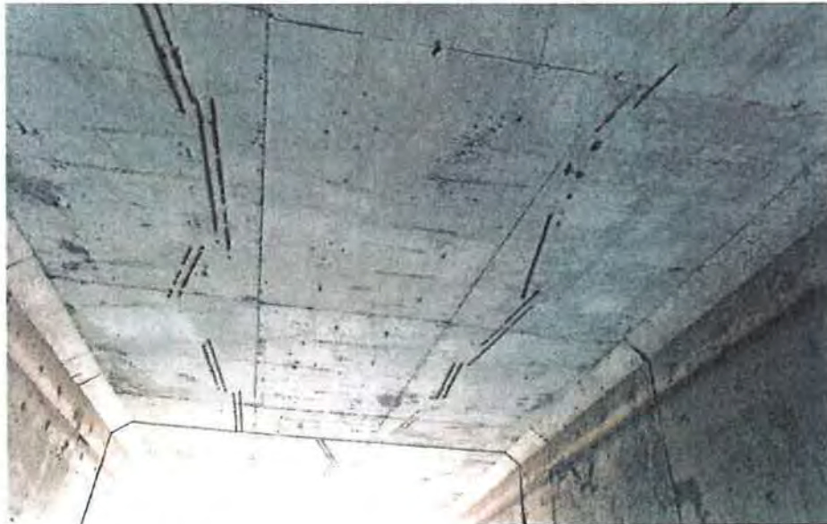
Figure 8: Unusual marks on the roof of Tunnel 3 near the outlet. This portion of the tunnel is located under I-70. It is unclear at this time what the cause of these markings are. Grand Valley Project, Colorado 3/1/2017.
