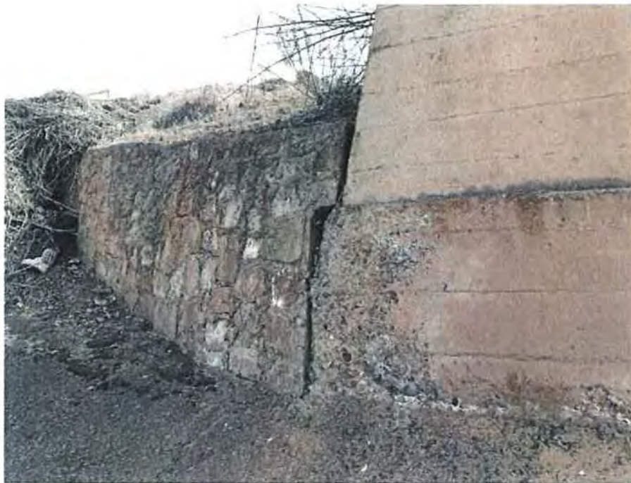
Figure 95: The gap between the masonry retaining wall and the siphon may indicate differential settlement. Grand Valley Project, Colorado 3/13/2017
