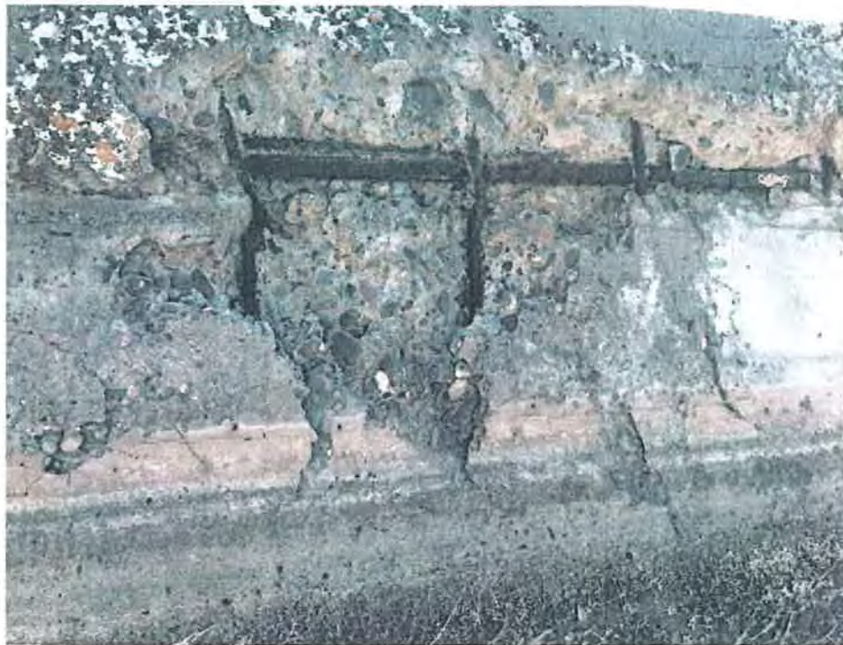
Figure 63: Damage concrete and exposed rebar on the 1270 flume. Grand Valley Project, Colorado 3/2/2017
