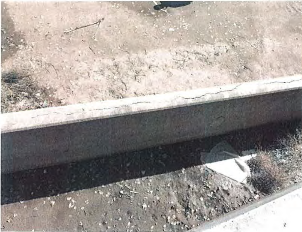
Figure 59: Longitudinal cracking at the A15 check structure. Grand Valley Project, Colorado 3/2/2017
