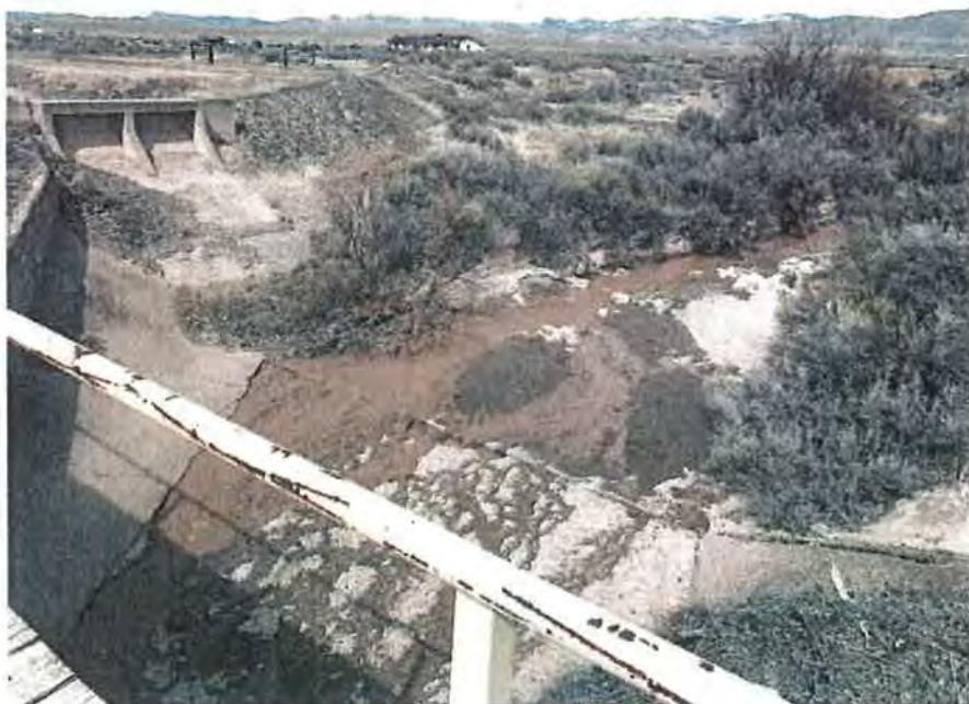
Figure 90: Vegetation encroaching on the Little Salt Wash channel. Grand Valley Project, Colorado 3/13/2017
