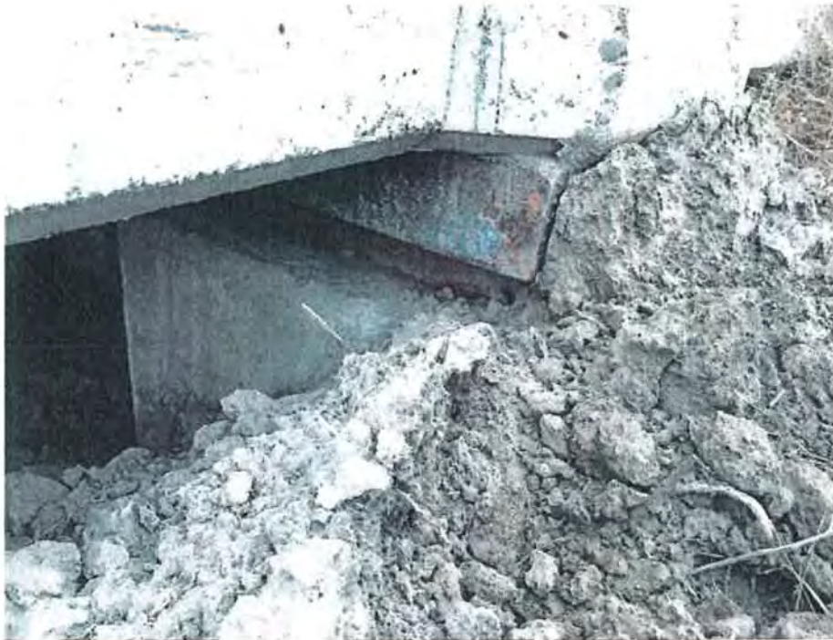
Figure 83: Dirt around one of the bearings for the Adobe Wash flume. Grand Valley Project, Colorado 3/13/2017
