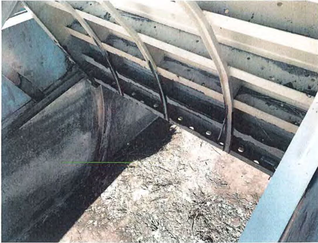
Figure 51: Rusting on some of check A 7. Grand Valley Project, Colorado 3/2/2017
