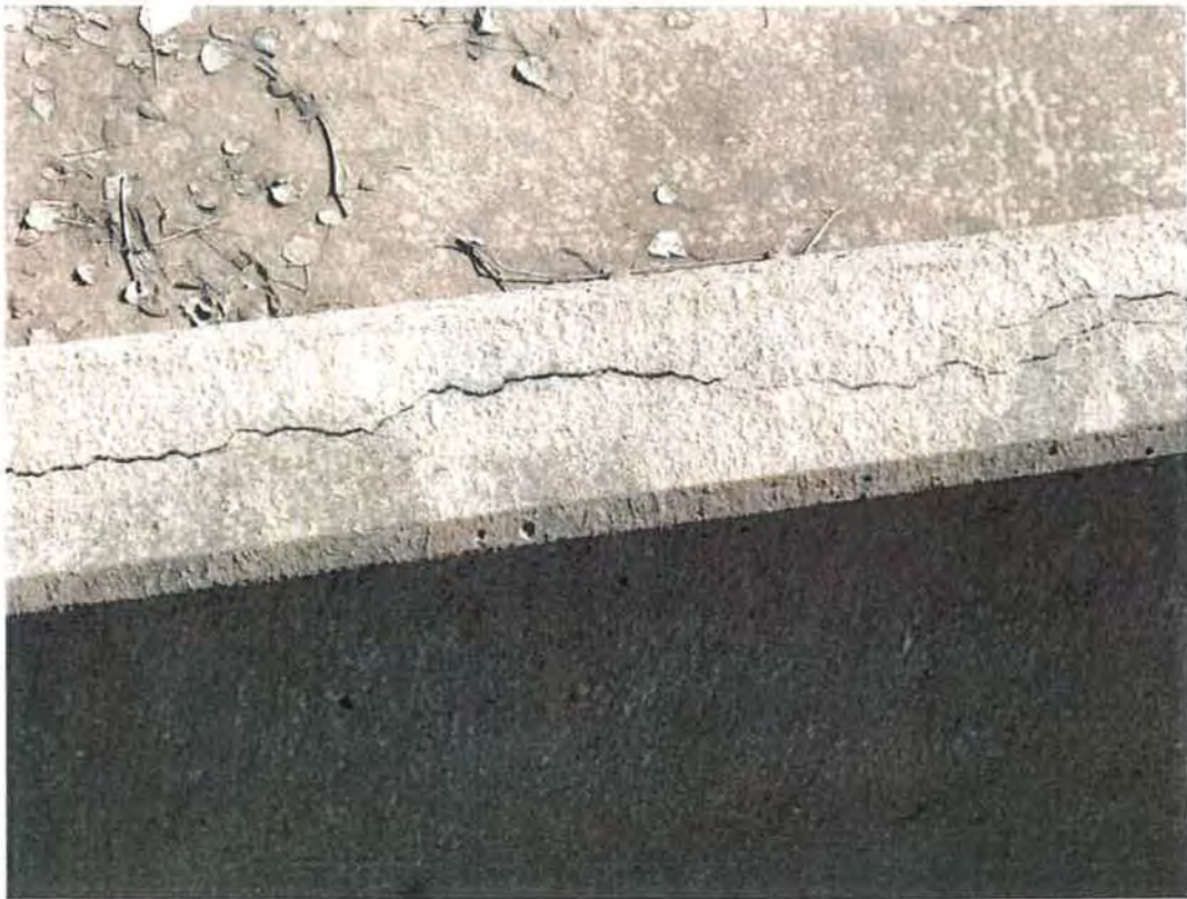
Figure 58: Close up of the longitudinal cracking at the A15 check structure. Grand Valley Project, Colorado 3/2/2017
