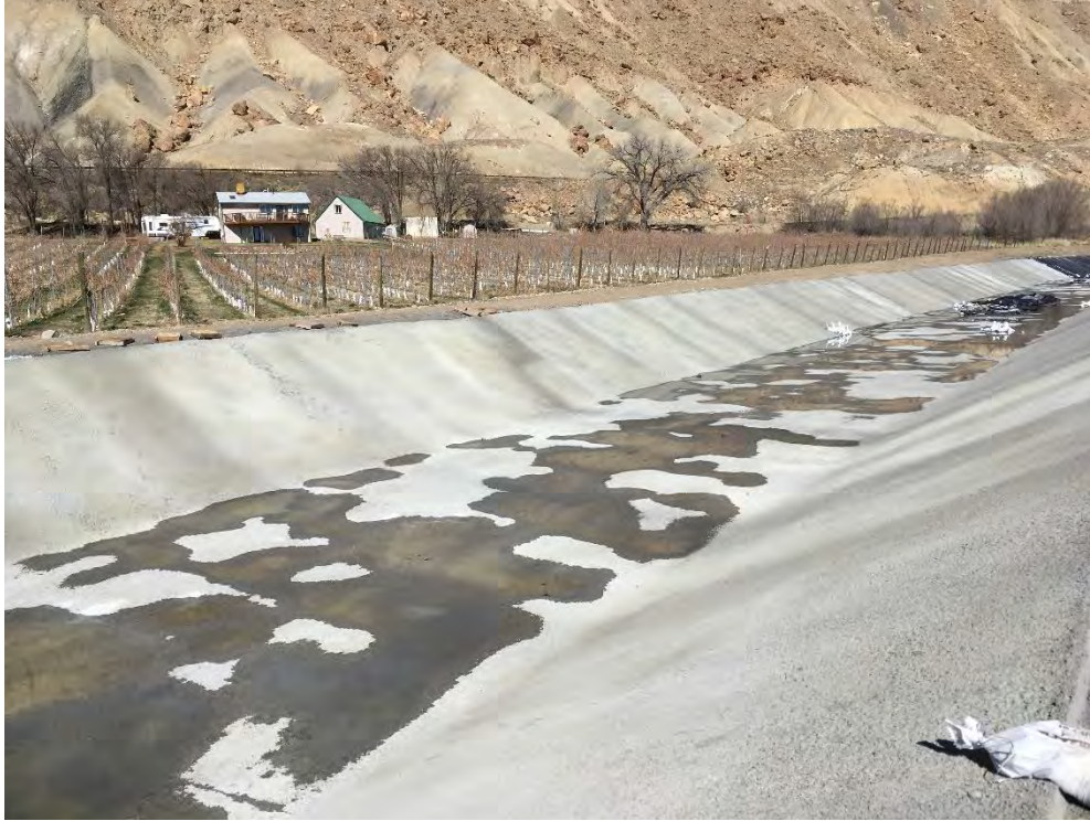
Figure 4.2.2. USBR Typical Canal Liner Cross Section Nearing Completion in Palisade, CO
