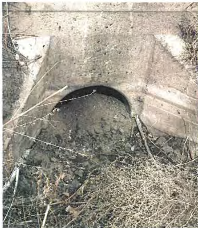
Figure 19: Plugged culvert at station 1353+05 just upstream of a timber bridge. Grand Valley Project, Colorado 2/21/2017
