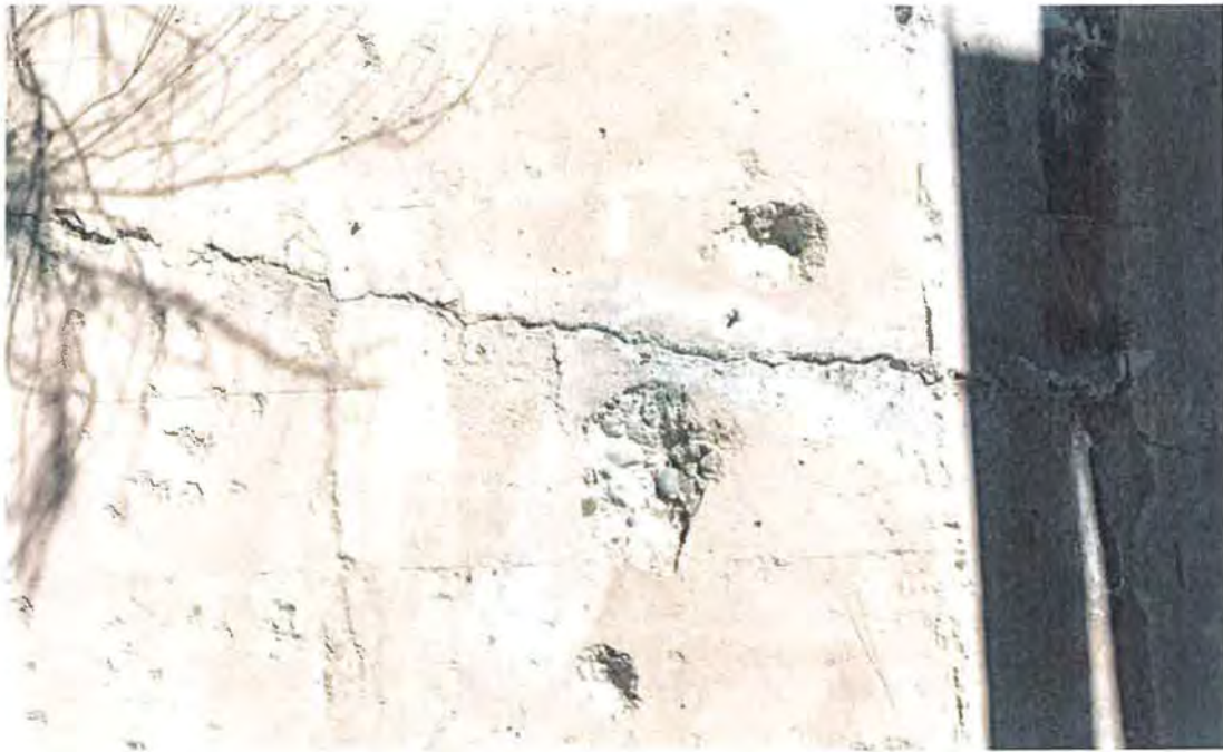
Figure 57: Significant cracking along the abutment of the 1220 flume O&M bridge. Grand Valley Project, Colorado 3/2/2017
