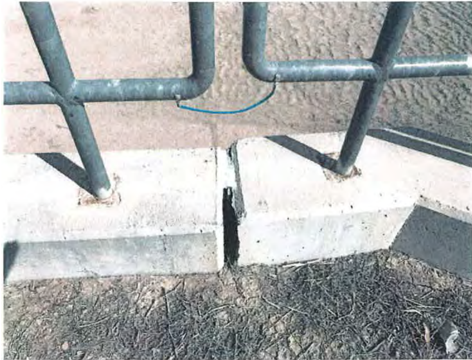
Figure 101: Possible movement of the wing walls of the A32 check structure. Grand Valley Project, Colorado 3/13/2017
