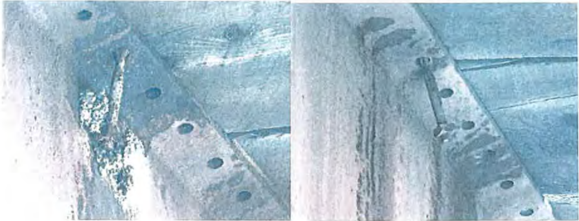
Figures 31 and 32: Close ups of the connection of the steel girder to the timber deck. Grand Valley Project, Colorado 2/21/2017
