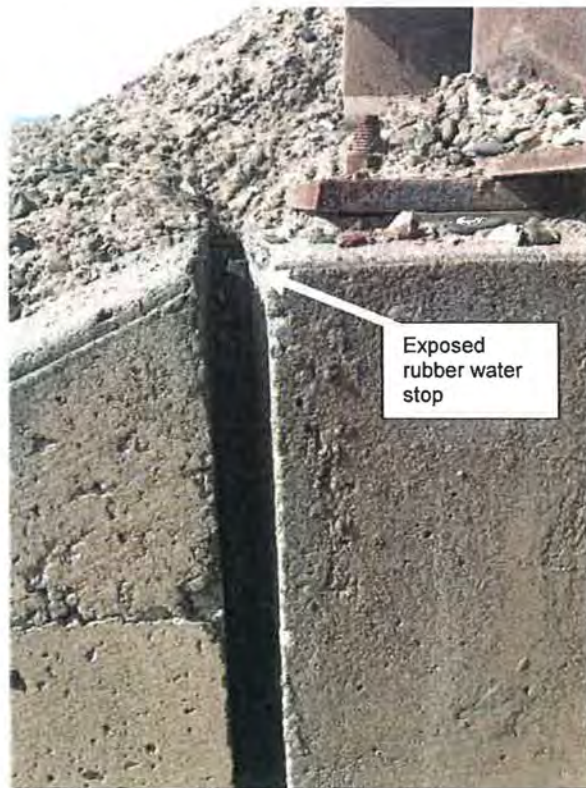
Figure 76: Possible differential settlement on the outlet wall for the Persigo Wash wasteway. Note the exposed rubber waterstop. Grand Valley Project, Colorado 3/13/2017
