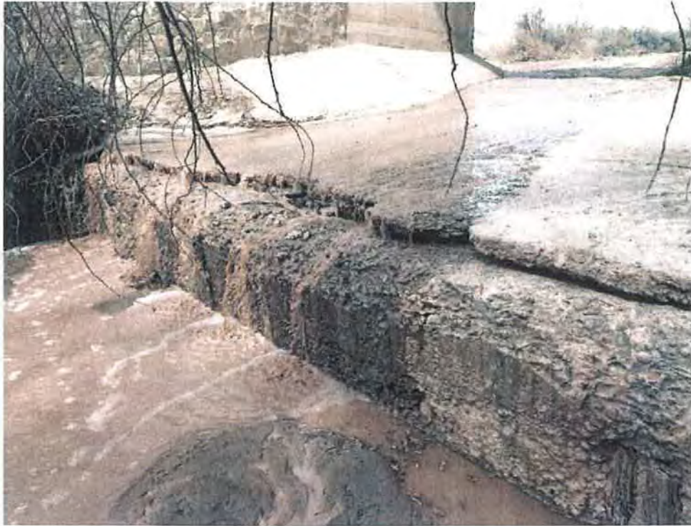
Figure 91: Undercutting on the Little Salt Wash channel. Grand Valley Project, Colorado 3/13/2017
