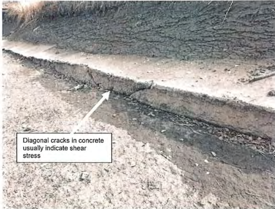
Figure 38: Shear cracks on the concrete lining. Grand Valley Project, Colorado 2/21/2017
