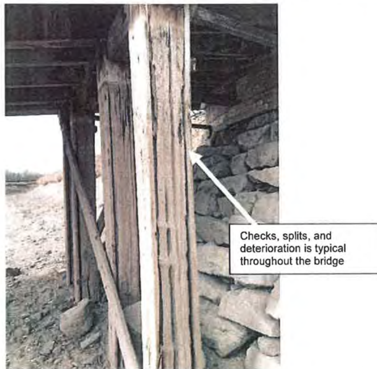
Figure 23: Checks, splits, and deterioration of the timber is typical. Grand Valley Project, Colorado 2/21/2017
