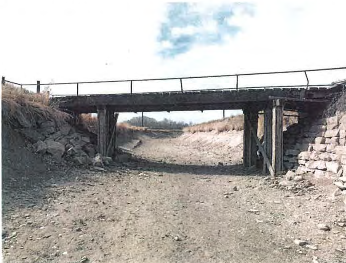
Figure 21: Overall view of the timber bridge at station 1354+52. Grand Valley Project, Colorado 2/21/2017
