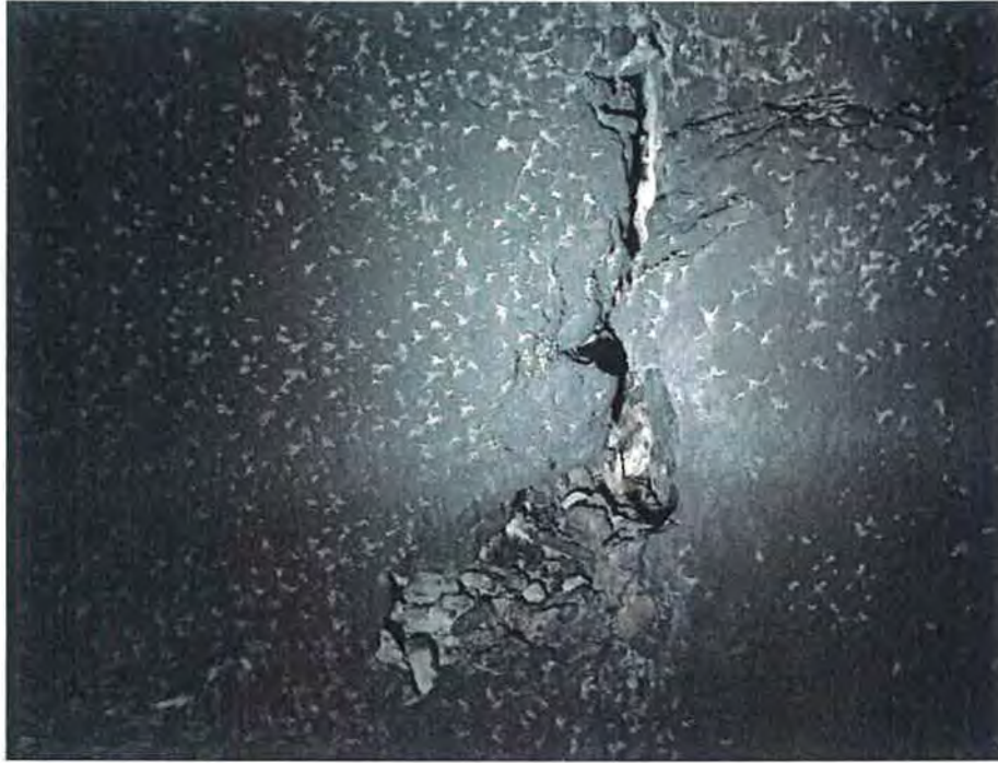
Figure 5: Significant cracking along the wall of Tunnel 3. Grand Valley Project, Colorado 3/1/2017.
