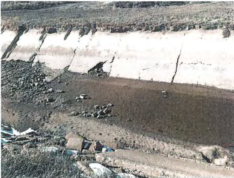
Figure 47: Damaged lining near Indian Wash. Grand Valley Project, Colorado 3/1/2017
