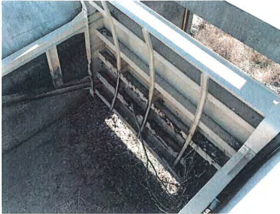
Figure 81: Rust on the downstream side of the radial gate for the A 21 ½ check structure. Grand Valley Project, Colorado 3/2/2017
