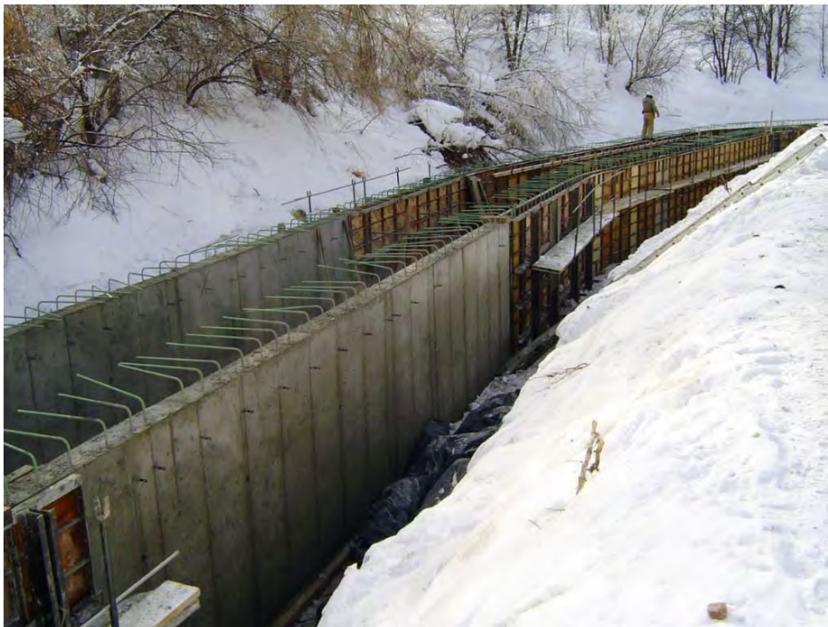
Figure 4.5.2. Construction Process for Cast-In-Place Concrete Box Culvert
