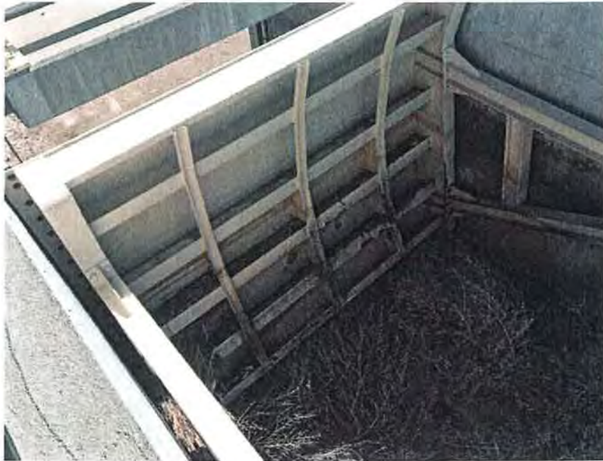
Figure 85: Rust on the downstream end of the A27 check structure radial gate. Grand Valley Project, Colorado 3/2/2017
