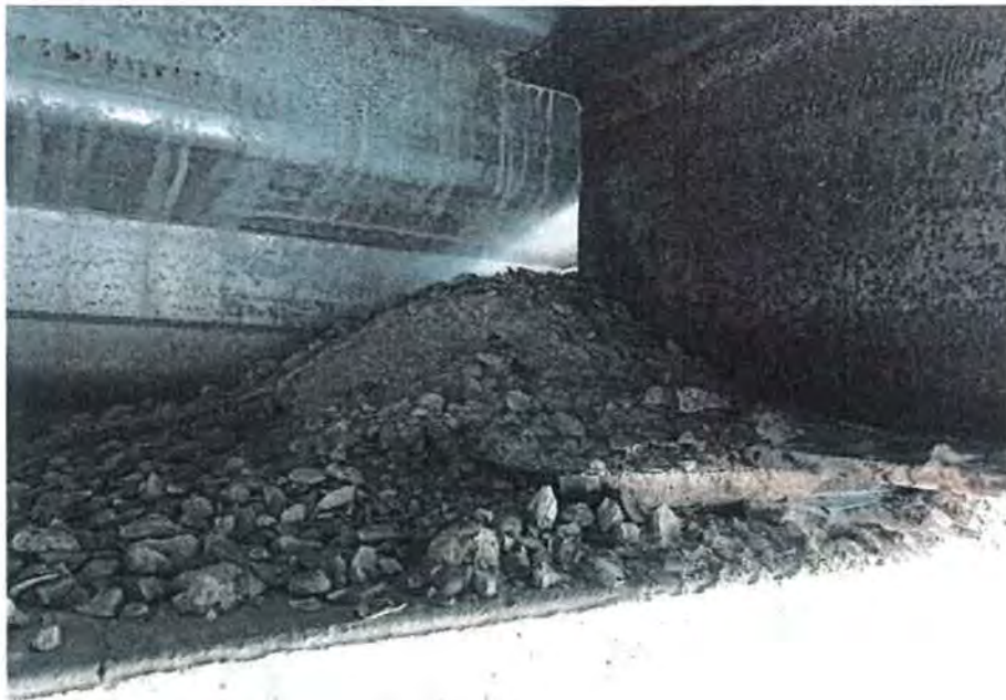
Figure 77: Possible differential settlement on the outlet wall for the Persigo Wash wasteway. Grand Valley Project, Colorado 3/13/2017
