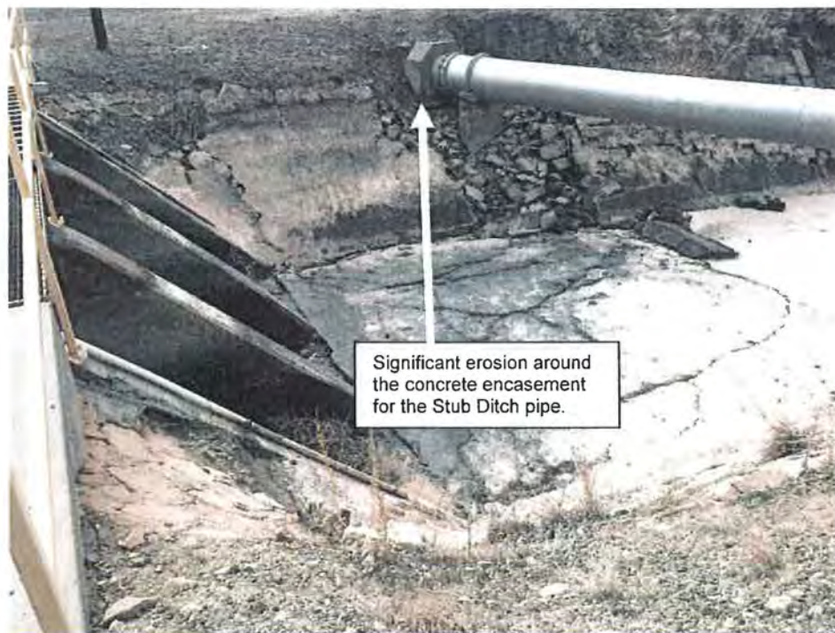
Figure 14: The right bank downstream of the Langemann gate at tunnel 3. Significant erosion has occurred around the concrete encasement of the Stub ditch pipe. Grand Valley Project, Colorado 2/21/2017
