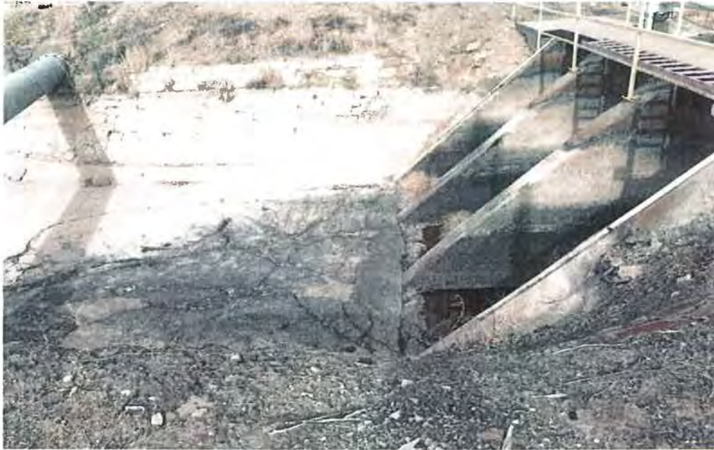
Figure 9: Looking at the downstream end of the Langemann gate at the tunnel 3 outlet. Photo was taken from the left (facing the direction of flow; typical) bank looking towards the right bank. Note the cracking and section loss in the concrete invert. Grand Valley Project, Colorado 2/21/2017.
