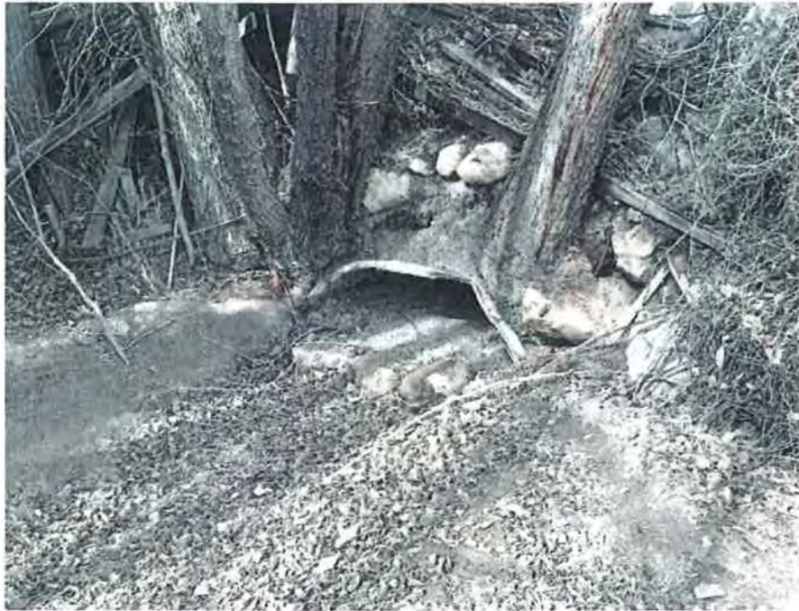
Figure 20: Plugged culvert at station 1361+55. Grand Valley Project, Colorado 2/21/2017
