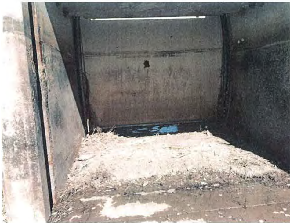
Figure 61: Rust on the radial gate of the A15 check structure. Grand Valley Project, Colorado 3/2/2017
