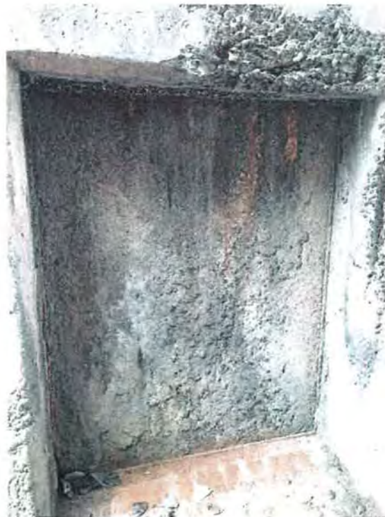
Figure 74: Spalling and rust on the gate of the Persigo Wash wasteway. Grand Valley Project, Colorado 3/13/2017
