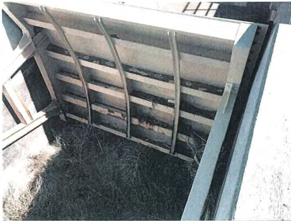
Figure 102: Rust on the downstream side of the A32 check structure radial gate. Grand Valley Project, Colorado 3/2/2017
