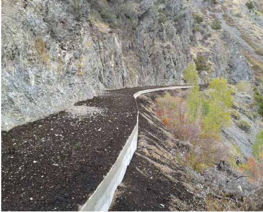
Figure 4.4.2. Installed Pre-Cast Box Culvert with No Cover
