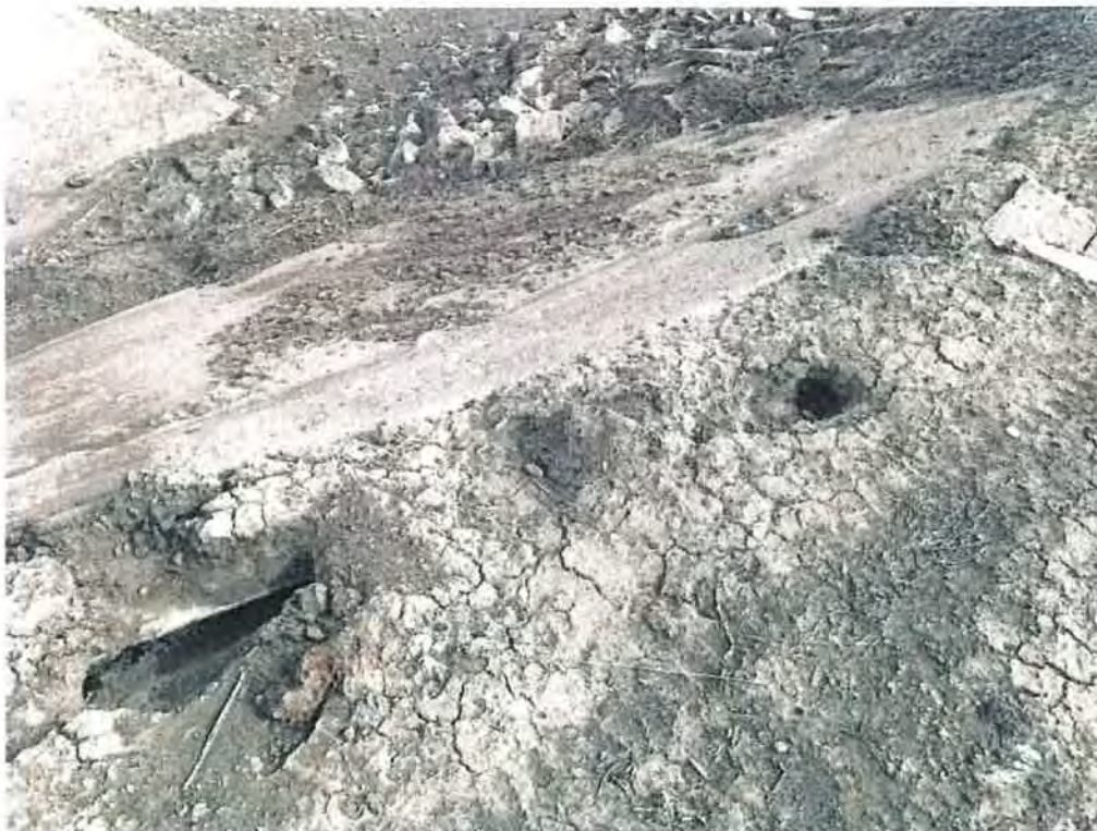
Figure 86: Erosion around the concrete wall of the A27 check structure. Grand Valley Project, Colorado 3/13/2017
