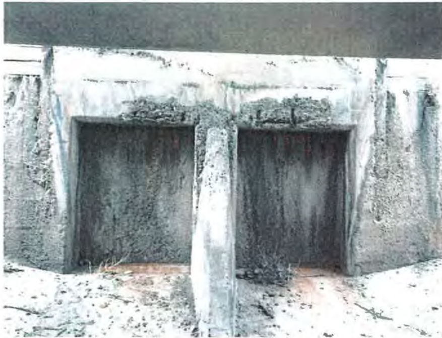
Figure 75: Exposed rebar on the wasteway structure near Persigo Wash. Grand Valley Project, Colorado 3/13/2017
