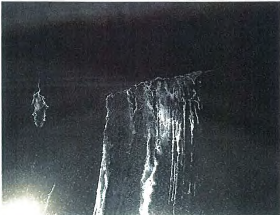
Figure 6: Some of the cracking shows what appears to be efflorescence. This seemed to be more prevalent near the end (downstream) of the tunnel. Grand Valley Project, Colorado 3/1/2017.
