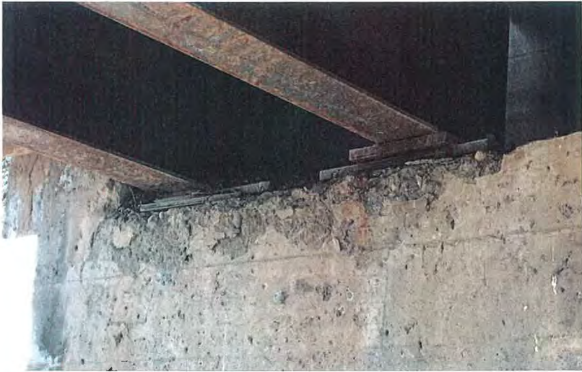
Figure 55: Section loss at the bearing pads. Note that one of the bearing pads is offset and may not be functioning properly. Grand Valley Project, Colorado 3/2/2017
