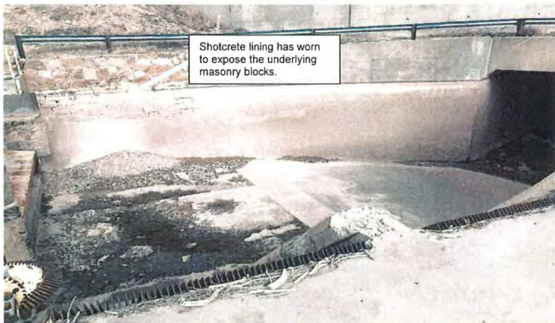
Figure 12: Looking at the downstream end of the Tunnel 3 outlet. Photo was taken from the left bank looking towards the right bank. Note the shotcrete lining has worn enough to expose the underlying masonry blocks. Grand Valley Project, Colorado 2/21/2017.
