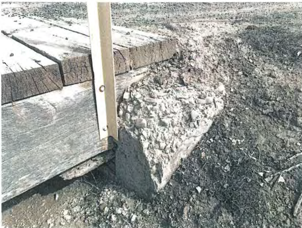
Figure 98: Spalling on the Little Salt Wash O&M bridge abutment. Grand Valley Project, Colorado 3/13/2017
