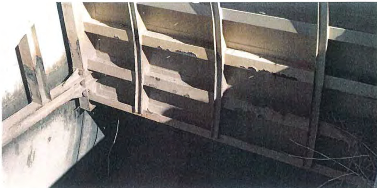
Figure 44: Downstream side of the Lewis Wash radial gate. Grand Valley Project, Colorado 3/1/2017
