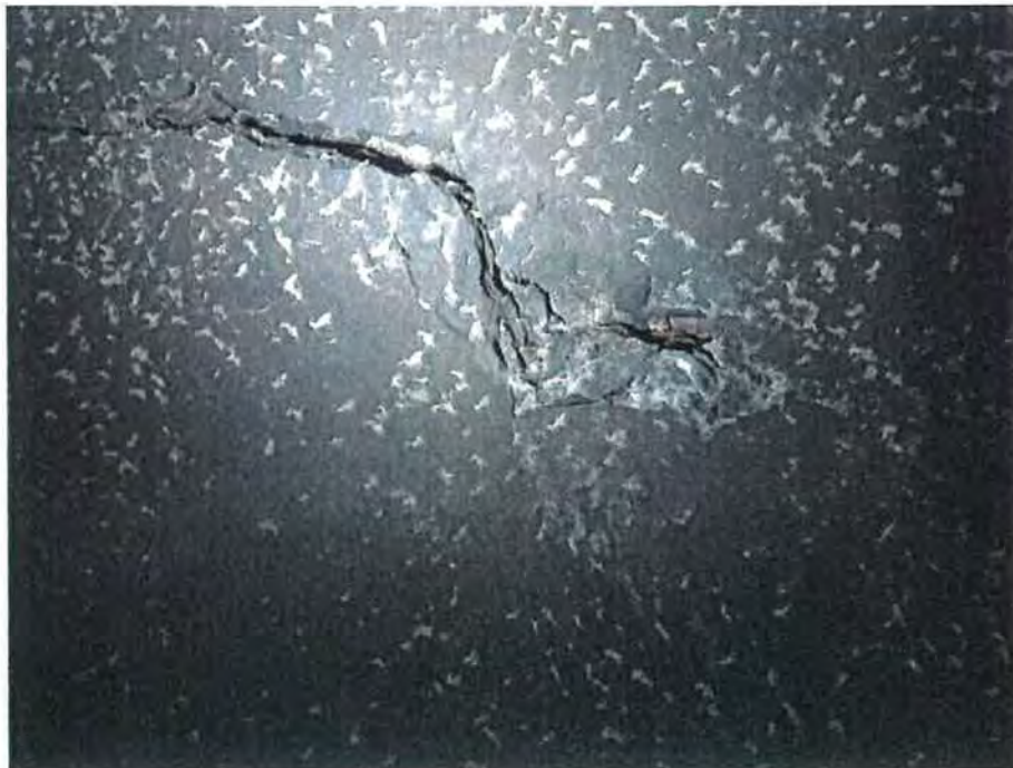
Figure 4: Significant cracking along the wall of Tunnel 3. The timber cribbing is exposed at several of the cracks. Grand Valley Project, Colorado 3/1/2017.
