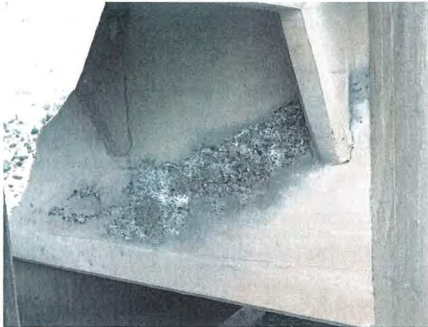
Figure 73: Spalling on the wasteway structure near Persigo Wash. Grand Valley Project, Colorado 3/13/2017
