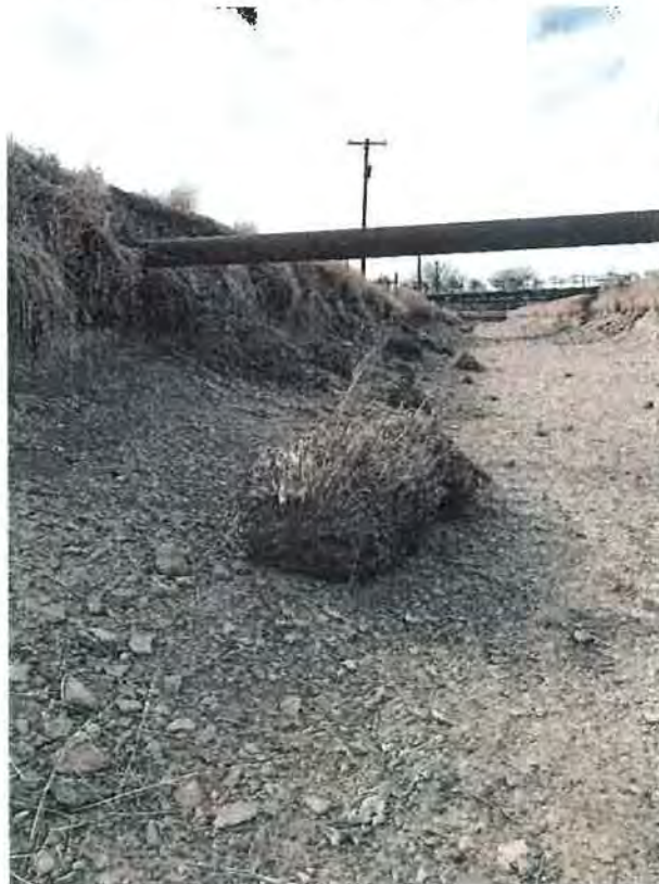
Figure 35: Sloughing along the banks. Grand Valley Project, Colorado 2/21/2017
