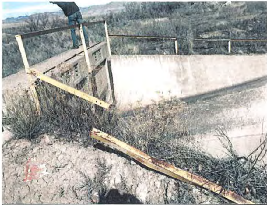
Figure 93: Damaged railing around the Little Salt Wash siphon. Grand Valley Project, Colorado 3/13/2017
