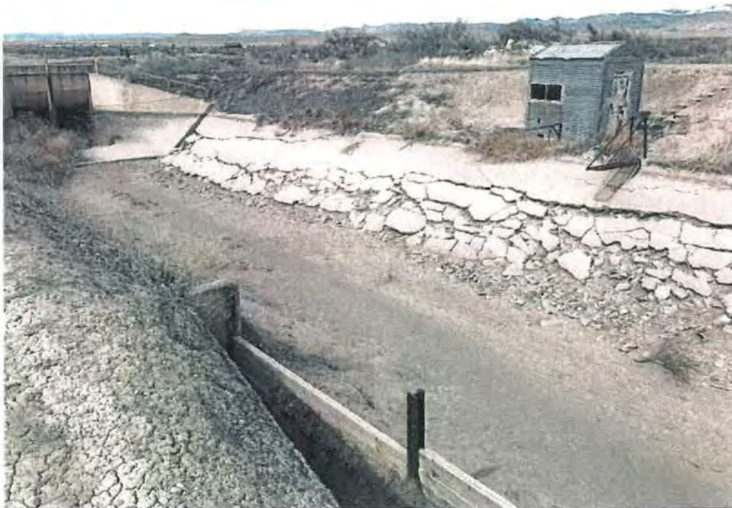
Figure 94: Deteriorated concrete lining upstream of the Little Salt Wash siphon. Grand Valley Project, Colorado 3/13/2017
