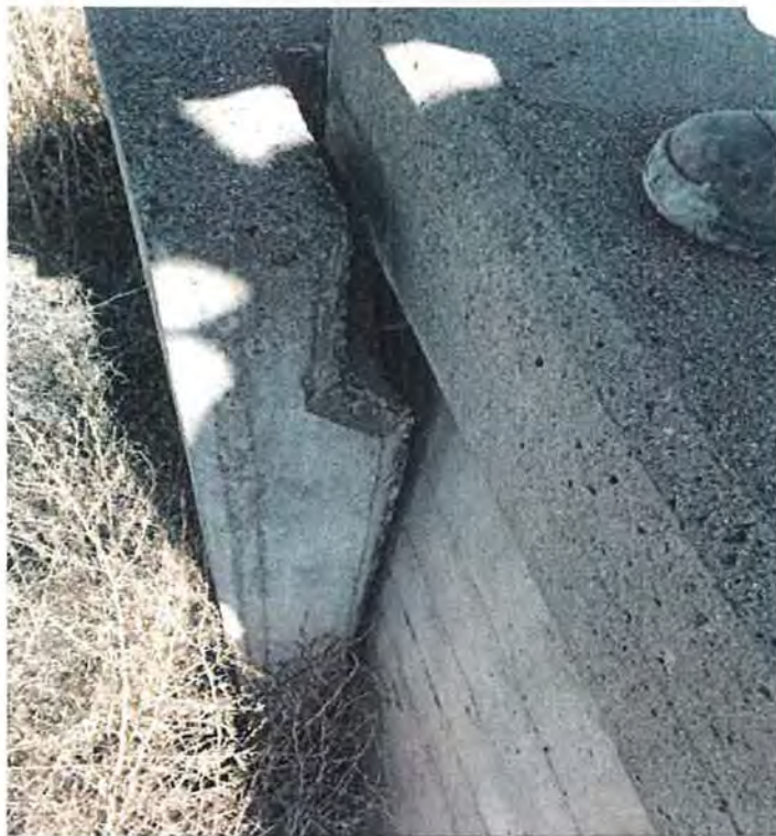
Figure 65: Offset at the expansion joint of the 1270 flume. Grand Valley Project, Colorado 3/2/2017
