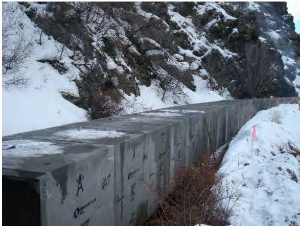
Figure 4.4.1. Installation of Pre-cast Box Culvert
