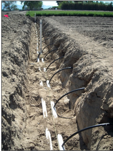
Fig. 2. Two subsurface drip zones with flush valves and drip lines exiting the main lines at the Colorado State University Western Colorado Research Center at Fruita.
