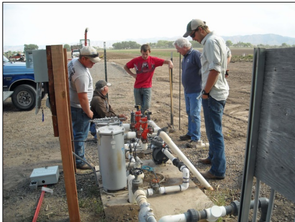
Fig. 3. Pumping and filter station for the subsurface drip irrigation system at the Colorado State University Western Colorado Research Center at Fruita.
