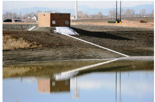
Figure 5 - Gravel Pit Pump Station near Fort Collins, CO
