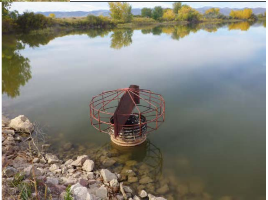
Photo 8. Service Spillway
