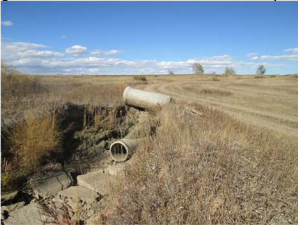
Downstream End of Existing 30-Inch RCP Inlet
