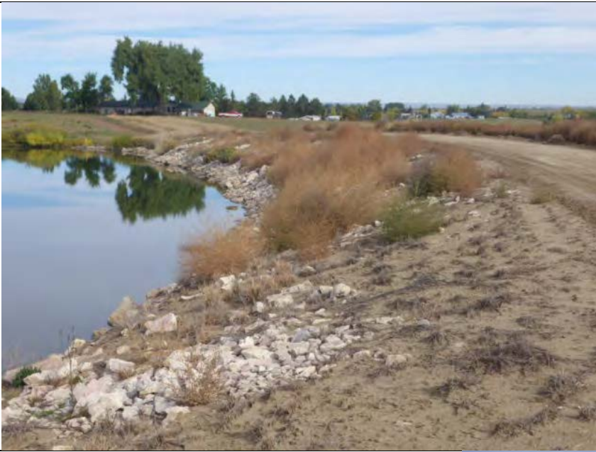
Photo 1. Upstream slope with some riprap and some vegetation
