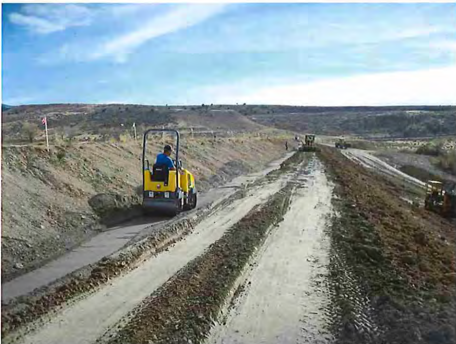
Photo #30: October 28, 2016 – Filter sand and embankment fill operations.
