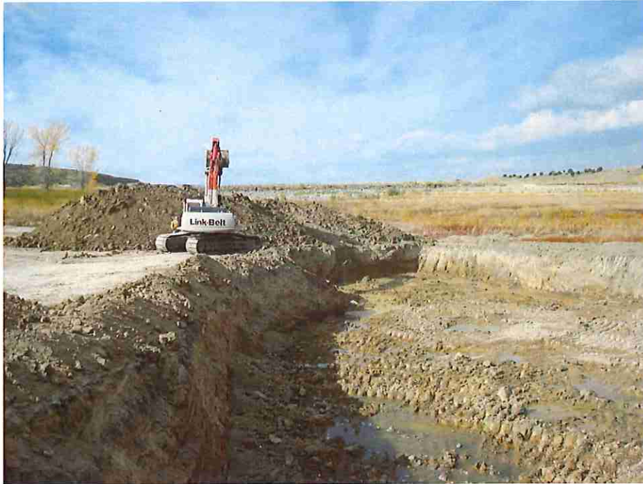
Photo #23: October 17, 2016 – Photo showing the borrow area within the reservoir pool area. The borrow area was towards the south end of the reservoir.
