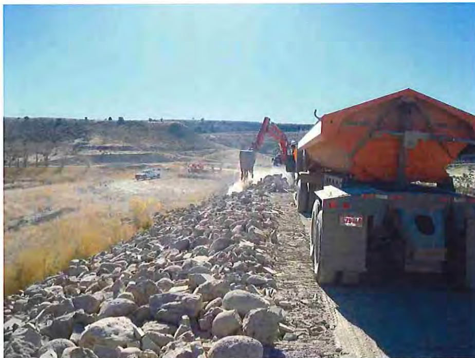
Photo #34: November 15, 2016 – Riprap placement along the upstream face of the dam.
