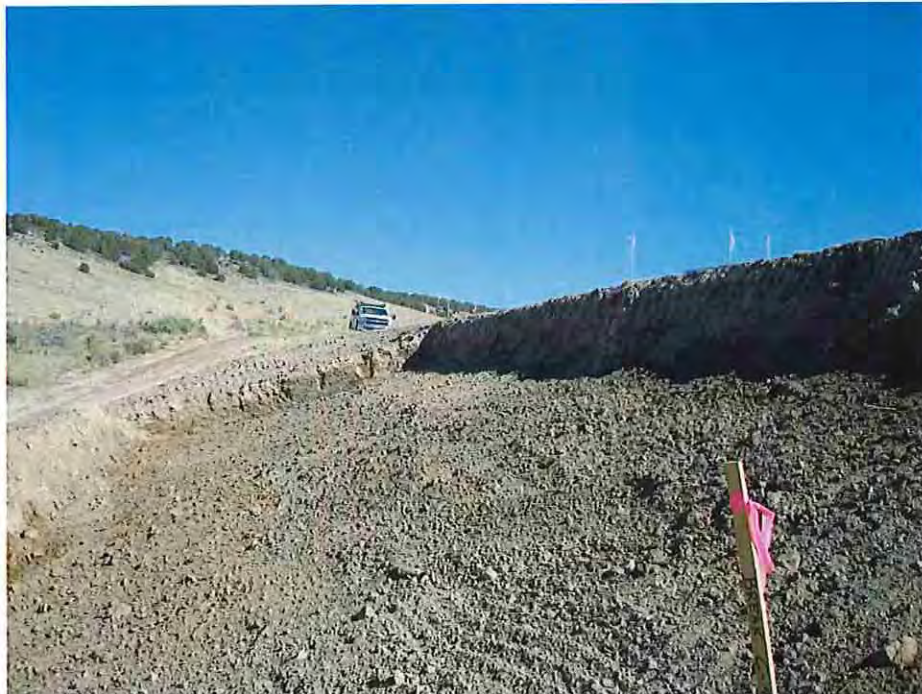
Photo #4: September 8, 2016 – Photo showing the over-excavation completed at the north end of the dam to accommodate the filter sand layer and the embankment fill. The same was done at the south end of the dam as well. This was done so the new embankment fill would tie into the existing dam grades at each end.
