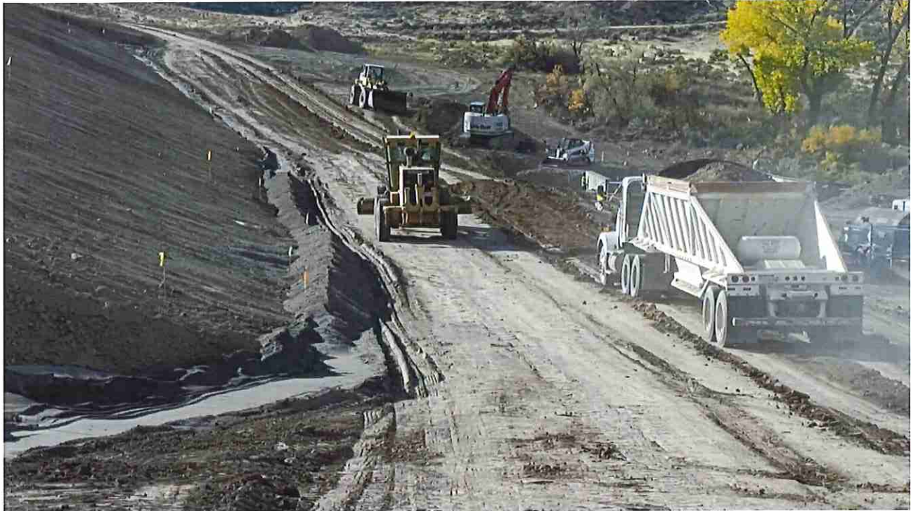
Photo #25: October 18, 2016 – Placement operations of the Embankment fill and filter sand.
