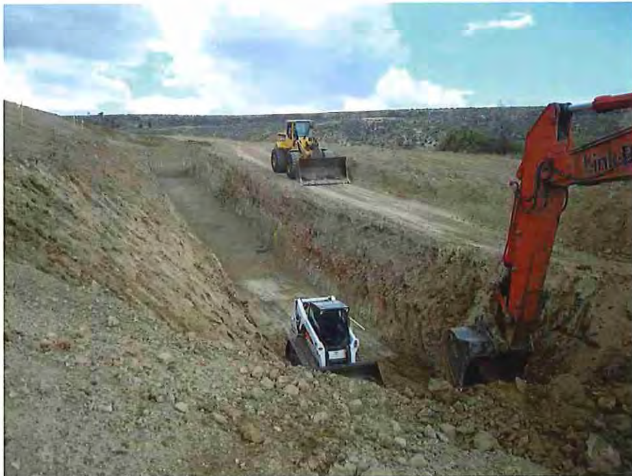
Photo #6: September 14, 2016 – Excavation begins on the south toe-drain.
