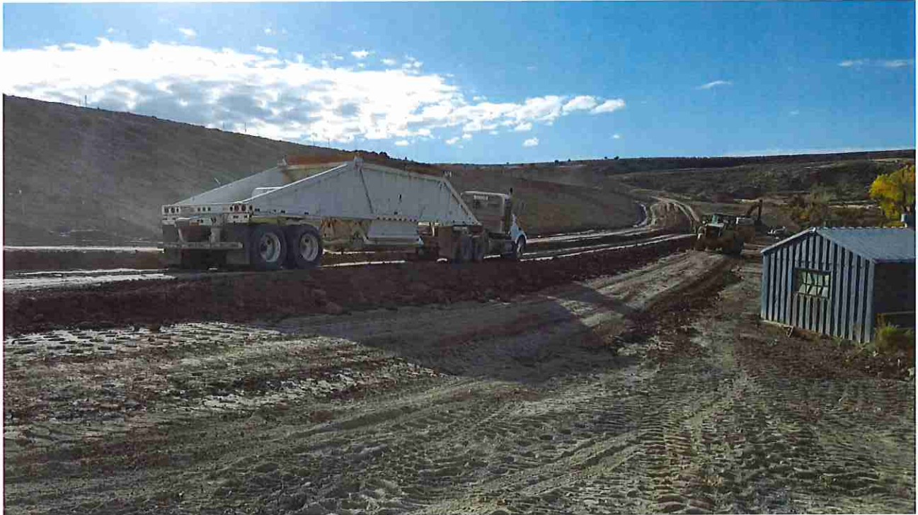
Photo #24: October 18, 2016 – Embankment fill operations.
