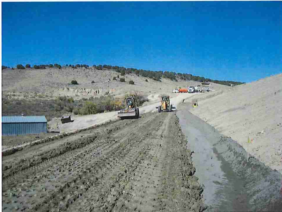
Photo #26: October 20, 2016 – Grading and compaction operations of the embankment fill.
