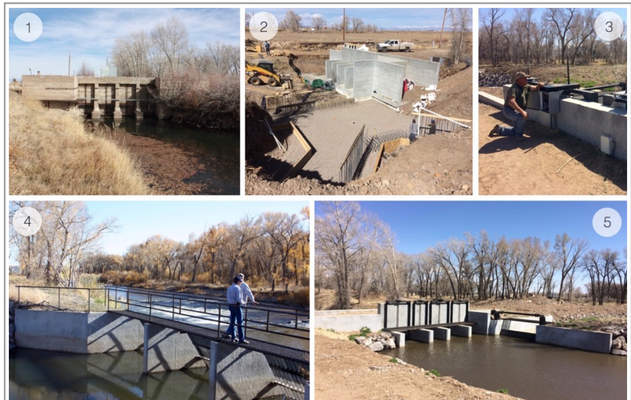
Figure 5: Headgate Replacement 1) Prairie Ditch headgate before; 2) Headgate and sluice gate construction; 3) Adjusting automation on new headgate; 4) Completed trash rack; 5) Completed Prairie Ditch headgate and sluice gate.
