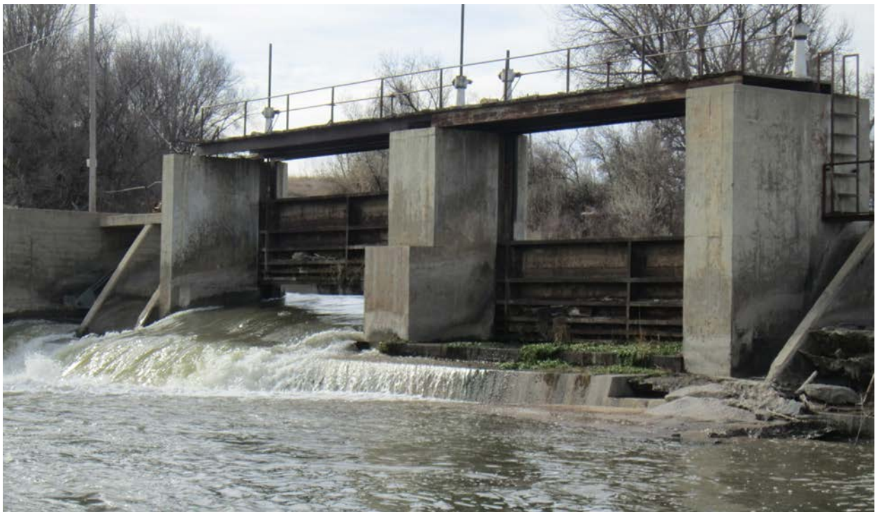
Photo No. 10 South Section. View from downstream channel looking upstream at the spillway slide gate structure.
