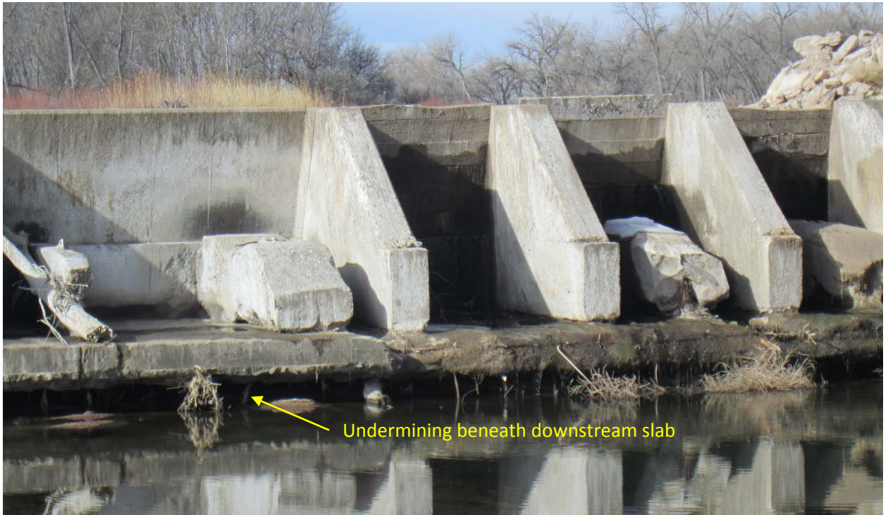
Photo No. 15 North Section. Closer view of the north buttress section, taken from the downstream channel.. Note, undermining (erosion) beneath the downstream slab.
