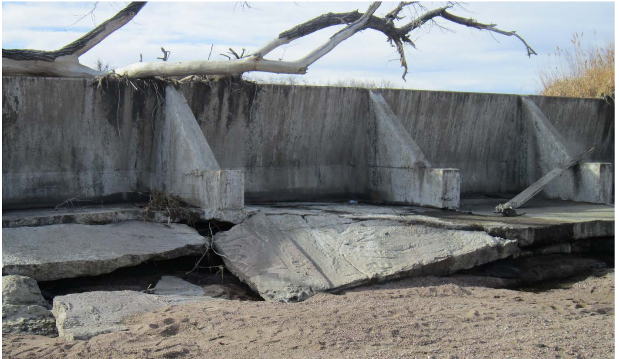
Photo No. 19 Diagonal Section. View of failed base slab, due to undermining (erosion) of foundation material from beneath the slab.
