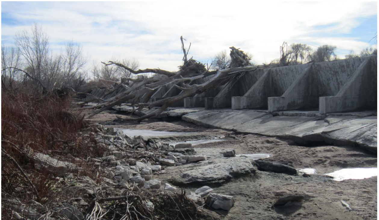
Photo No. 18 Diagonal Section. View shows typical undermining erosion that resulted in collapse of base slab.
