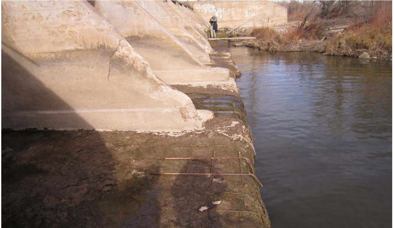
Photo No. 25 South Section. View showing exposed reinforcement in bottom slab of the south buttress section.
