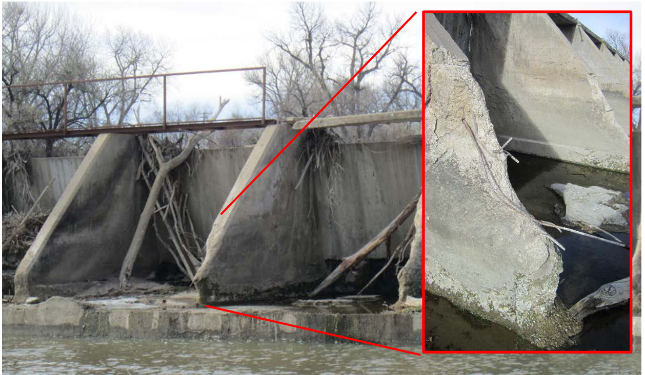
Photo No. 23 South Section. View shows concrete deterioration of buttress (inset).
