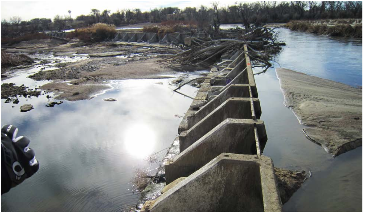
Photo No. 1 North Buttress Section. View of taken from left (north) abutment, looking south. There is significant reservoir sedimentation upstream of the dam, and woody debris on the crest from previous flood events.
