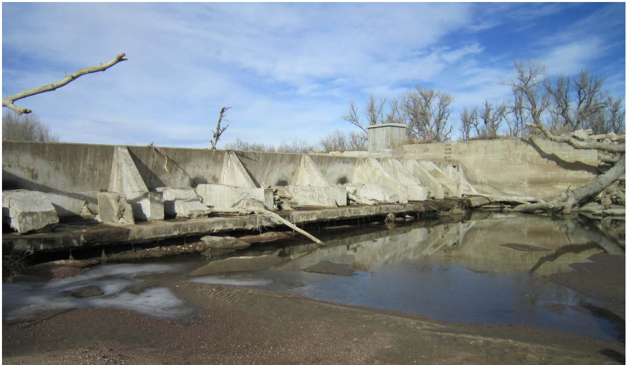
Photo No. 2 North Buttress Section. View of the upstream slab and buttresses, taken from the downstream channel.
