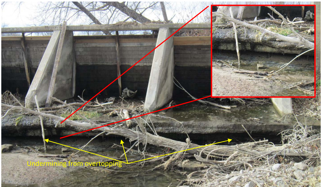
Photo No. 22 South Section. Closer view of the south buttress section, showing undermining (erosion) of foundation material beneath base slab. Note, the view shows exposed shear key (inset). .
