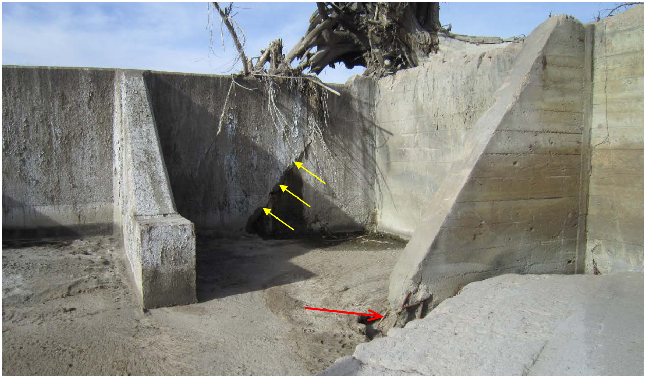
Photo No. 17 Transition Section. Seepage through construction joint in upstream slab, and deterioration at base of buttress.
