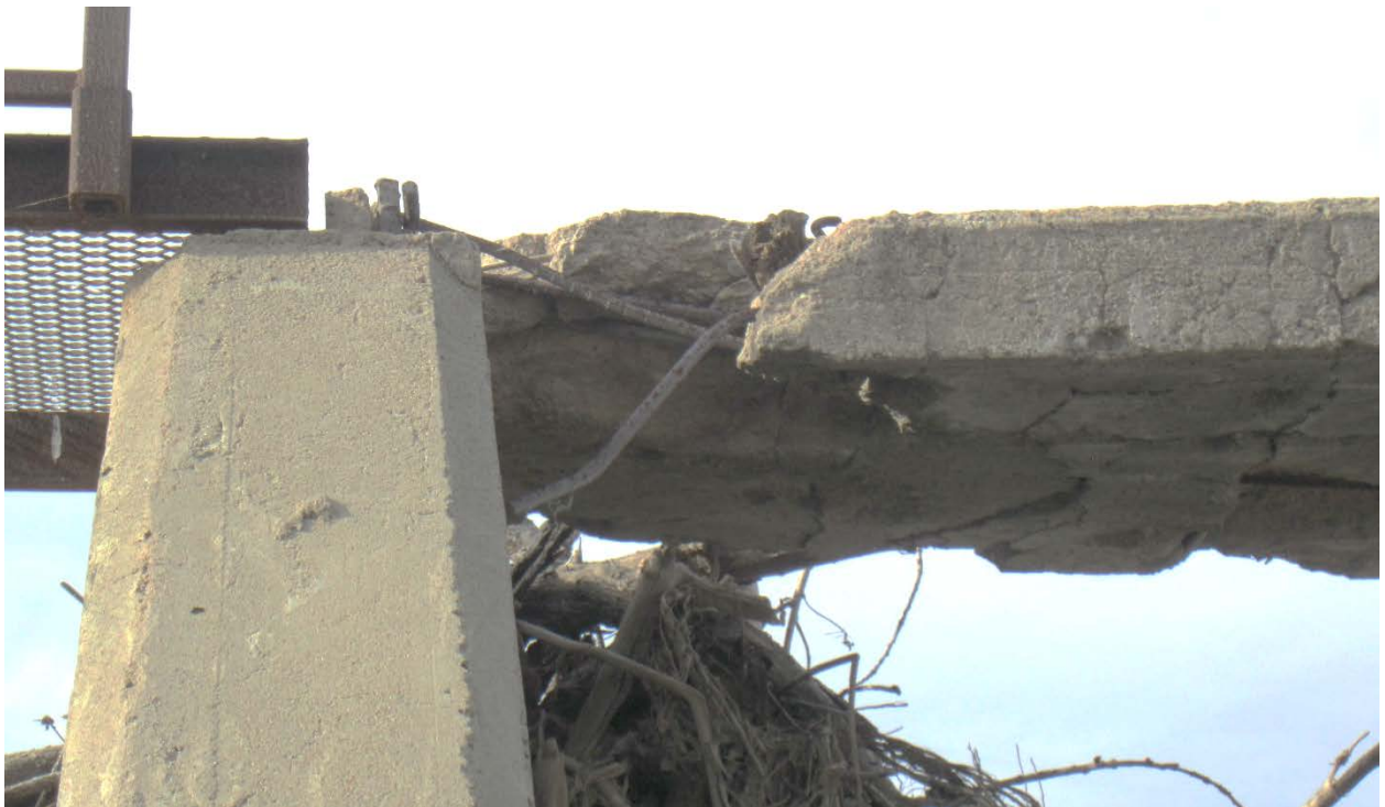
Photo No. 24 South Section. View showing deteriorated walkway that spans south buttresses and leads from the drop gate structure.
