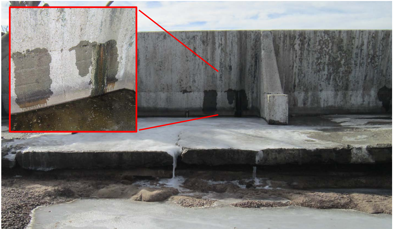
Photo No. 21 Diagonal Section. Inspection observed ice (from ponding) on the downstream slab in the central section as shown above. Inset photograph shows seepage through the upstream wall slab that caused the pool to develop.
