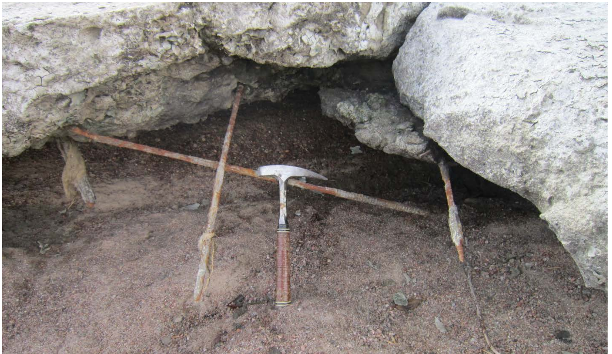
Photo No. 20 Diagonal Section. Closer view of the deterioration of base slab. Note, exposed and deteriorated reinforcement. .
