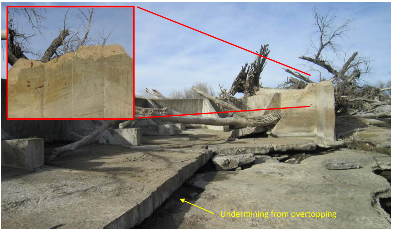
Photo No. 16 Transition Section. Deterioration and undermining on the transition section. Taken looking towards the north section. Inset shows close up view of typical deterioration along top of buttress and slab walls.
