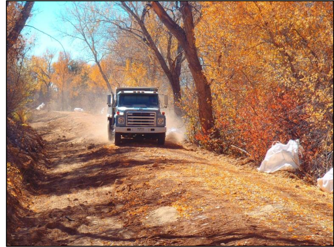
Photo 2. Bentonite and lime being staged along the 5,000-foot section to be lined.
