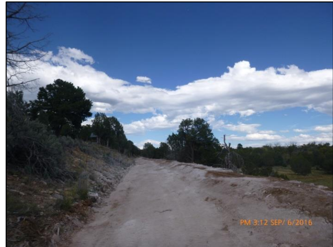
Photo 12. Completed lining project by amending the soil with approximately 440 cubic yards of clayey soils, 110 tons of bentonite, and 25 tons of lime.
