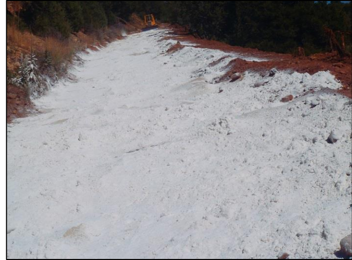
Photo 10. The lime will help bind bentonite to soil and as well as help to reduce rodents from burrowing in and along the ditch.
