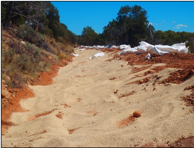
Photo 7. Bentonite was worked into the soil approximately 15 inches deep.
