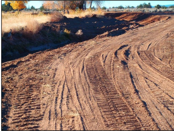
Photo 5. Re-shaping ditch by grading back some of the slopes to better retain the lining material.
