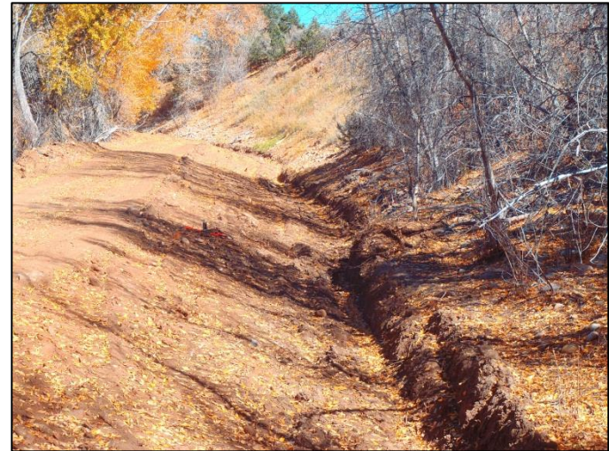
Photo 3. A section of the ditch that has been re-shaped prior to lining.
