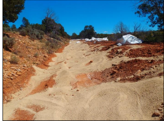
Photo 6. Applying layers of bentonite.
