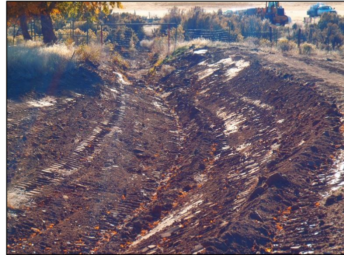
Photo 6. Ditch after removal of excessive weeds and re-shaping work.
