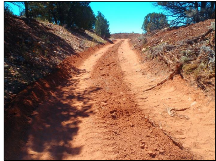
Photo 4. Beginning to re-work the ditch soil.
