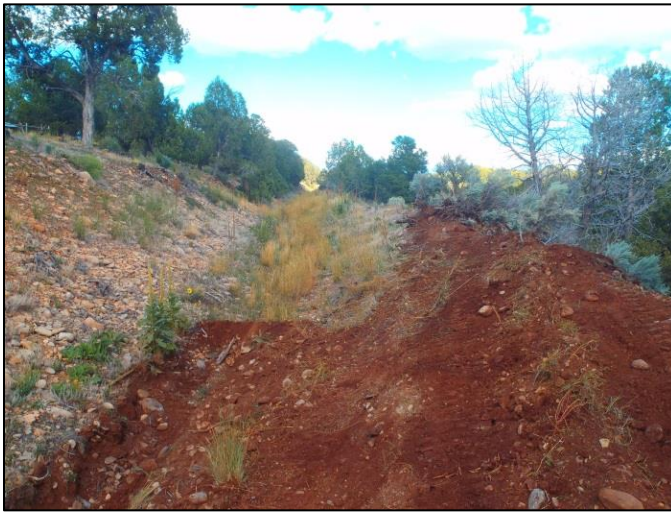
Photo 3. Removing vegetation in ditch.
