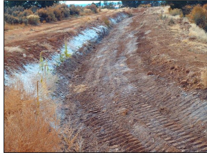
Photo 10. Soil amendments were incorporated into the upper 15 inches of existing soils to bind materials.
