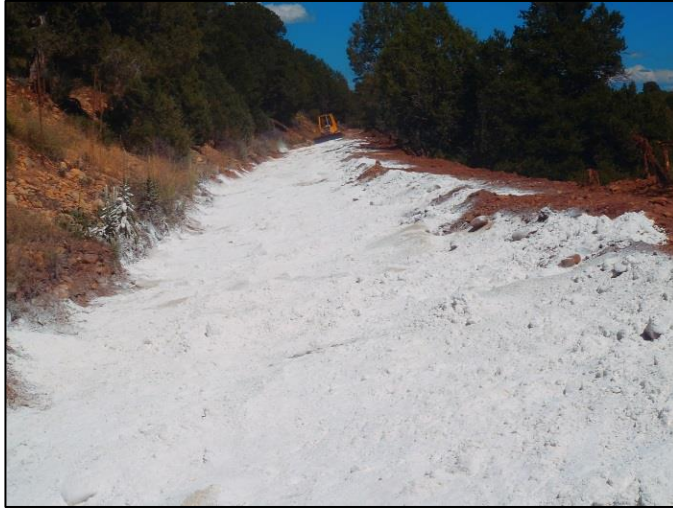
Photo 9. Lime being worked into the soil and bentonite.
