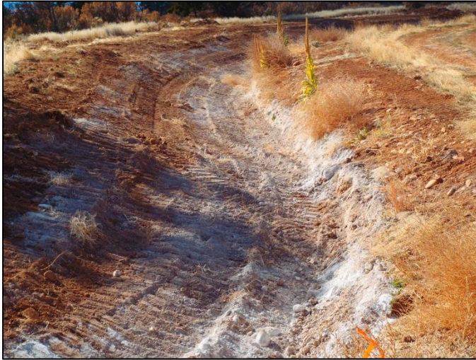
Photo 9. Completed ditch lining with soil amendments of bentonite and lime.
