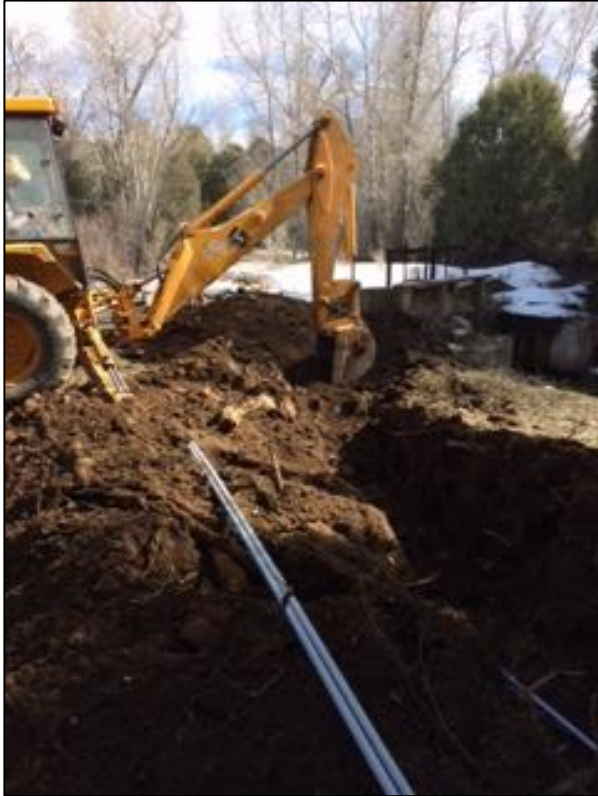
Photo 1. Digging the trench from the flume to the headgate.
