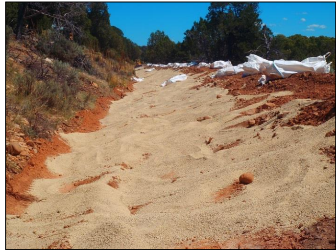
Photo 8. The natural moisture will help bind and seal the bentonite to the lime and clayey soil to help reduce leakage in the ditch.
