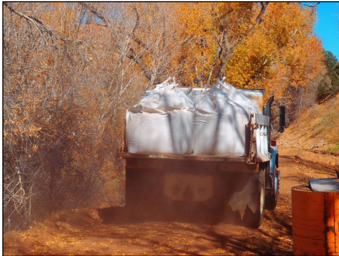
Photo 3. All material was delivered in approximate 1-ton TOTE bags, making placement more efficient.
