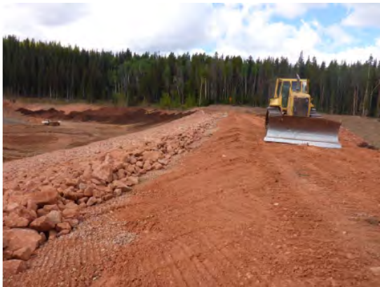
Figure 4 - Riprap Placement
