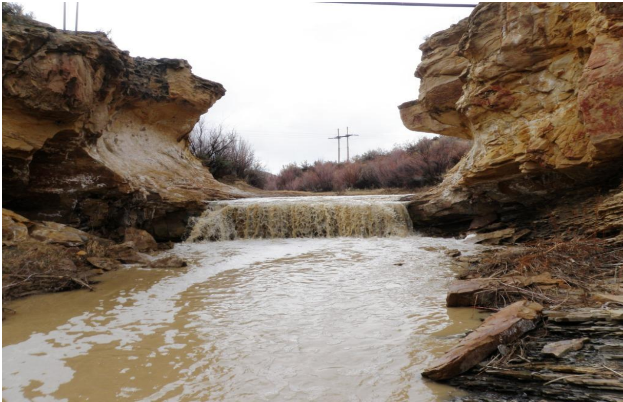
Large natural barrier 4.5 foot drop
