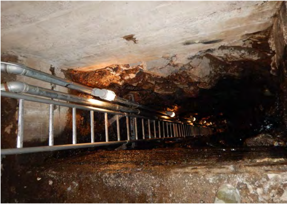
Photograph 5: February 24, 2016. Ladder, encasement pipe, and lighting in the vertical rock-cut shaft.
