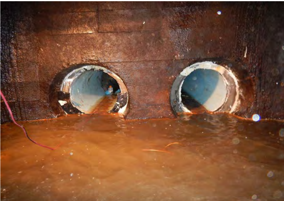
Photograph 10: February 19, 2016. Annular Space between 24-inch and 30-inch diameter pipes following secondary grouting.
