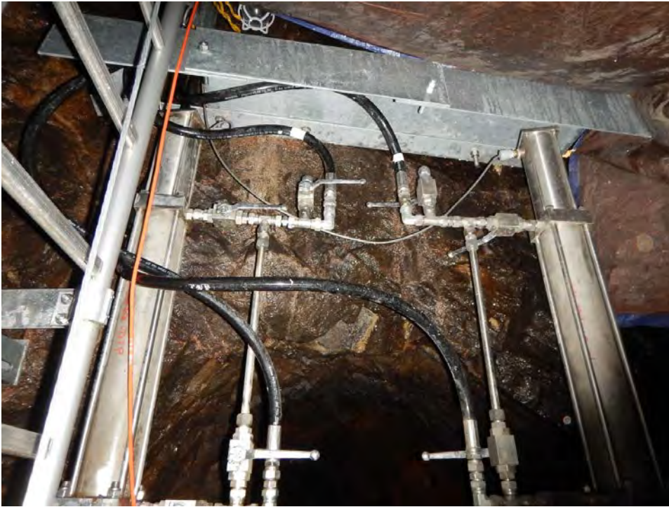
Photograph 12: May 3, 2016. Knife gate valve hydraulic cylinders, hydraulic manifolds, flexible hydraulic control tubing, and removable shield.
