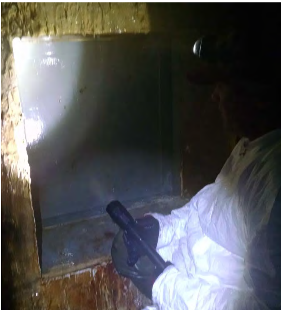
Photograph 17: June 21, 2016. 30-inch slide gate under full reservoir head. Springer leaks have been sealed.
