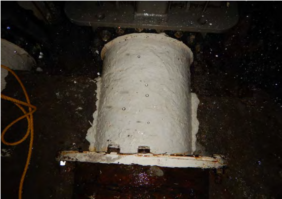
Photograph 9: June 7, 2016. 24-inch steel pipe coated with Aquatapoxy above the concrete cradle.
