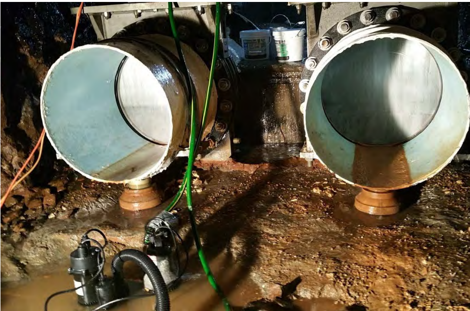
Photograph 8: June 14, 2016. Pipe supports and backfill concrete.
