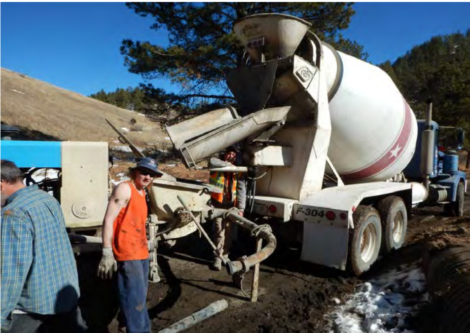
Photograph 6: February 9, 2016. Forces mobilized to place the concrete cradle for the 24-inch diameter steel pipes.
