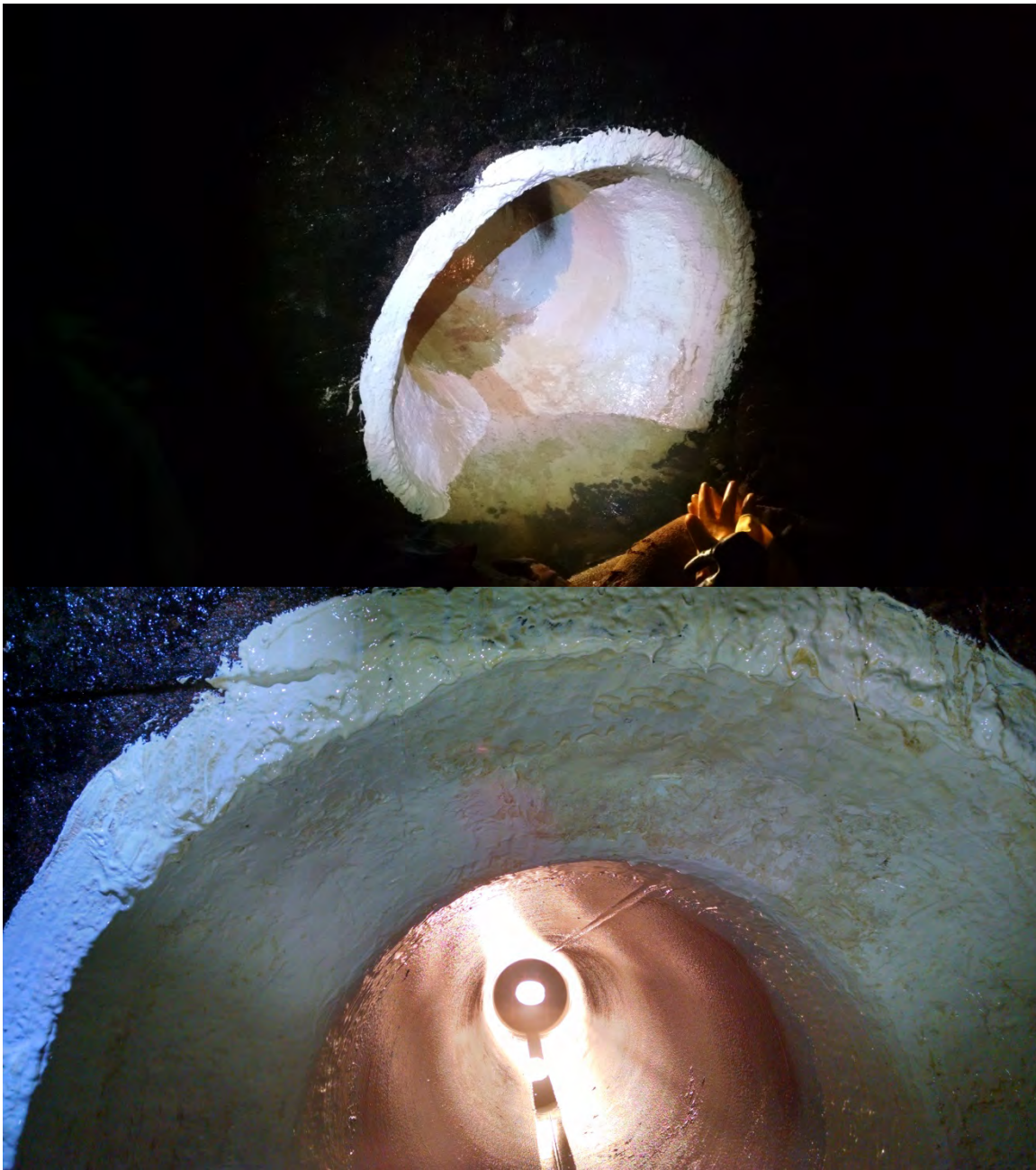
Photograph 11: June 21, 2016. Completed transition from the concrete bulkhead wall to the 24-inch diameter steel pipes.
