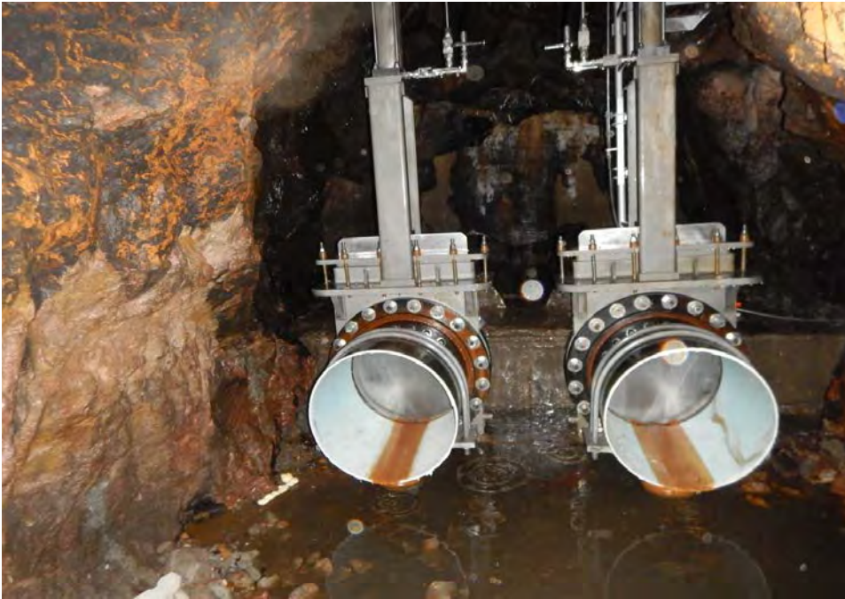
Photograph 7: March 2, 2016. 24-inch diameter pipes and concrete cradle.
