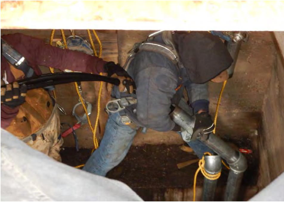
Photograph 3: January 31, 2016 Installation of flexible hydraulic tubing in the vertical rock-cut shaft.
