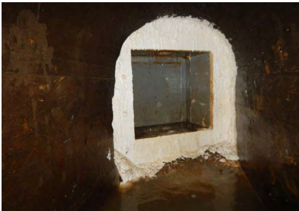
Photograph 16: March 2, 2016. Downstream face of the steel bulkhead plate, thimble, and 30-inch slide gate (first installation).
