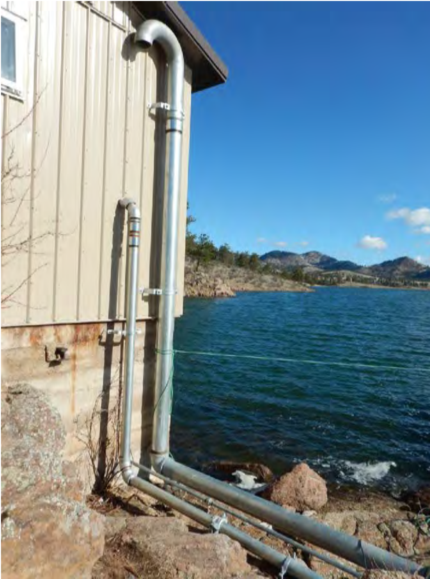
Photograph 19: May 3, 2016. Vent pipe and encasement pipe installed on the east wall of the valve house.
