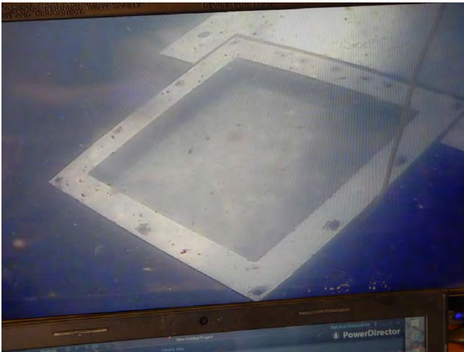
Photograph 15: May 4, 2016. 30-inch slide gate (second installation) coated with Aquatapox prior to installation.
