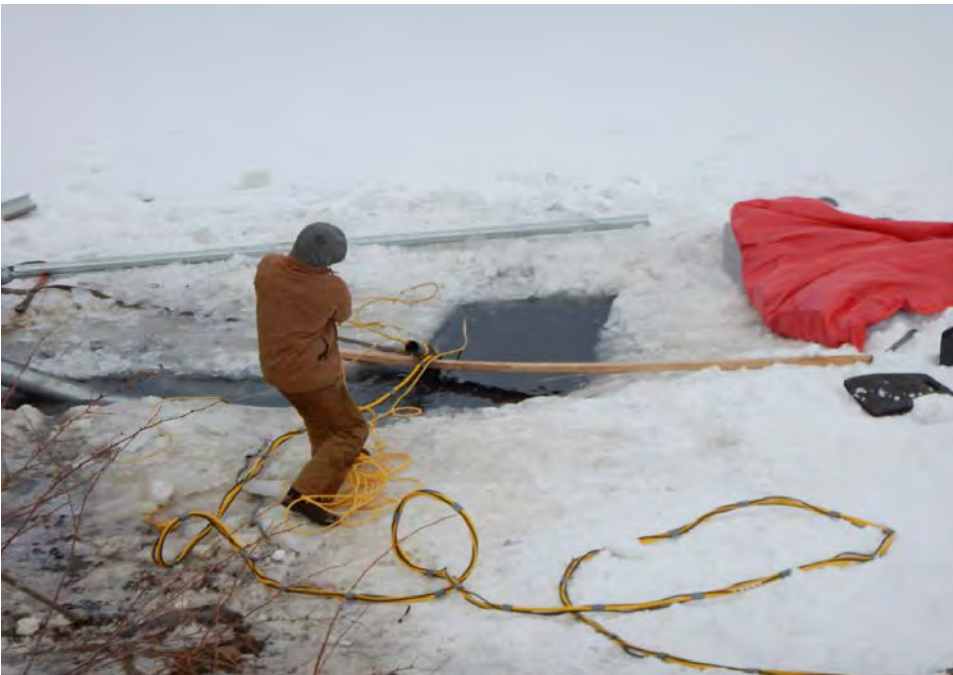
Photograph 2: February 6, 2016 Installation of flexible hydraulic tubing for the 30-inch slide gate.
