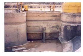
completely rebuilt or replaced with a more modern design. Each gate is uniquely designed and will require a review of the historical drawings and reissued before a local craftsman can rebuild them. More modern replacement options such as vertical lift gates could be used and will be easier to maintain in the future.
