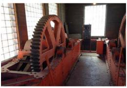
The existing Roller Dam has an overhead three phase service from Xcel Energy. The largest load on the dam is a motor-generator which converts AC power to DC power. The DC power is then used to operate the seven roller gate motors. Each roller gate motor is 10
