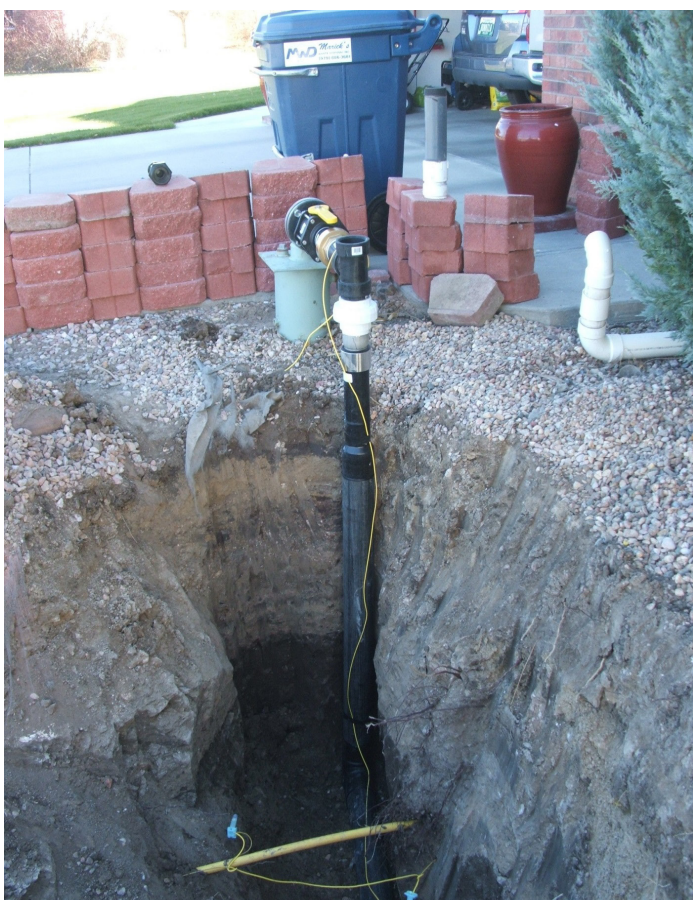
The St. John dewatering well as it is being tied into the permanent pipeline.
