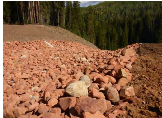
Figure 5 - Spillway Channel Riprap Armoring
