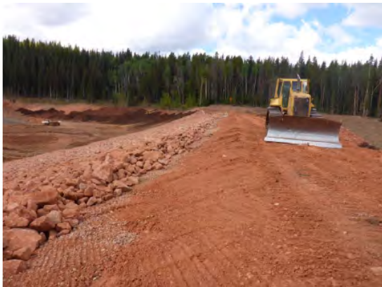
Figure 4 - Riprap Placement
