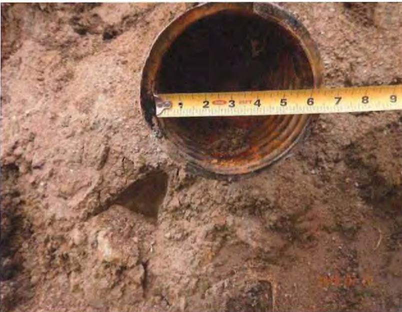
Photo 4 – Existing toe drain pipe exposed on the north side of the excavation.
