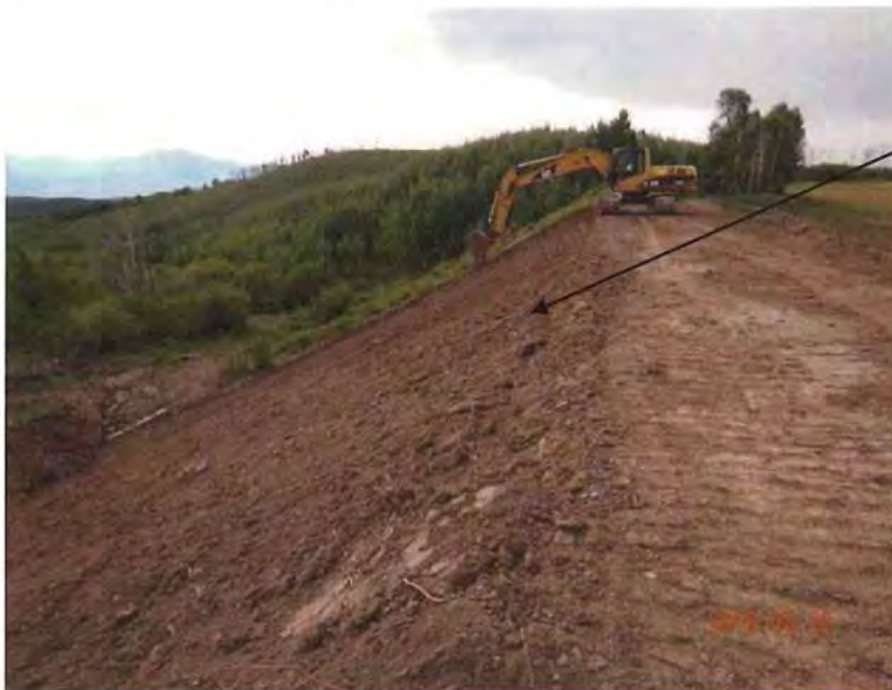
Photo 2 – Placing topsoil on the downstream slope.
