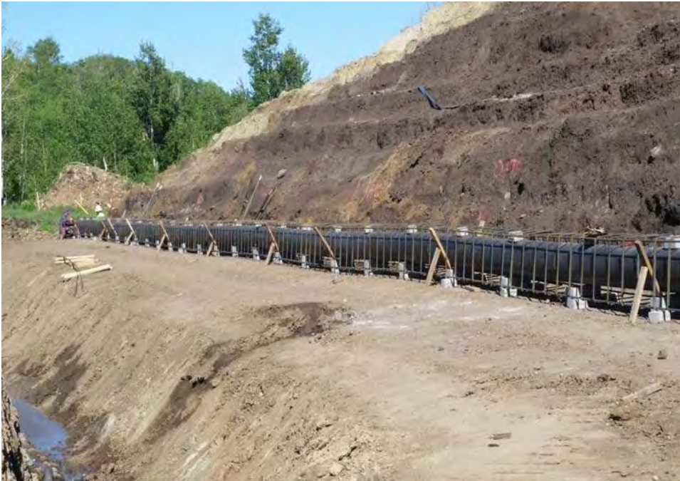
Photograph 25: HDPE conduit and encasement reinforcing steel in place.
