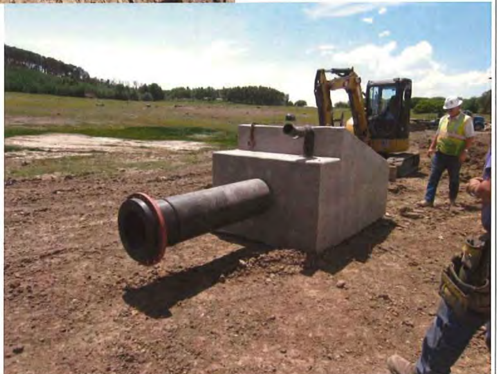
Flanged end on precast intake structure.
