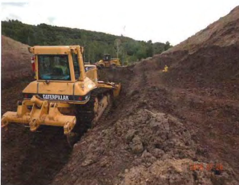
Photo 3 – Cutting existing embankment at new fill contact.
