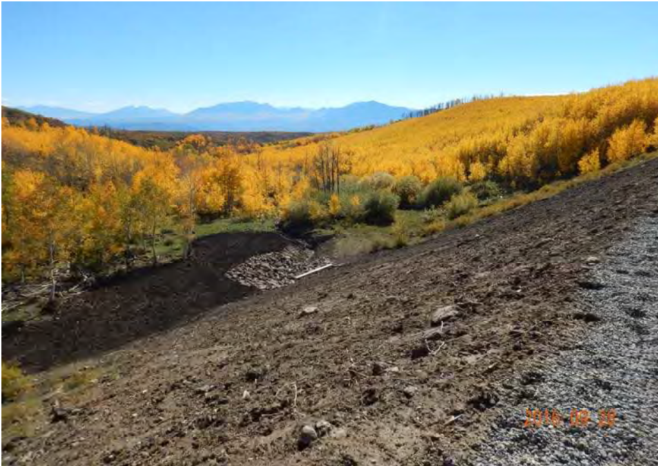
Photograph 23: Completed downstream slope and discharge channel.
