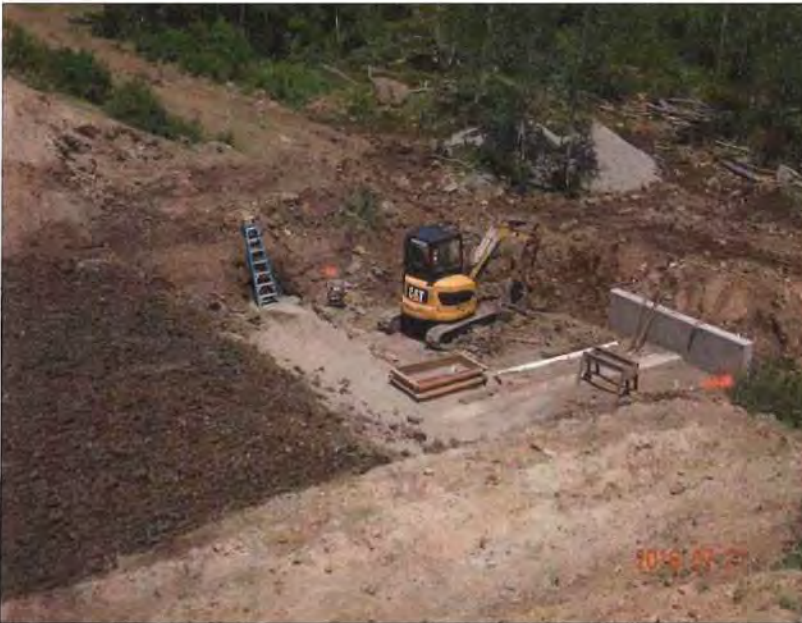
Photo 4 – Filter collar to about Elevation 8738.
