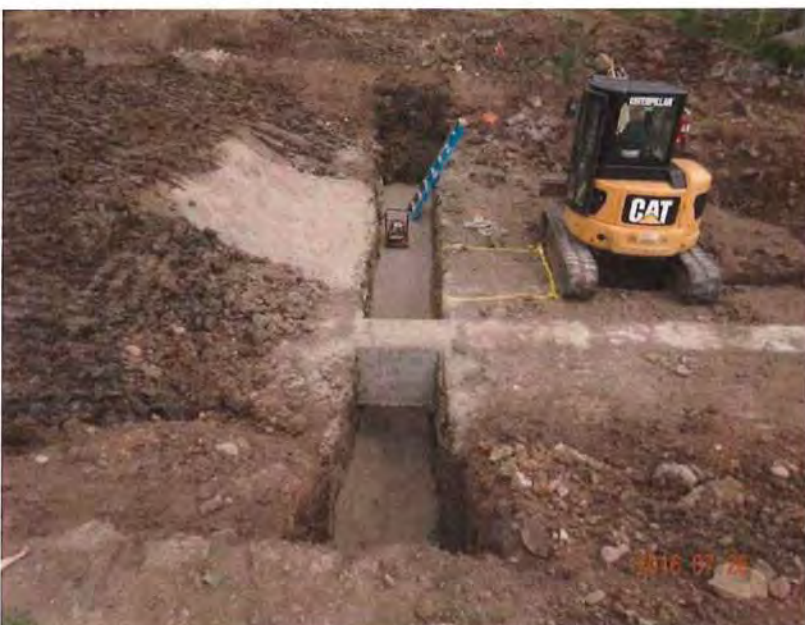
Photo 4 – Filter collar construction (near Station 2+95).
