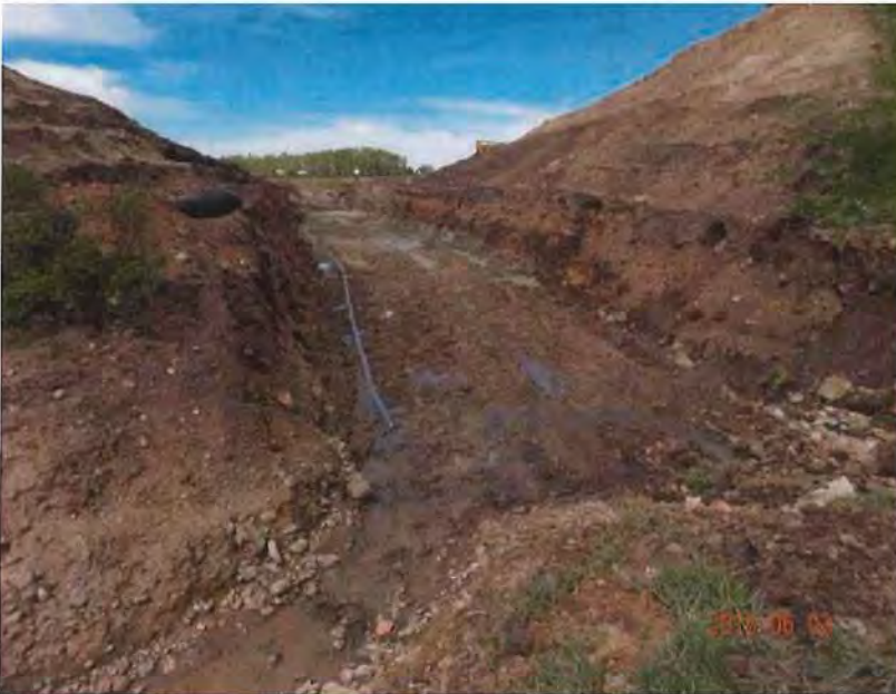
Photo 2 – Condition of the outlet works subgrade, looking upstream.
