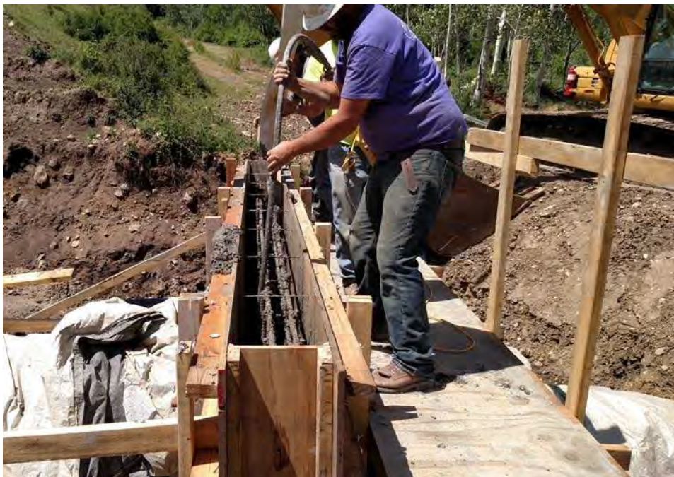
Photograph 30: Placing concrete for the downstream headwall.
