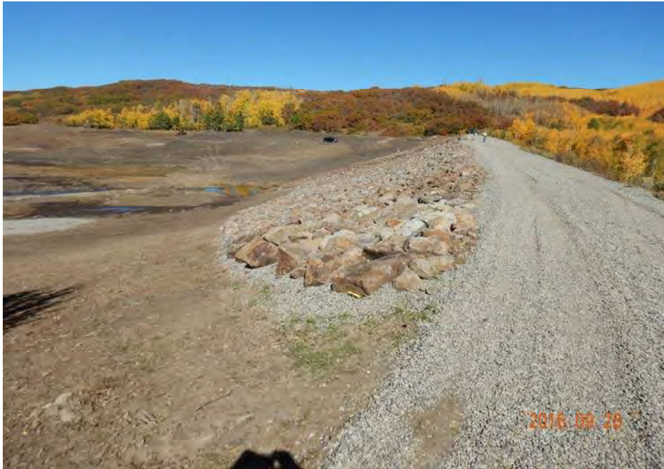
Photograph 47: Riprap on the upstream slope from the right abutment.
