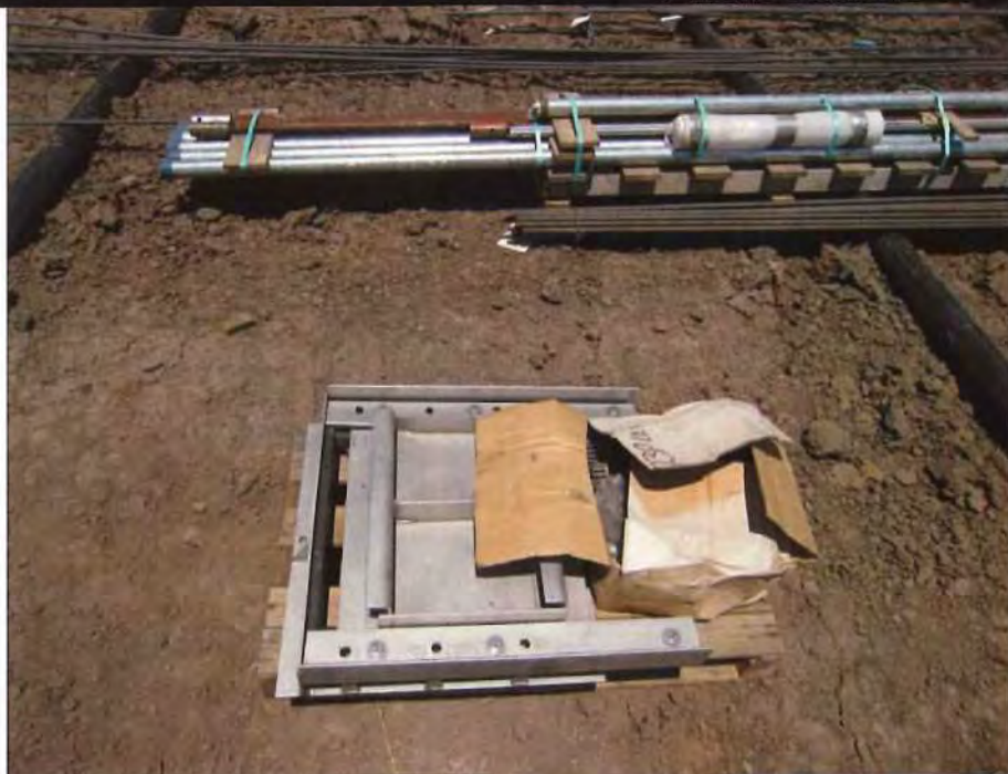
Outlet valve with stem and stem casing in background.
