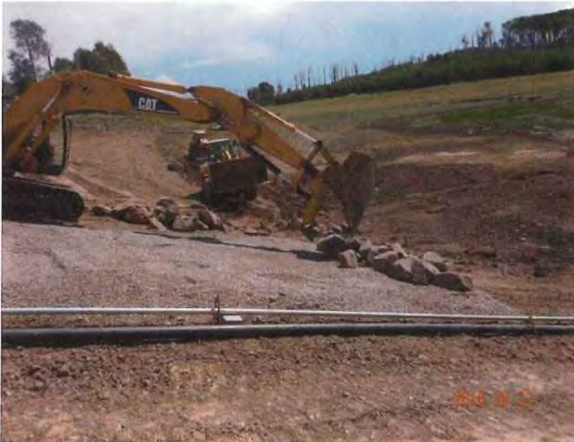
Photo 4 – Placing riprap.
