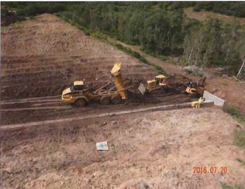
Photo 6 – Placing embankment fill.
