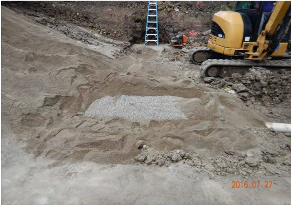
Photograph 19: Filter sand and filter gravel with forms removed.
