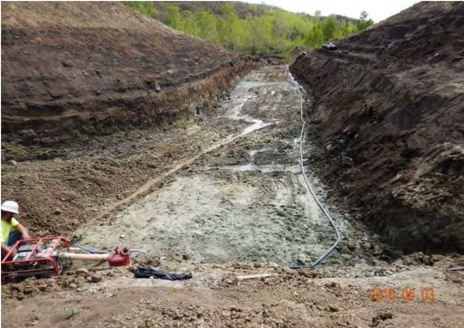
Photograph 5: Condition of excavation at the start of 2016.
