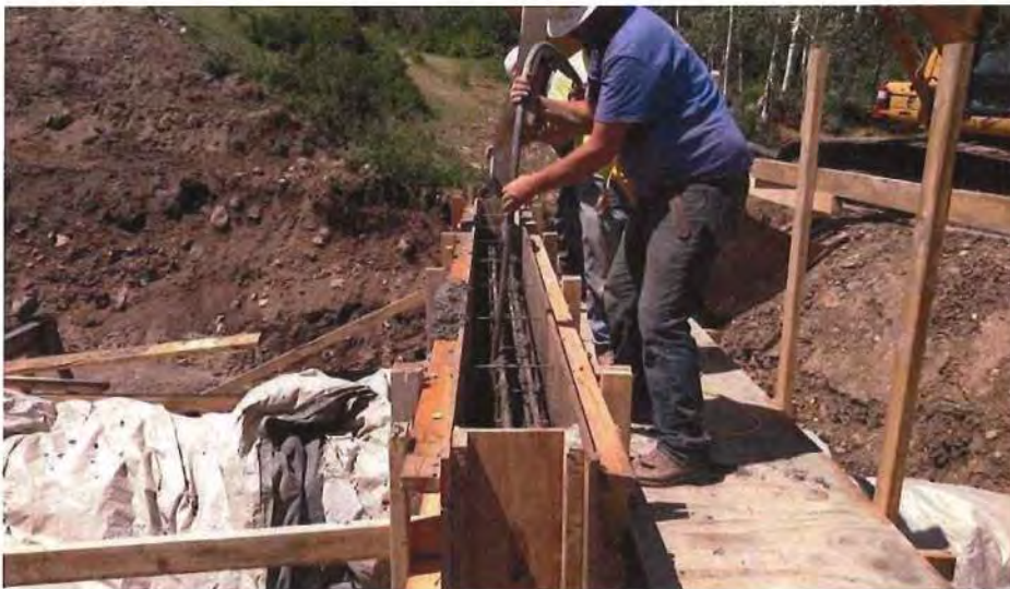
Photo 2 – Placing concrete for the downstream headwall.
