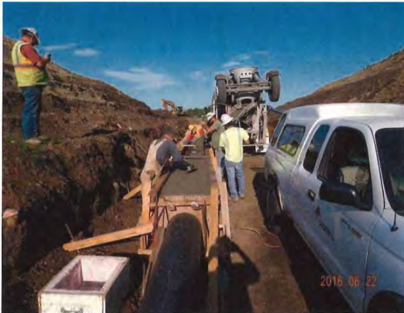
Photo 1 – Placing concrete for the outlet works conduit encasement.
