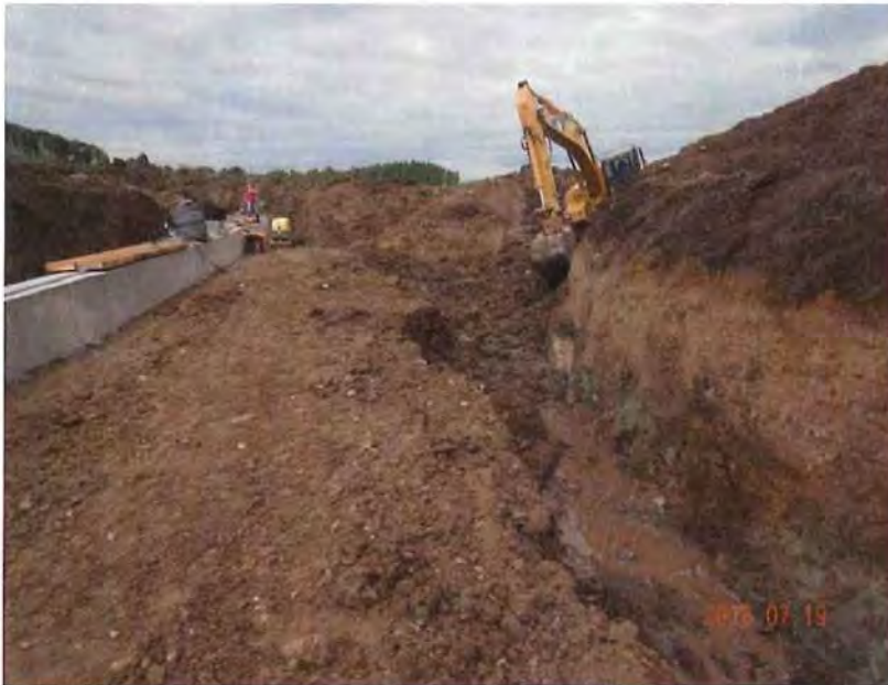
Photo 3 – Beginning excavation of the dewatering trench on the north side of the excavation.
