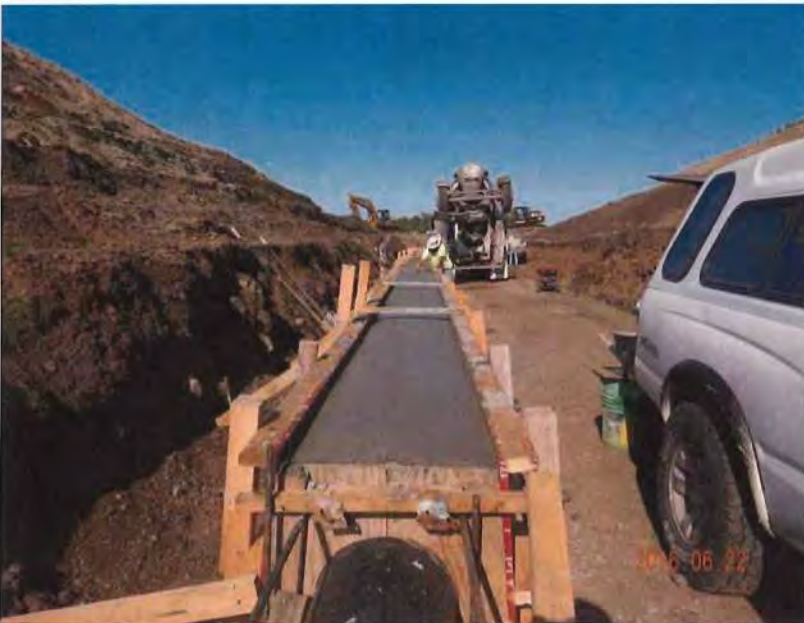
Photo 4 – Placing concrete for the outlet works conduit encasement.
