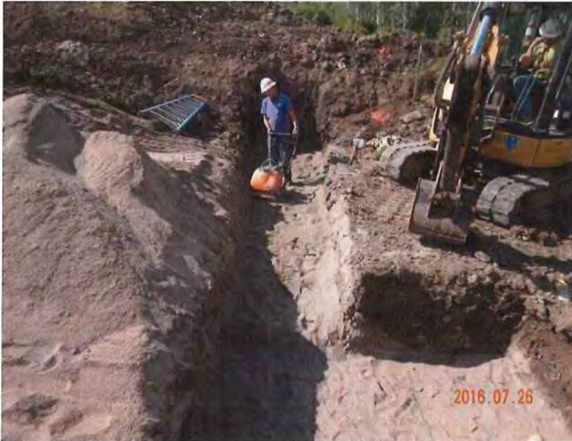
Photo 5 – Compacting filter sand for the filter collar.
