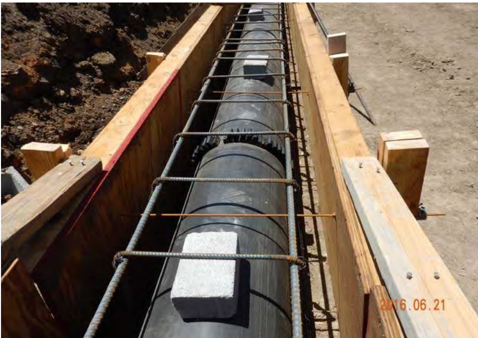
Photograph 26: Outlet conduit prior to concrete placement. Note the exterior band welded to the HDPE conduit.
