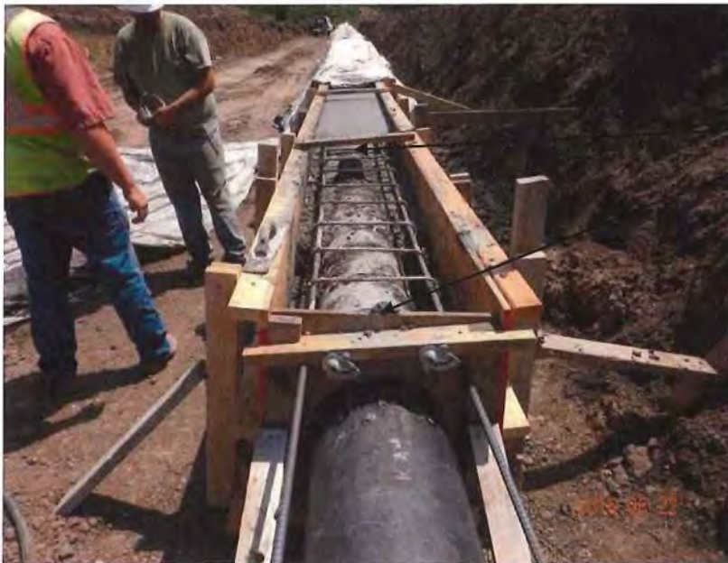
Photo 8 – Placing concrete for the outlet works conduit encasement.
