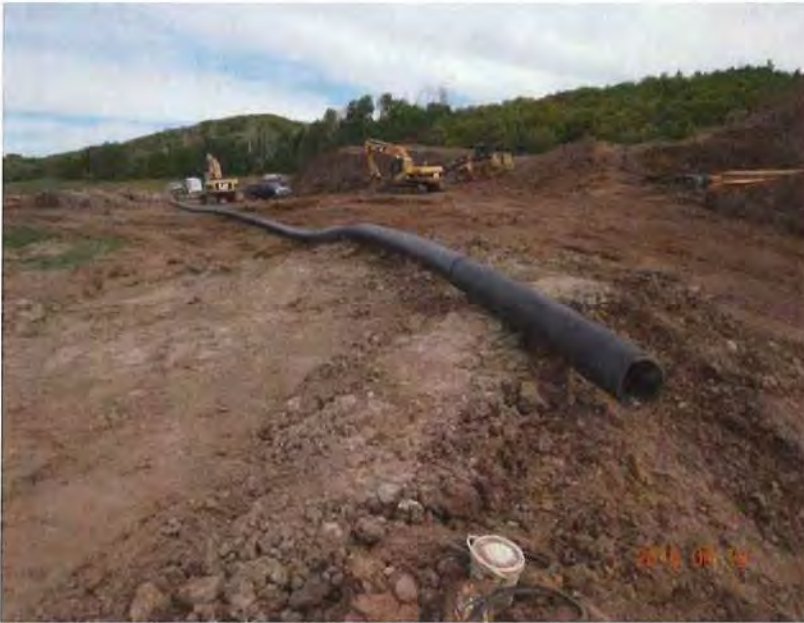
Photo 3 – Outlet works conduit (HDPE pipe) prior to placement in the dam.
