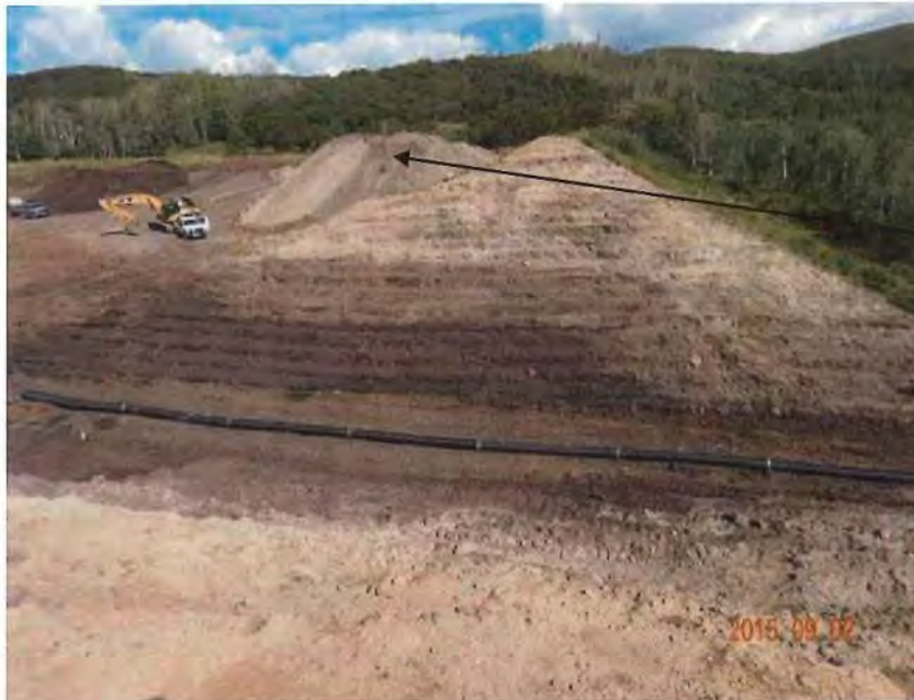
Photo 1 – Excavation through existing embankment.
