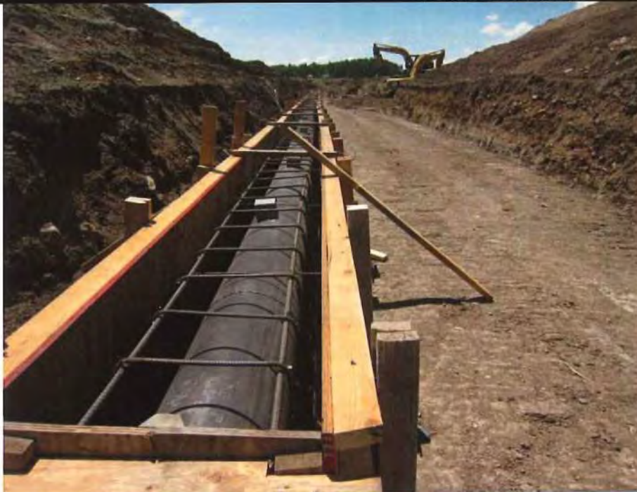
HDPE outlet pipe placed on prepared foundation with encasement reinforcement and concrete forms.
