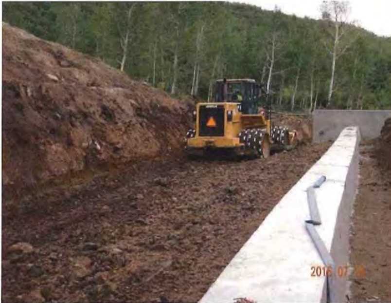
Photo 5 – Compacting embankment fill.
