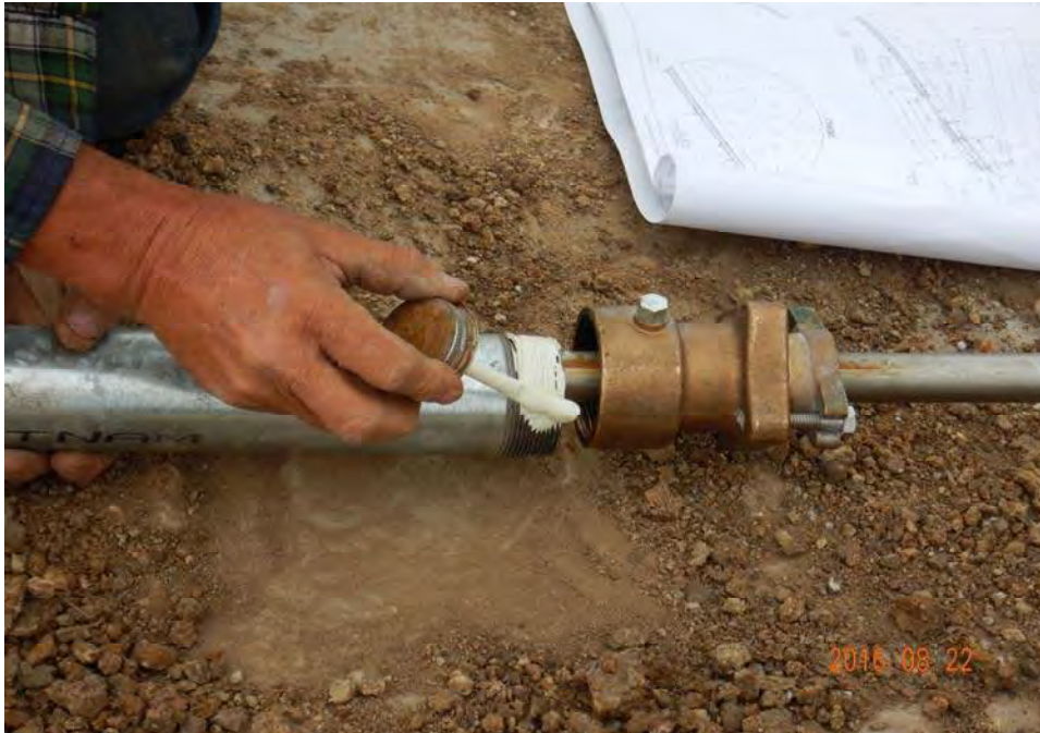
Photograph 35: Placing pipe joint compound to seal the gate stem cover at the inlet structure.
