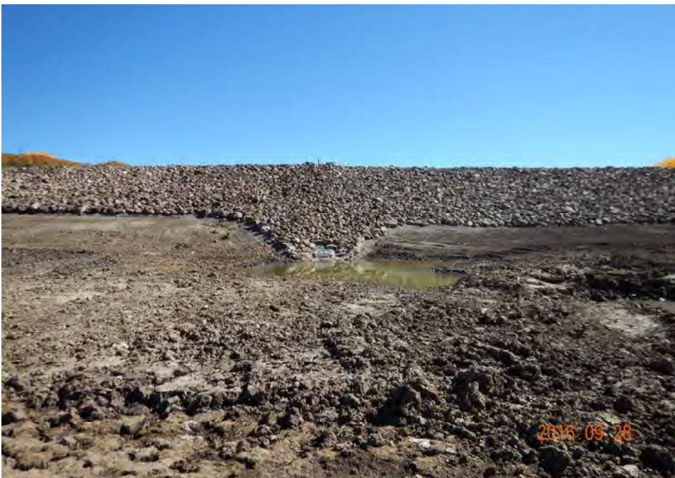
Photograph 50: Upstream slope. Note riprap around the inlet structure.
