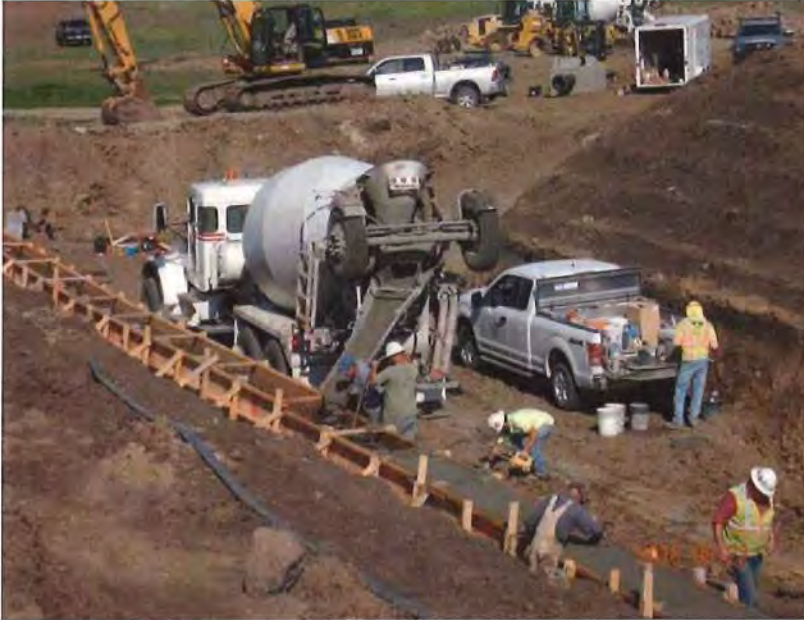
Photo 7 - Placing concrete for the outlet works conduit encasement.
