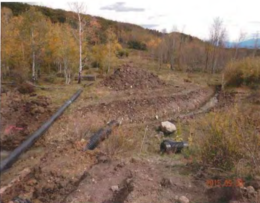
Photo 2 – Channel excavation downstream of dam (to Jay Creek).
