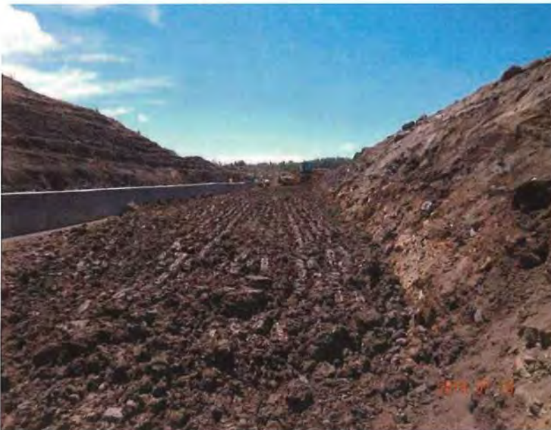
Photo 6 – Completed embankment fill to about Elevation 8740. Note slope of existing embankment (right side of photograph).
