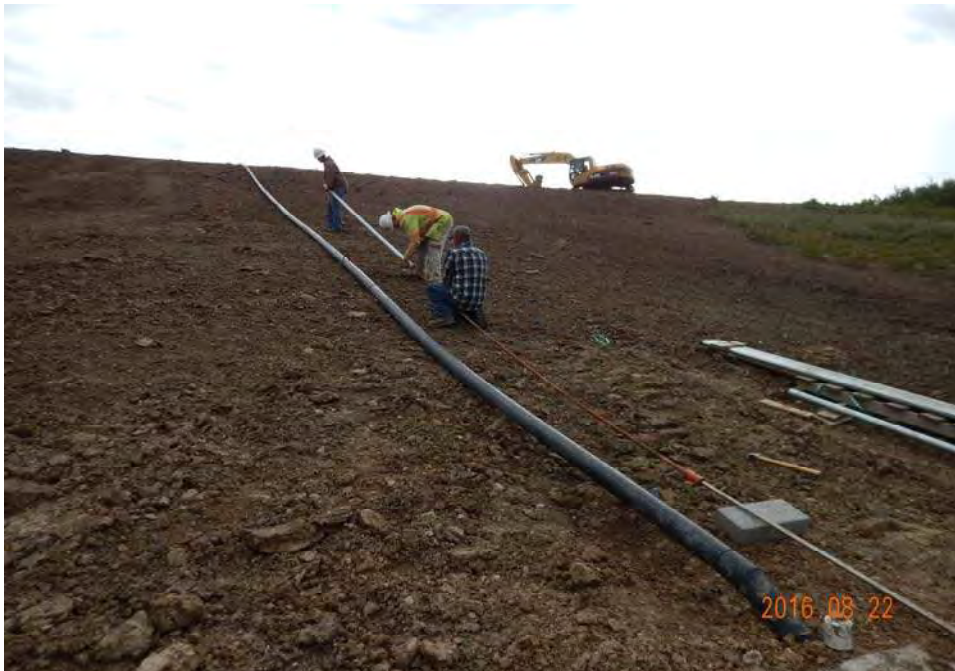
Photograph 34: Placing gate stem and stem cover on the upstream slope.
