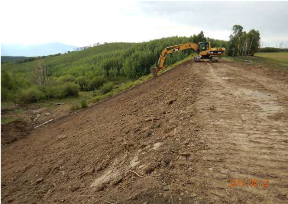
Photograph 13: Placing topsoil on the downstream slope.
