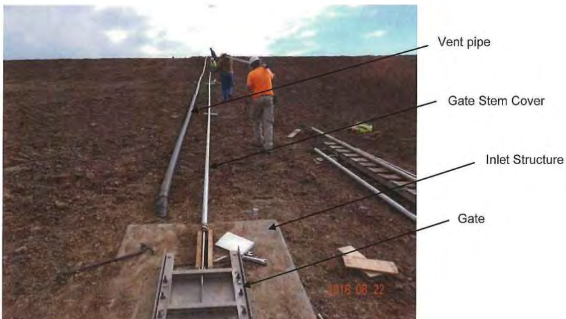
Photo 4 – Vent pipe and gate stem/stem cover on the upstream slope.
