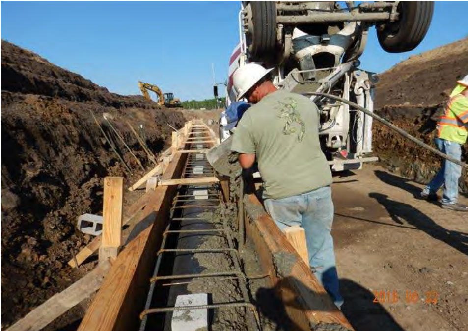
Photograph 27: Placing encasement concrete. Concrete placed and vibrated on one side of the pipe until flow under the conduit is observed.
