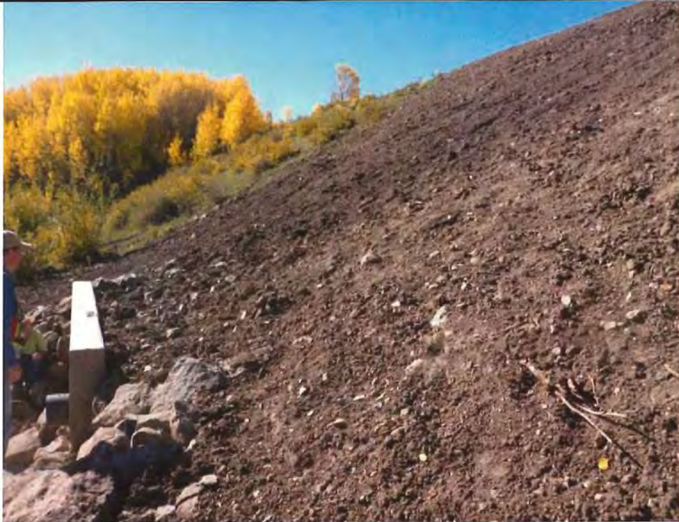
Downstream slope of dam in repaired breach area.
