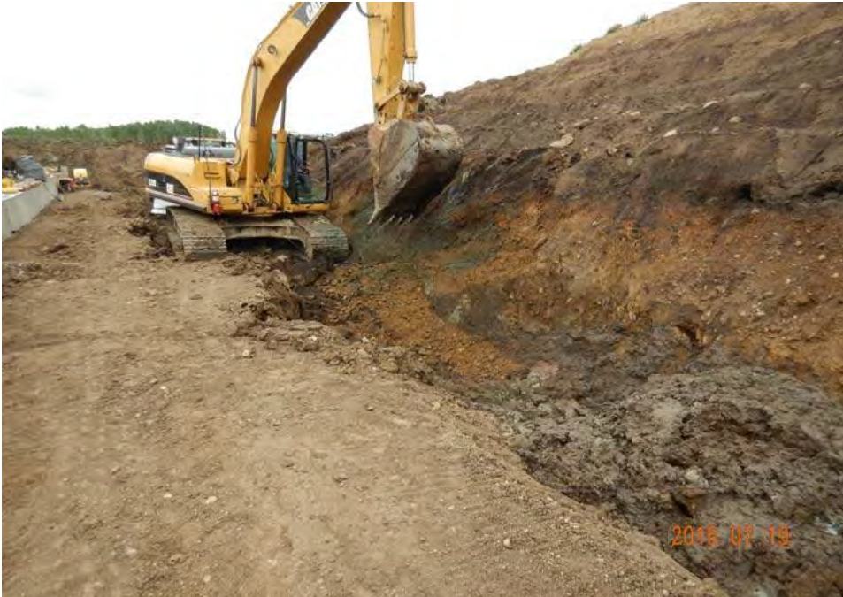
Photograph 7: Excavating the dewatering trench on the left side of the working platform prior to placing common fill for the embankment.
