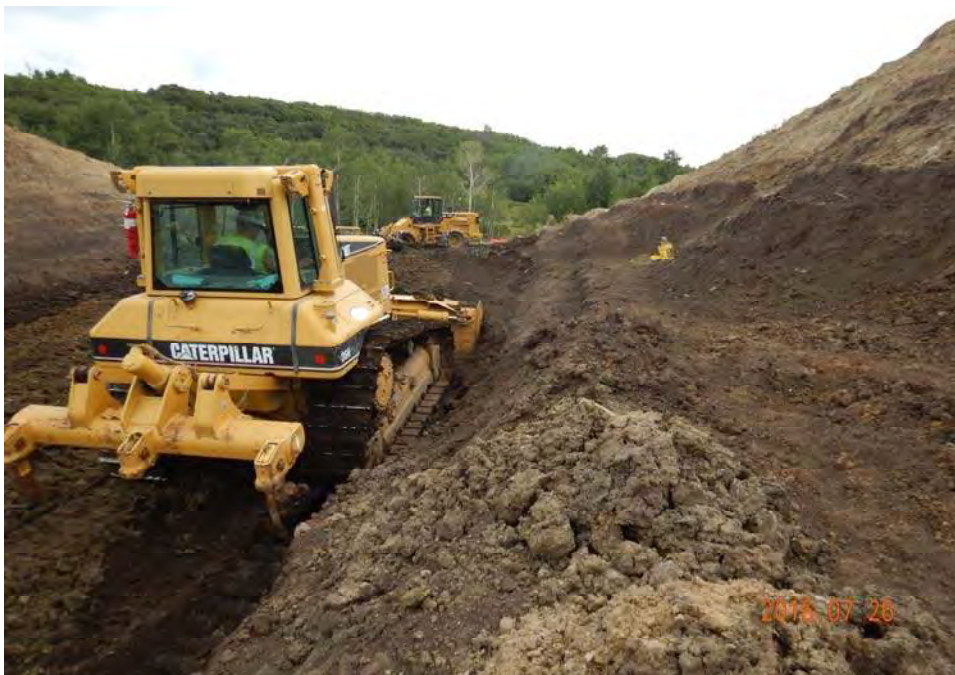
Photograph 12: Cutting the existing slope back to fresh material and eliminating steep slopes.
