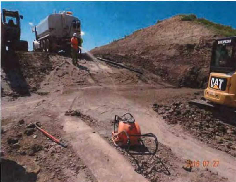
Photo 6 – Spraying water on the partially completed filter collar.
