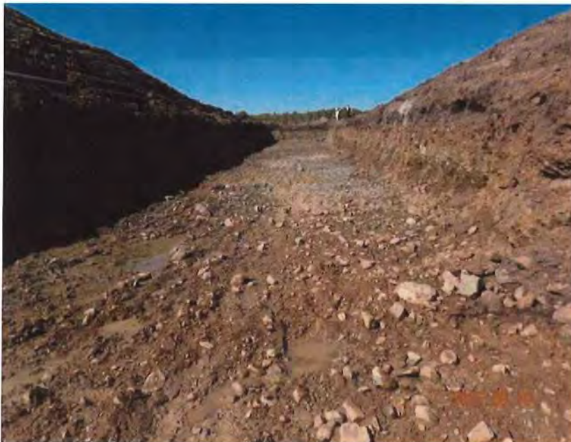
Photo 2 – Bottom of the excavation looking upstream.
