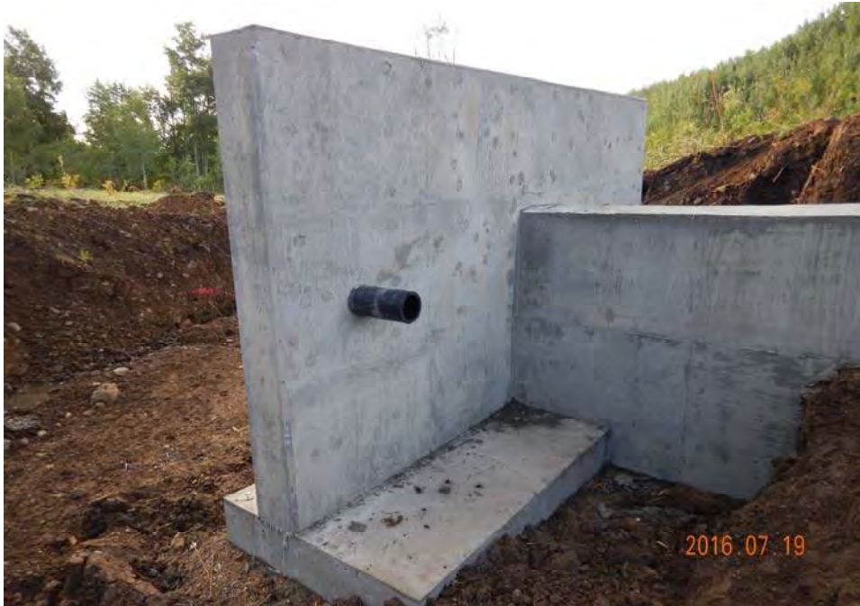
Photograph 31: Downstream headwall, upstream side.
