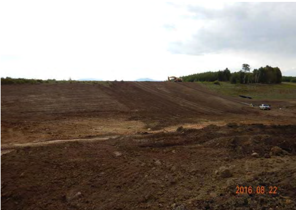
Photograph 14: Finished embankment, upstream slope.
