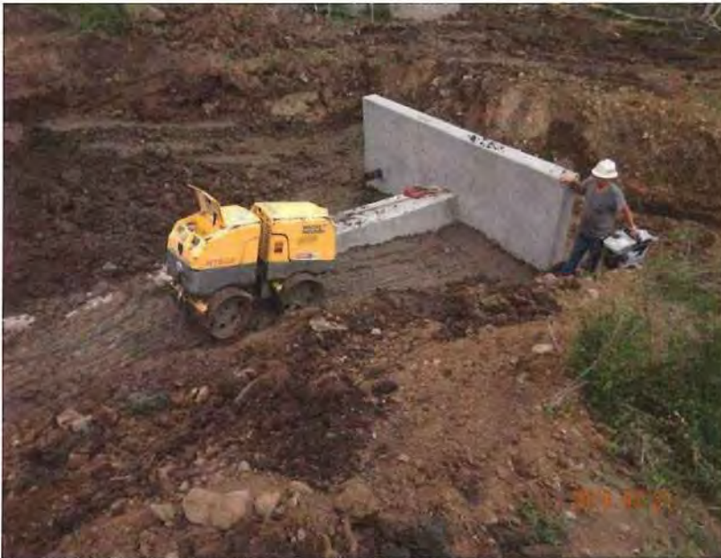
Photo 3 – Compacting fill on south side of headwall.
