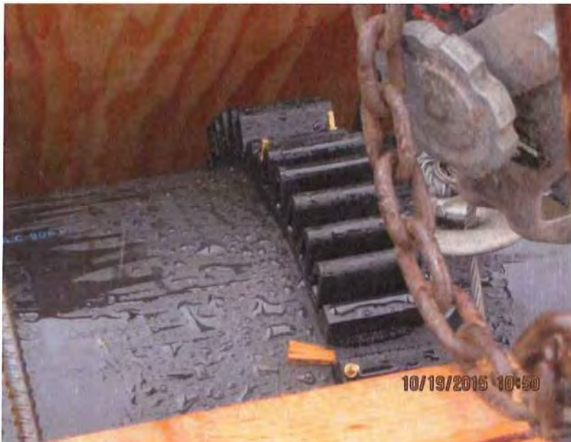
Photo 4 – Exterior band attached to HDPE pipe.
