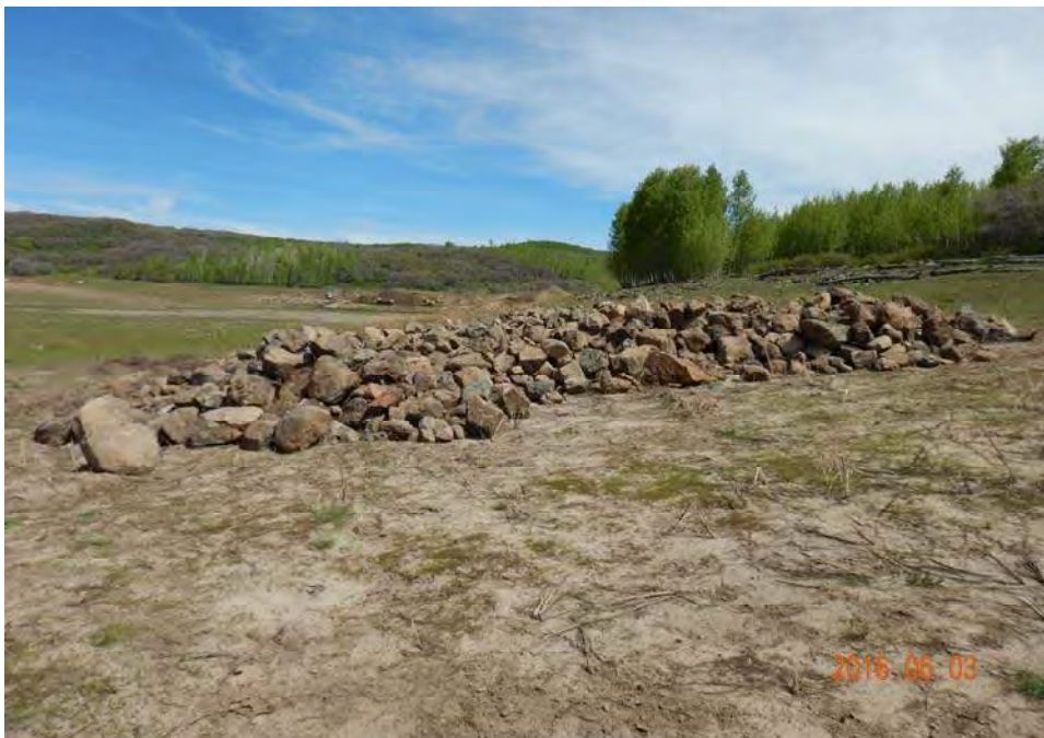
Photograph 44: Riprap stockpile from on-site materials.
