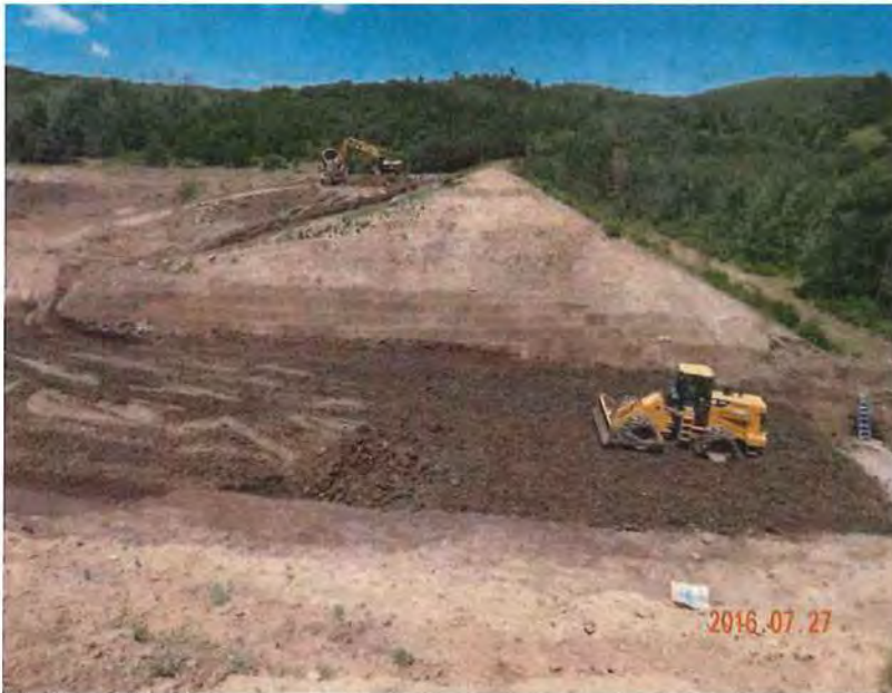
Photo 1 – Placing common fill for the embankment.
