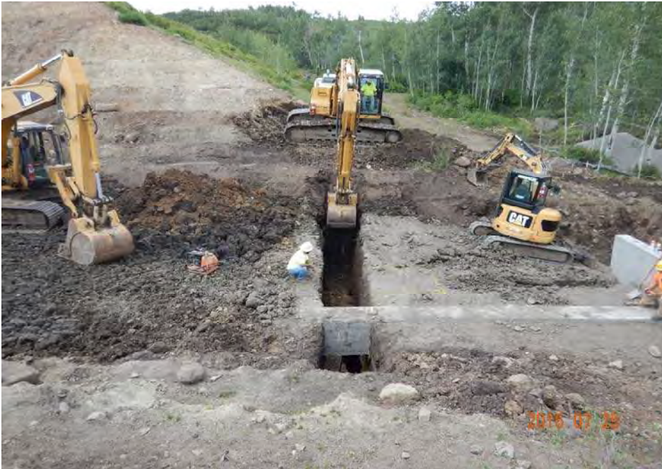
Photograph 15: Excavating the trench for the filter collar.
