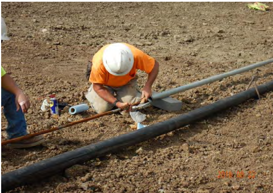
Photograph 36: Connecting gate stem segments.
