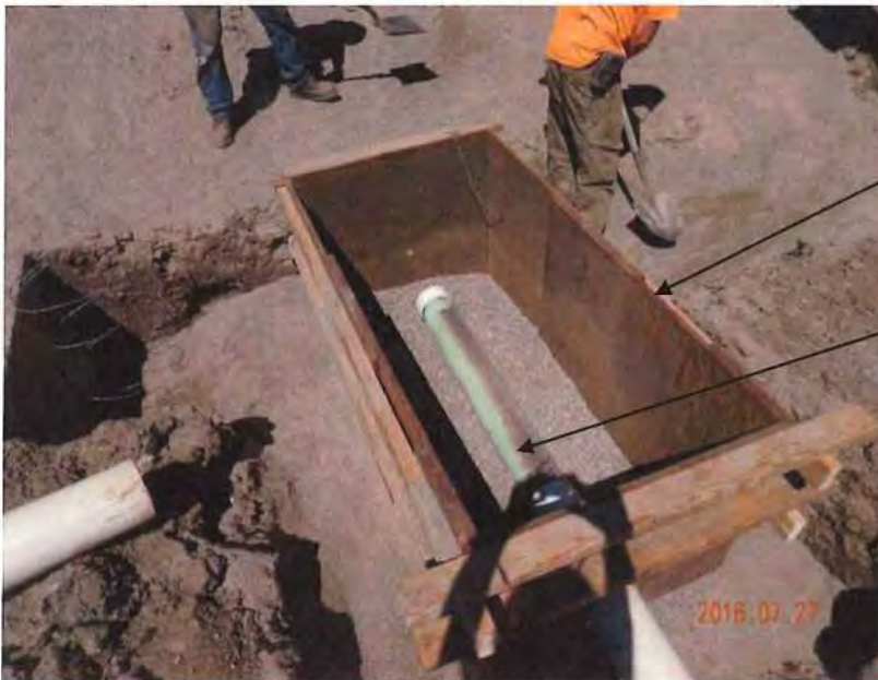
Photo 2 – Placing filter collar near Station 2+95.
