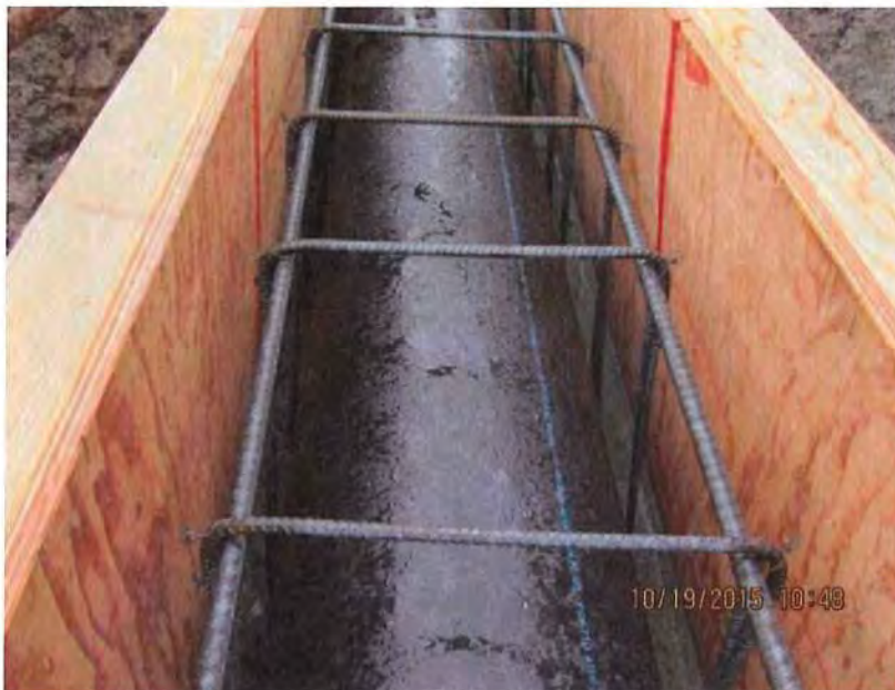
Photo 3 - Reinforcing steel for the outlet works encasement.
