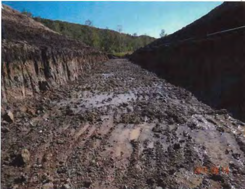
Photo 1 – Bottom of excavation looking downstream. Note the standing water.
