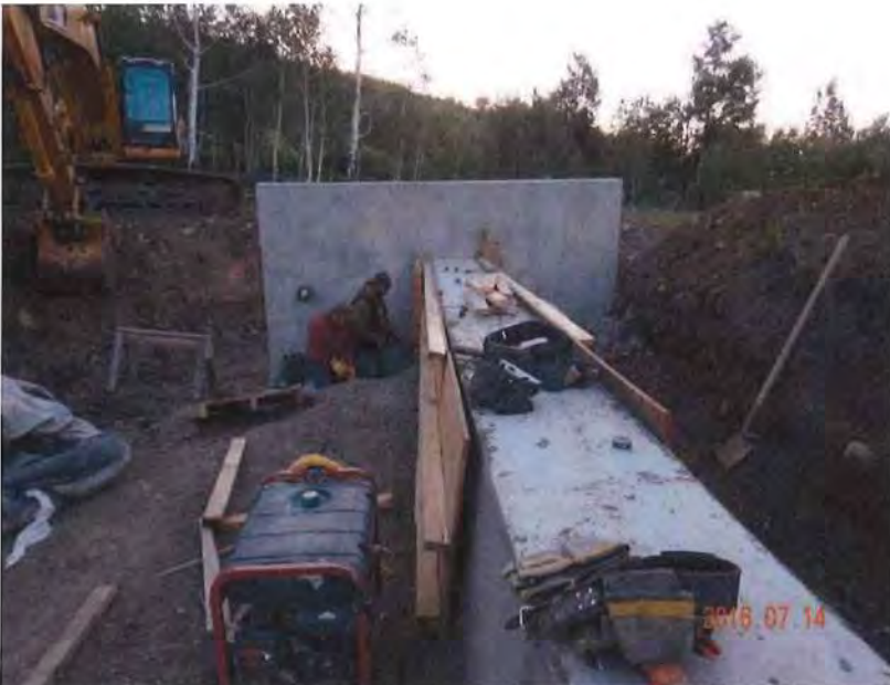
Photo 2 – Removing formwork from the downstream conduit encasement.
