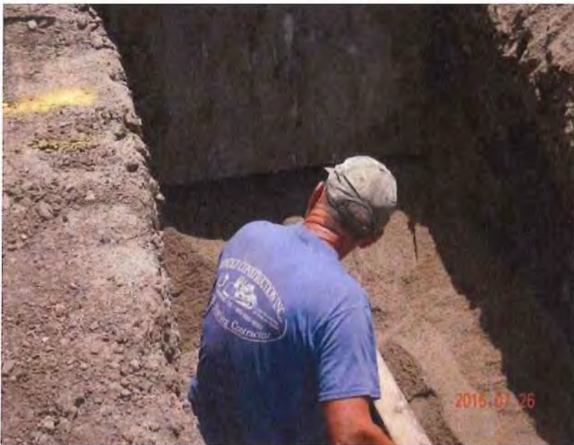
Photo 6 – Compacting filter sand beneath the conduit encasement.
