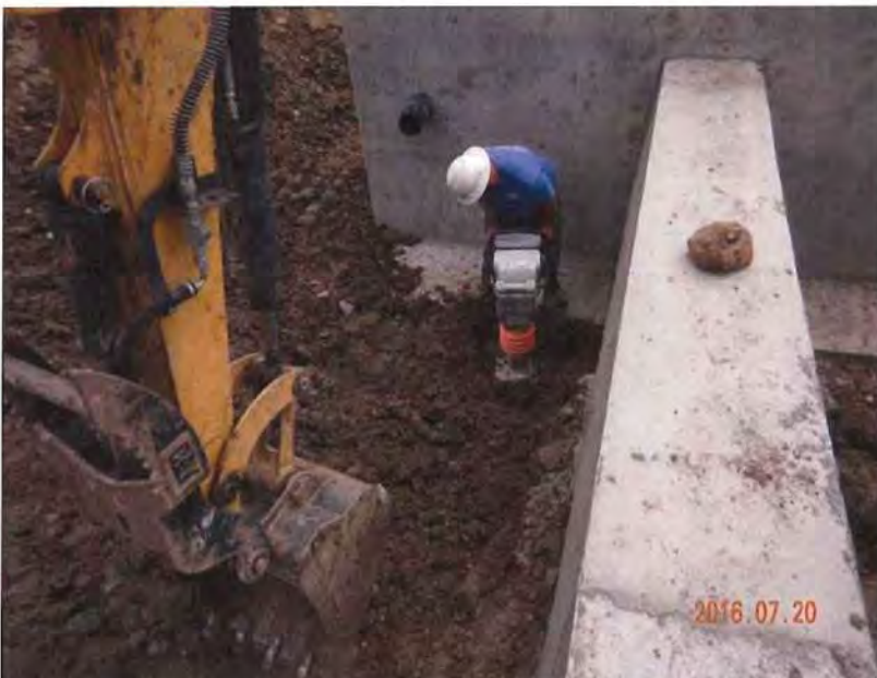
Photo 4 – Compacting backfill on the north side of the conduit encasement using hand operated equipment.
