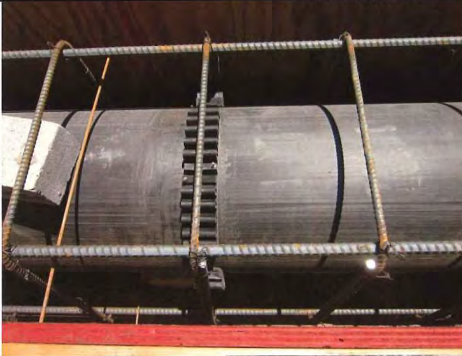
Close-up of outlet pipe, rebar cage, concrete forms, and exterior band to prevent lateral displacement of pipe.
