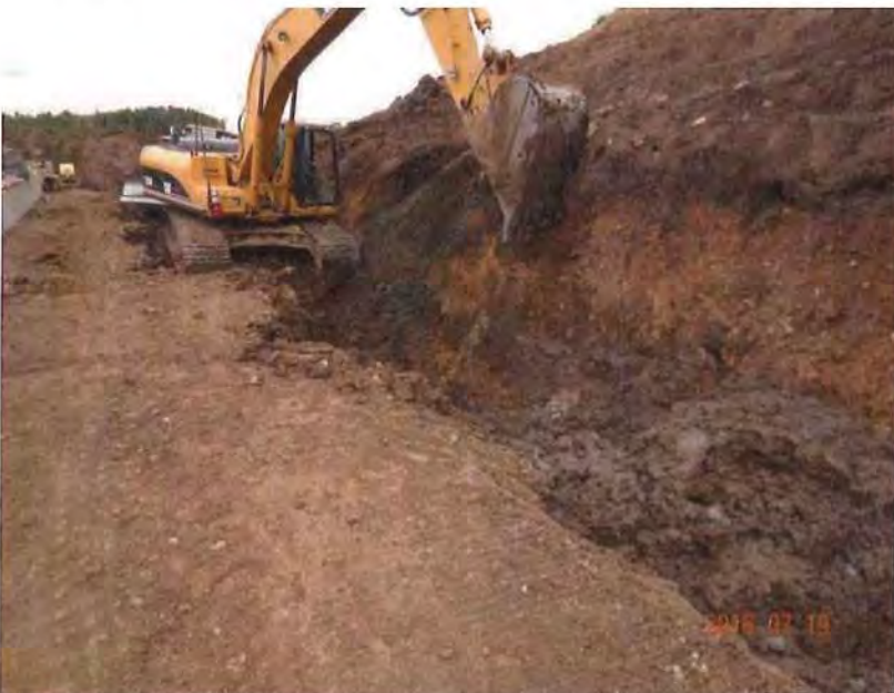
Photo 4 – Excavation of the dewatering trench on the north side of the excavation. Note width of excavation and excavation of the existing embankment to create a slope.
