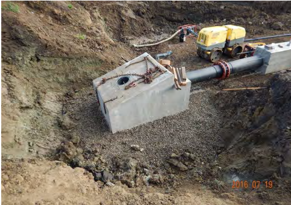
Photograph 33: Precast inlet structure in-place. Note the flange connection downstream of the structure.
