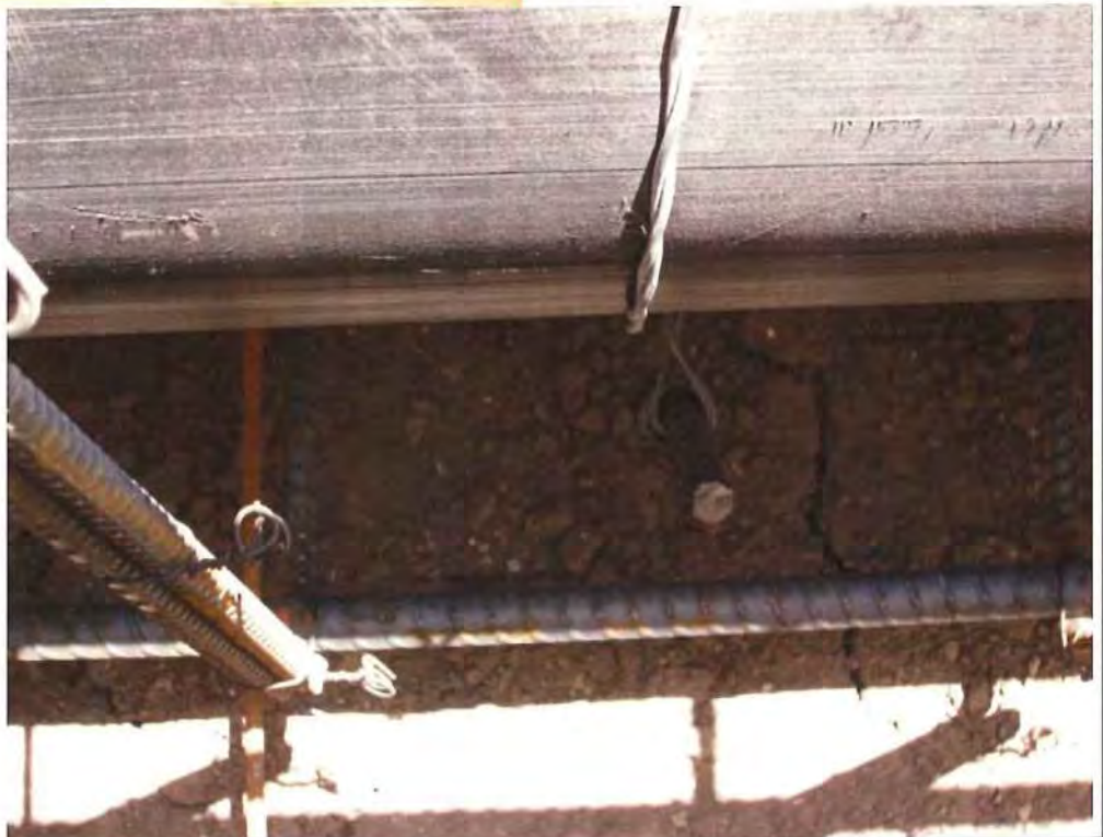
Close-up of wire tie and rebar to prevent floatation of the outlet pipe during concrete placement.
