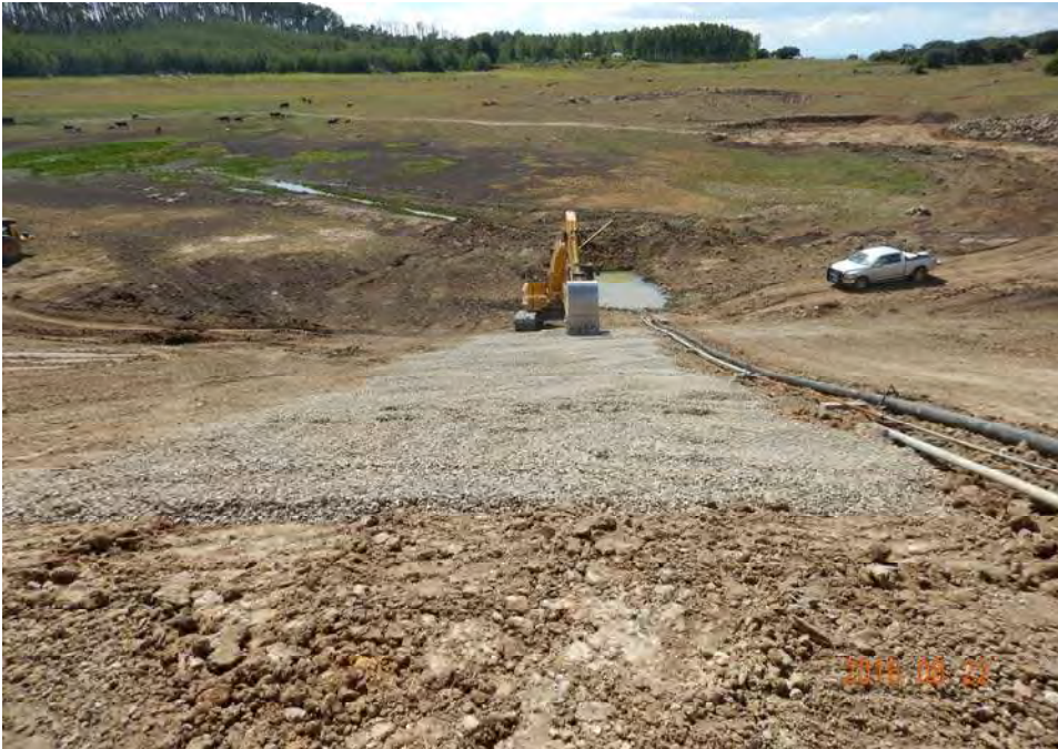
Photograph 45: Placing riprap bedding on the upstream slope.
