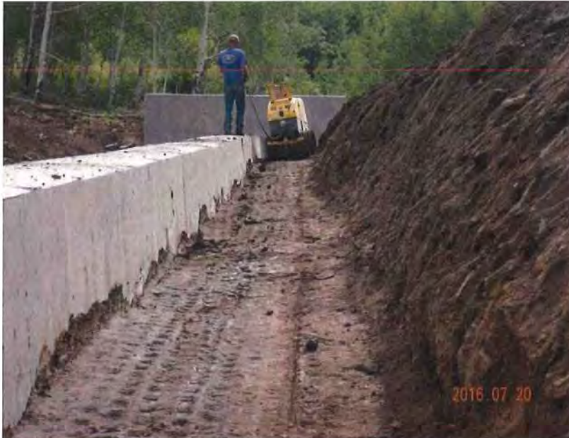
Photo 3 – Compacting fill on the south side of the conduit encasement.
