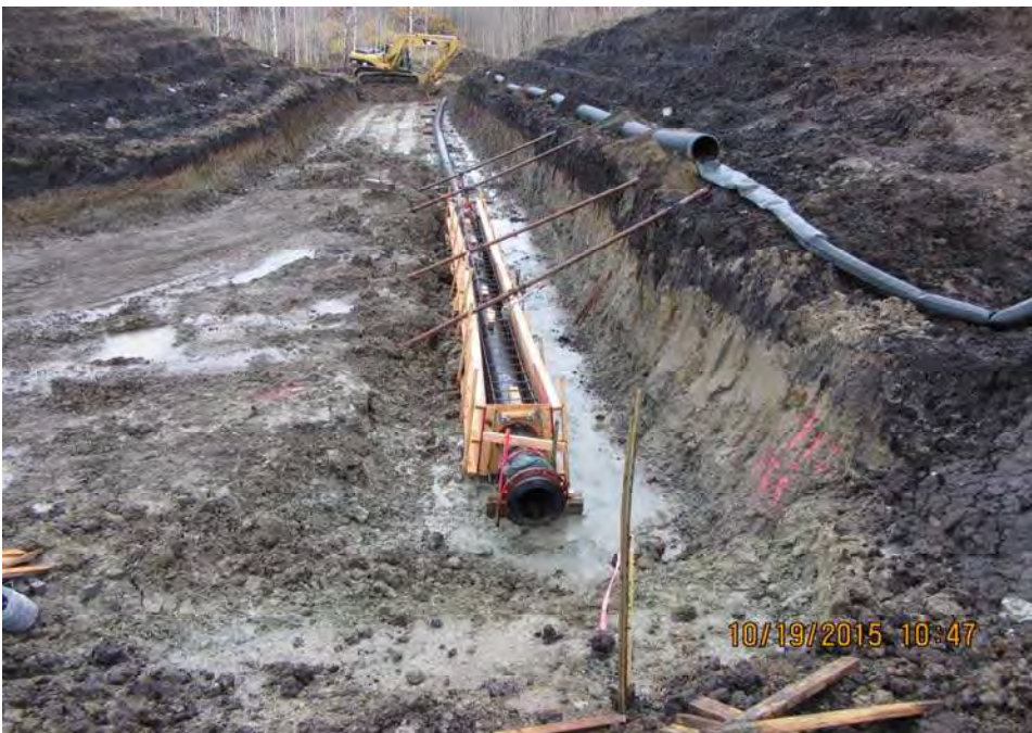
Photograph 4: Condition of excavation at the end of 2015.
