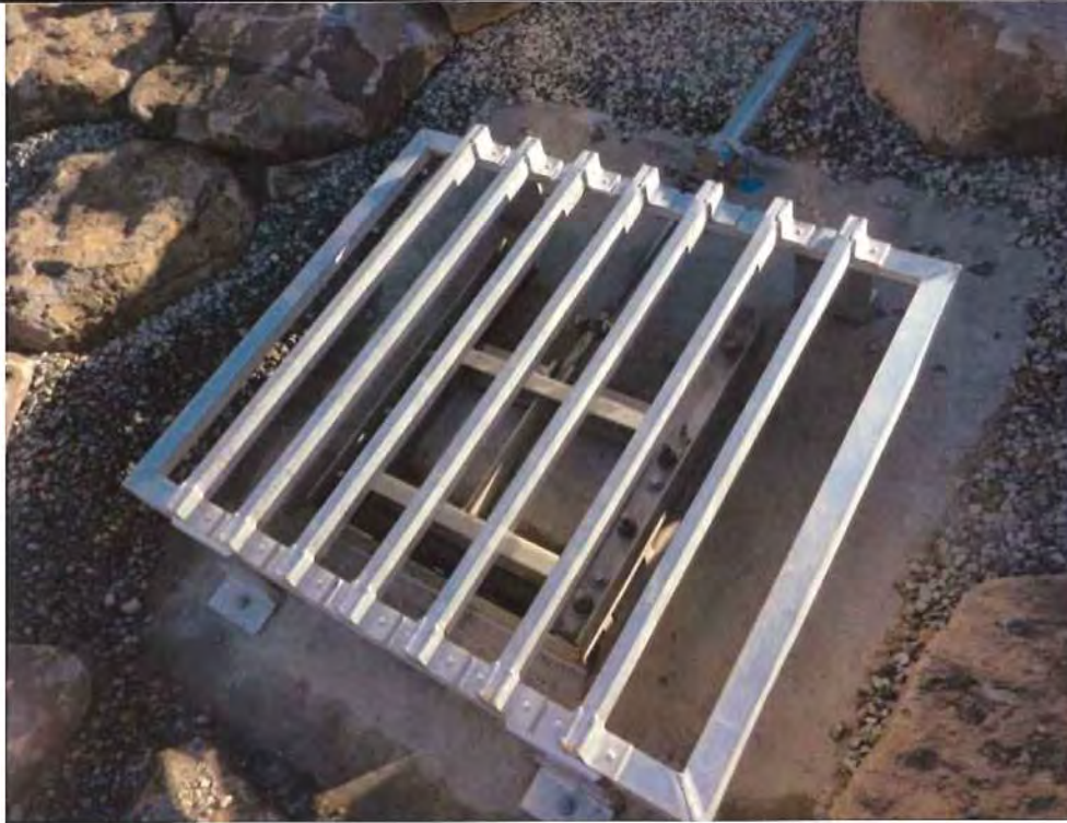
Aluminum trash rack on outlet gate.
