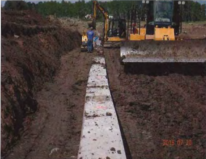
Photo 5 – Completed backfill on both sides of the conduit encasement.
