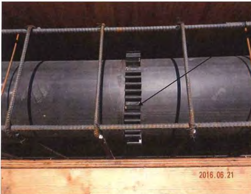
Photo 2 – Outlet works conduit (HDPE pipe) and reinforcing steel.
