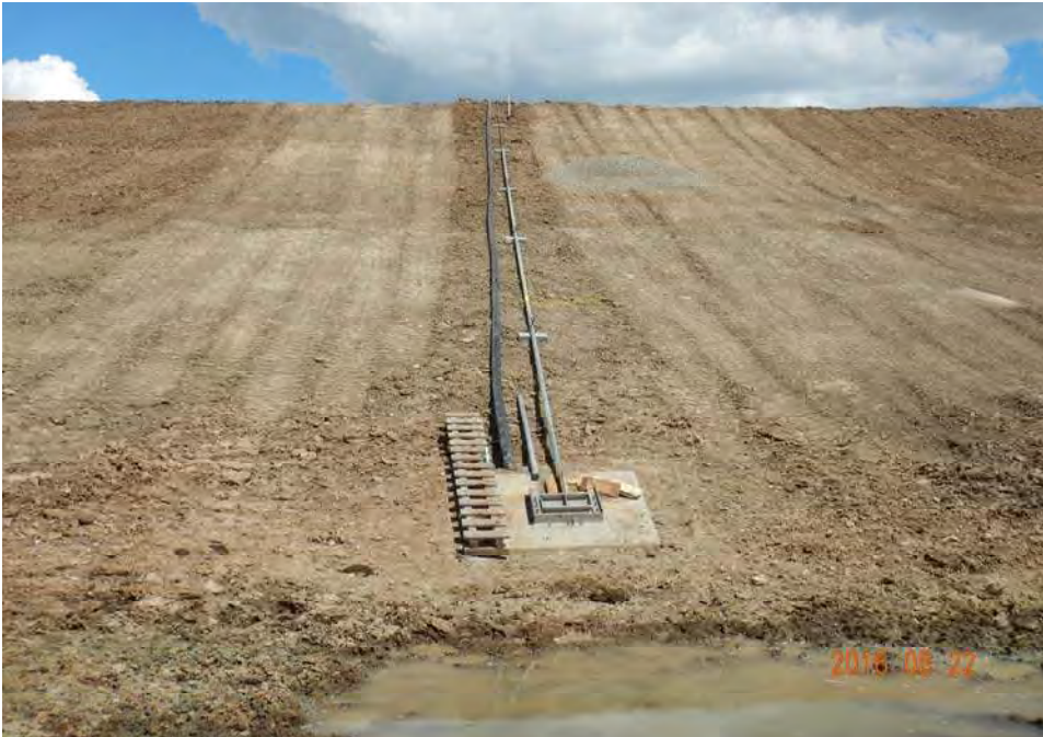
Photograph 37: Gate stem cover and vent pipe on the upstream slope.
