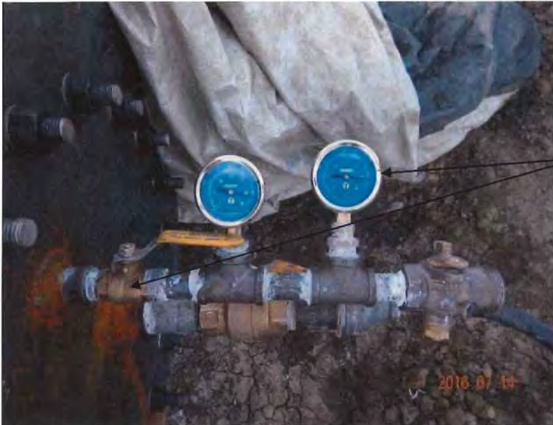
Photo 1 – Gauges and valves used for pressure testing the outlet works conduit.
