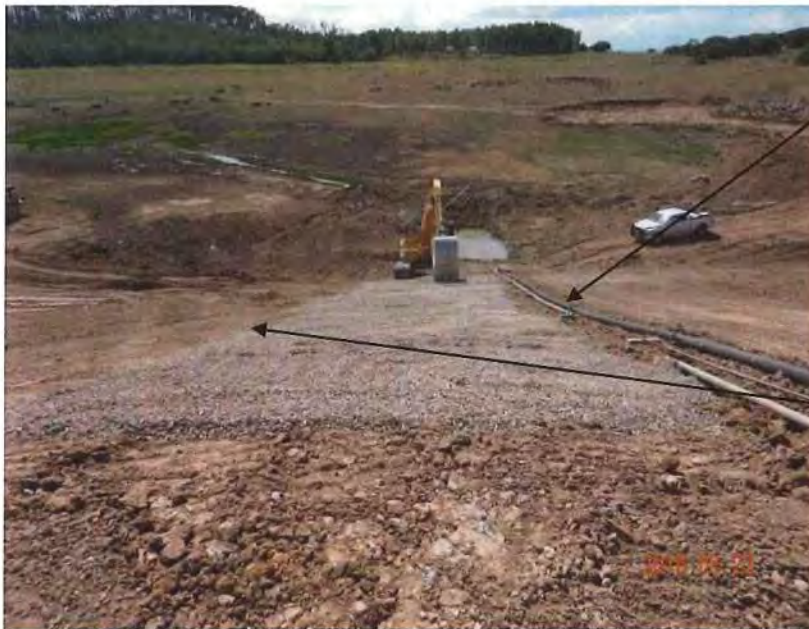
Photo 3 – Placing riprap bedding.
