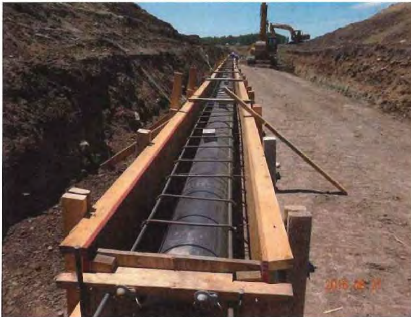
Photo 1 – Outlet works conduit encasement formwork, looking upstream.
