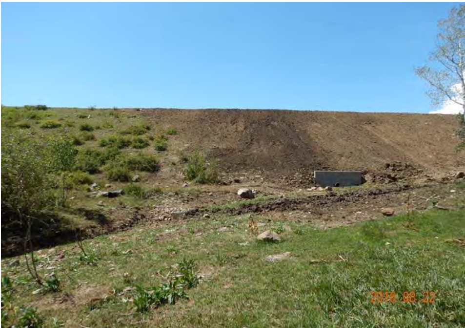
Photograph 22: Completed downstream slope.
