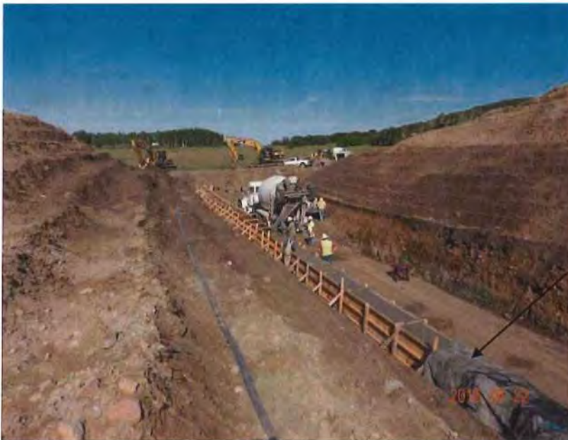
Photo 6 – Placing concrete for the outlet works conduit encasement.
