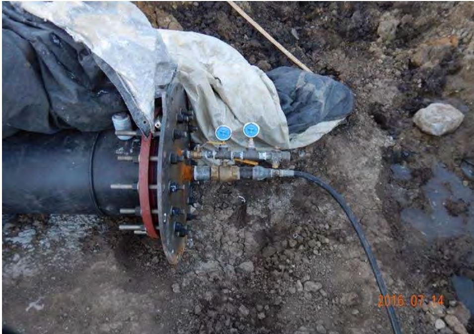
Photograph 29: Conduit pressure test apparatus (valves and pressure gauges).
