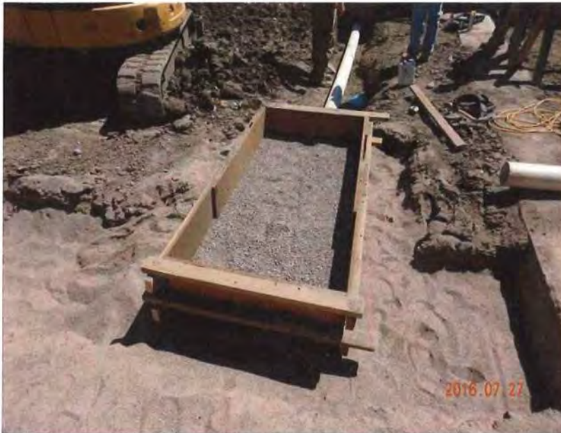
Photo 3 – Forms used to contain filter gravel.
