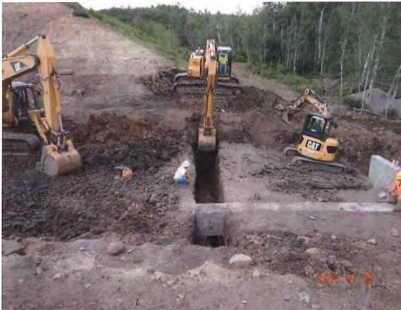
Photo 1 – Excavating for the filter collar near Station 2+95.
