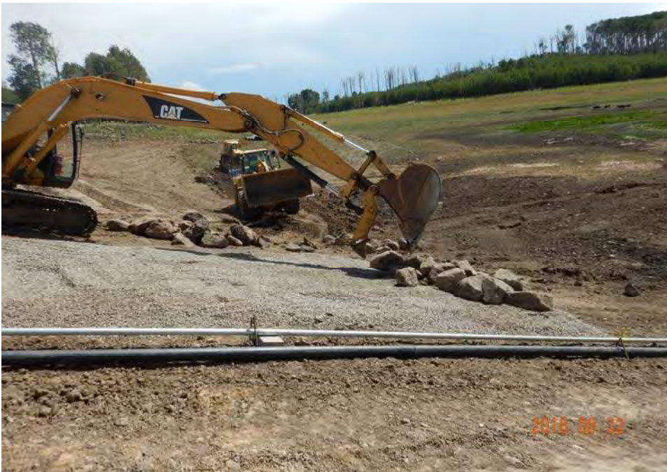
Photograph 46: Placing riprap on the upstream slope.
