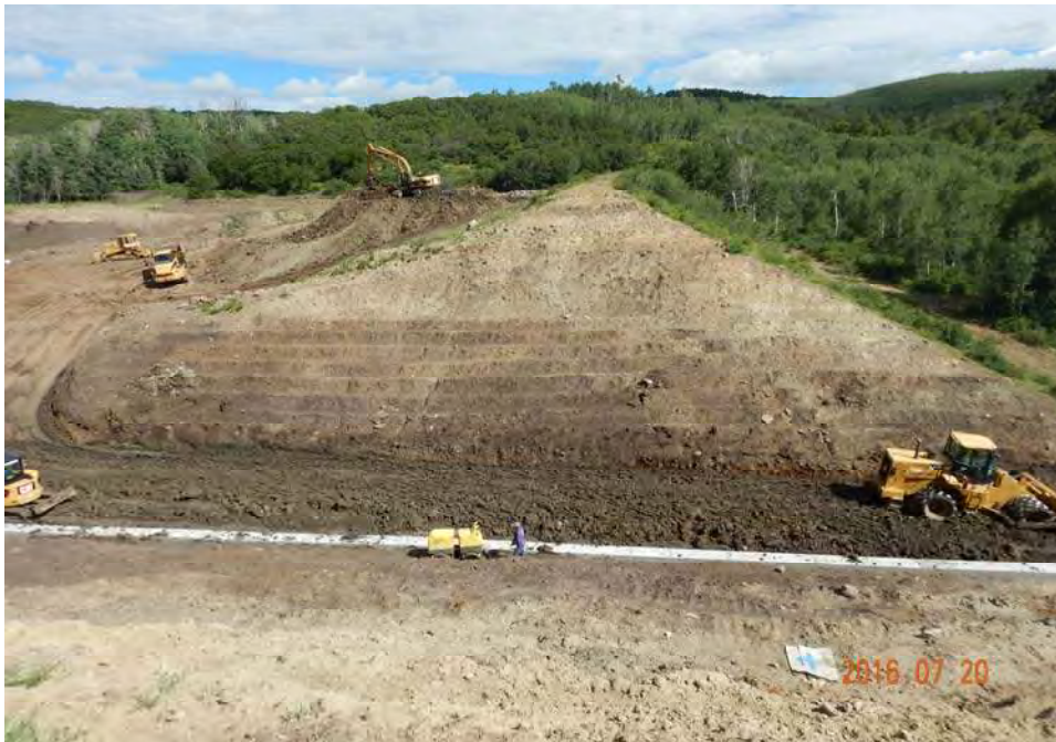
Photograph 10: Placing common fill for the embankment.
