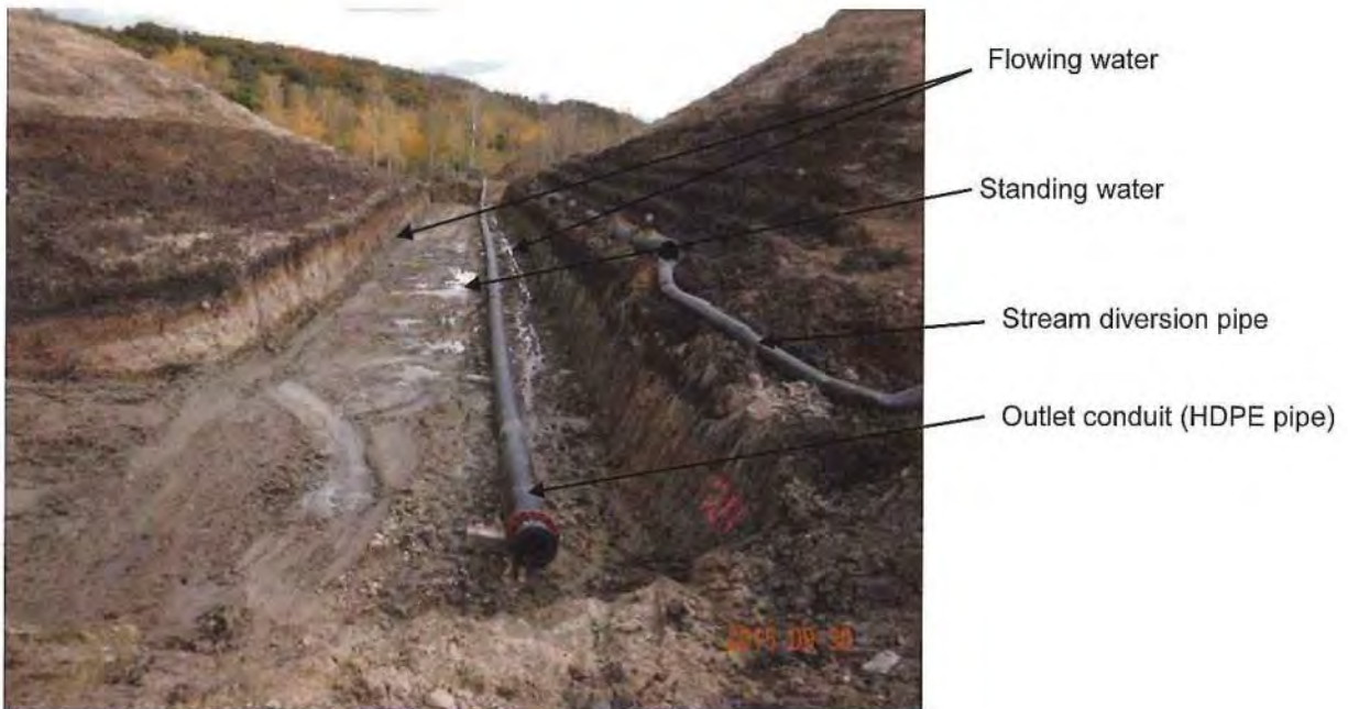
Photo 1 – Outlet works excavation.
