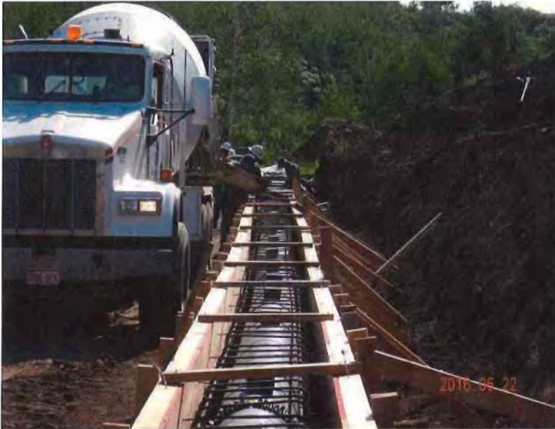
Photo 5 - Placing concrete for the outlet works conduit encasement.
