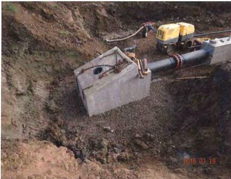
Photo 1 – Outlet works inlet structure.
