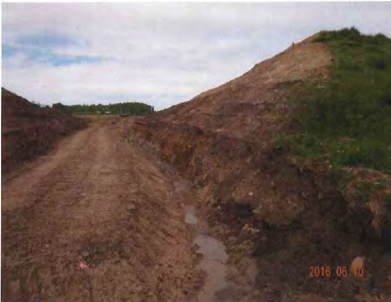
Photo 2 – Working platform looking upstream.
