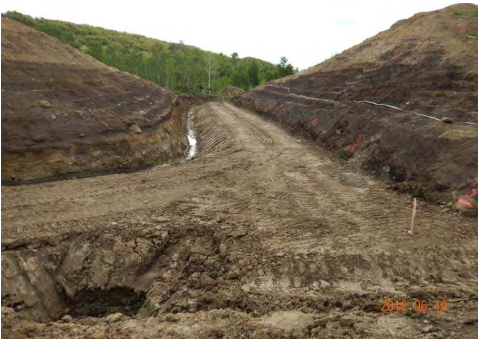
Photograph 6: Working platform constructed in 2016.
