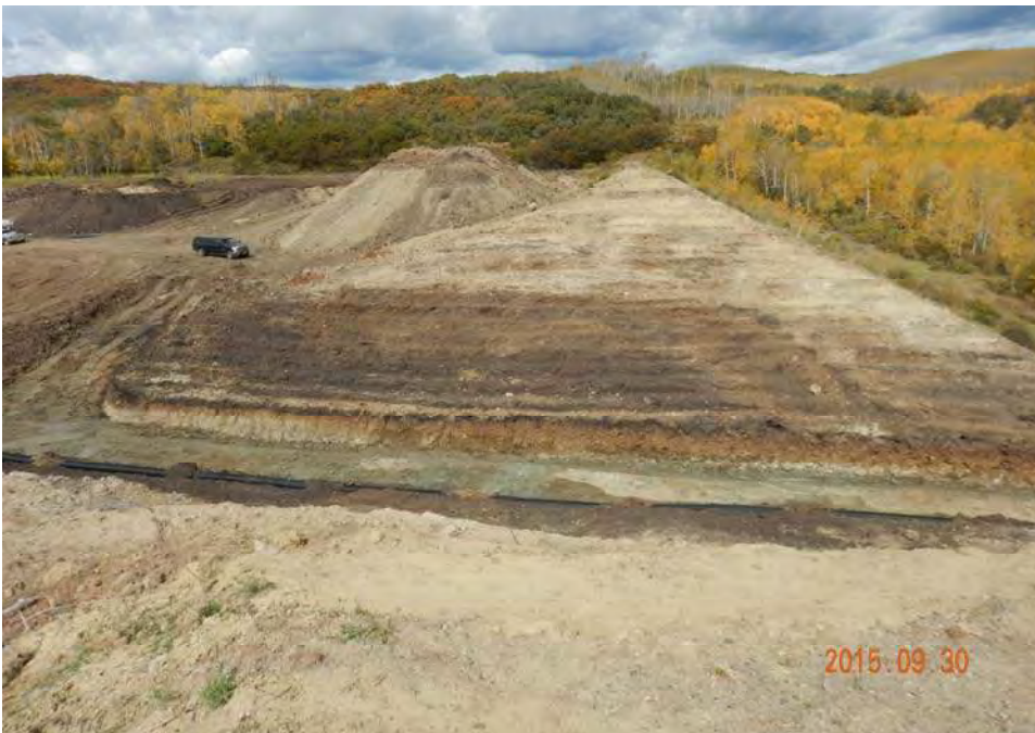
Photograph 2: Completed excavation above the outlet works.
