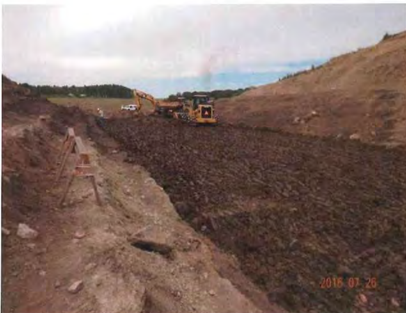
Photo 2 – Placing embankment fill, looking upstream.
