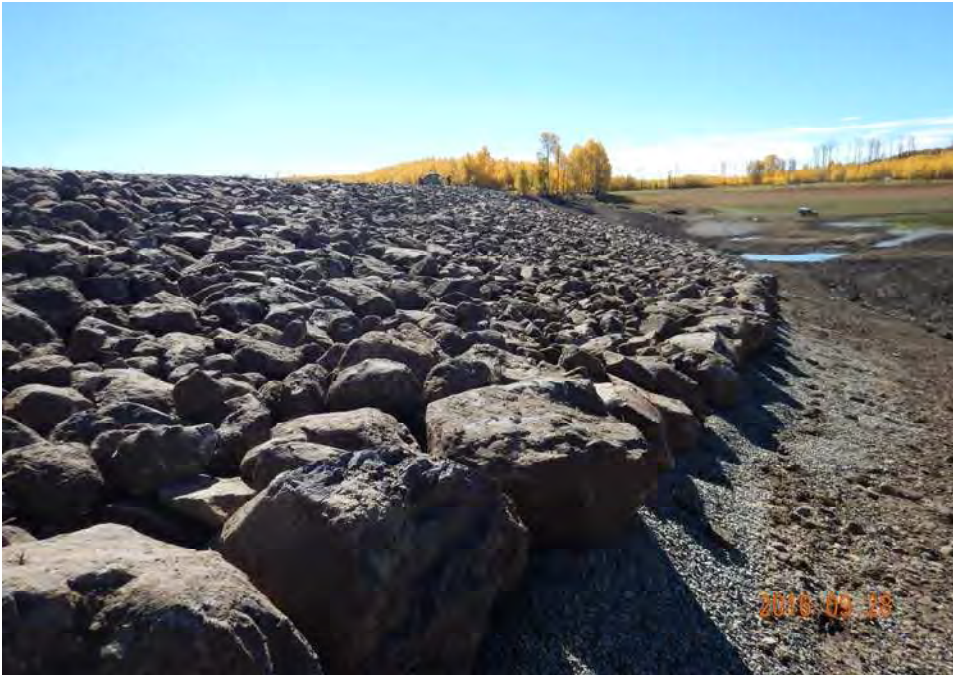
Photograph 49: Toe of riprap on the upstream slope. Note large rocks on the toe.
