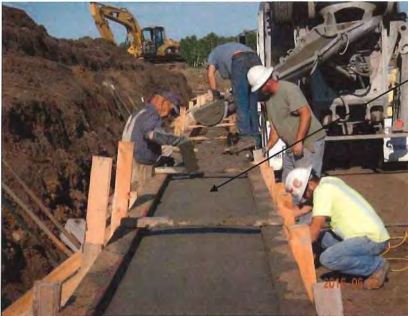
Photo 3 - Placing concrete for the outlet works conduit encasement.
