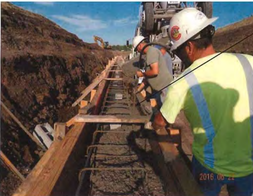
Photo 2 – Placing concrete for the outlet works conduit encasement.
