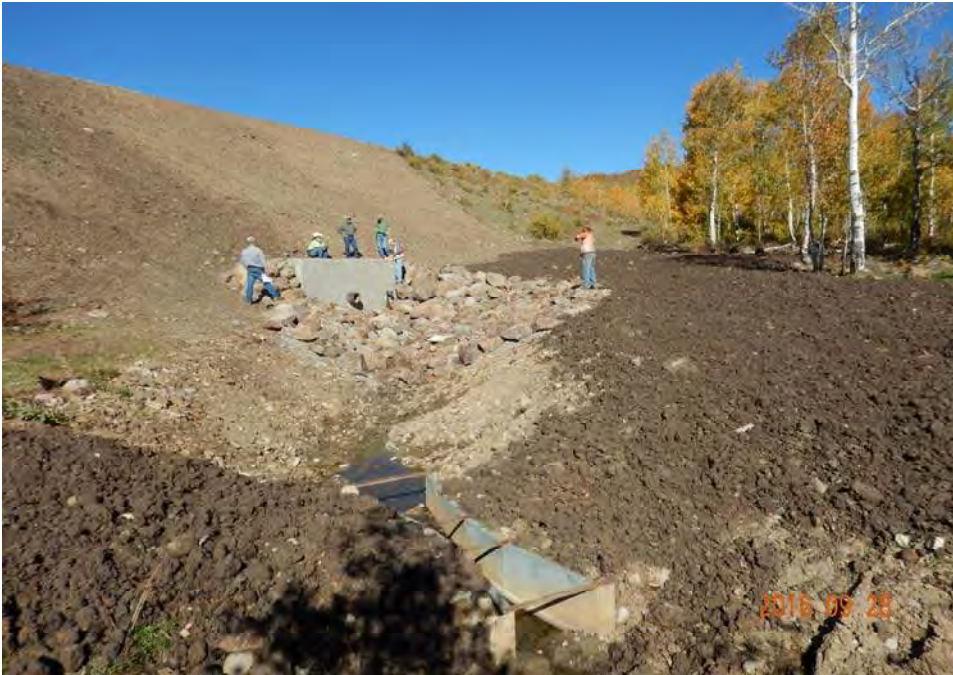
Photograph 41: Downstream headwall, discharge channel, and Parshall flume.
