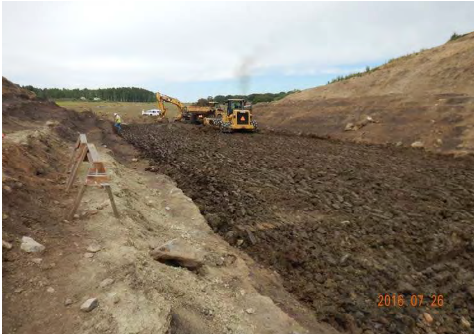
Photograph 11: Placing common fill for the embankment.
