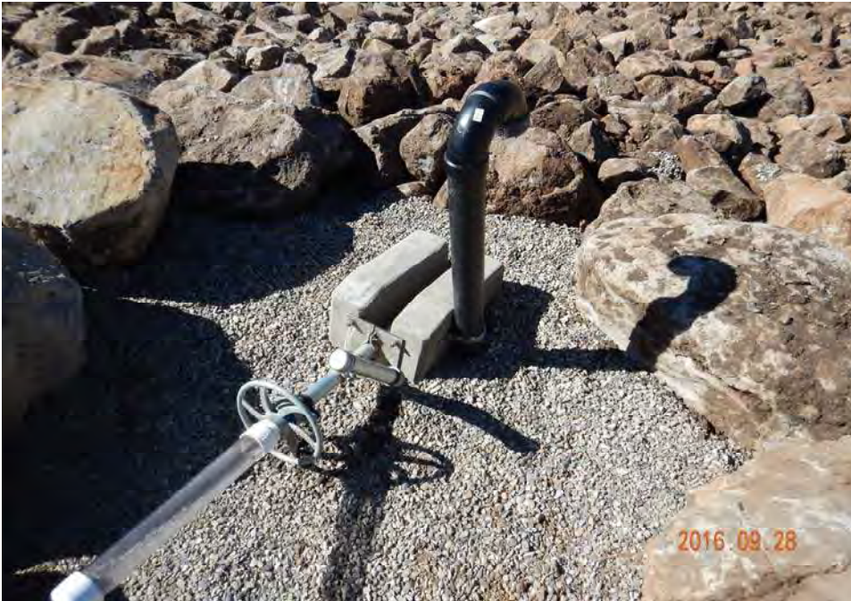
Photograph 39: Hand wheel pedestal on the dam crest. Note the vent pipe, stem cover and fill tube for the stem cover.
