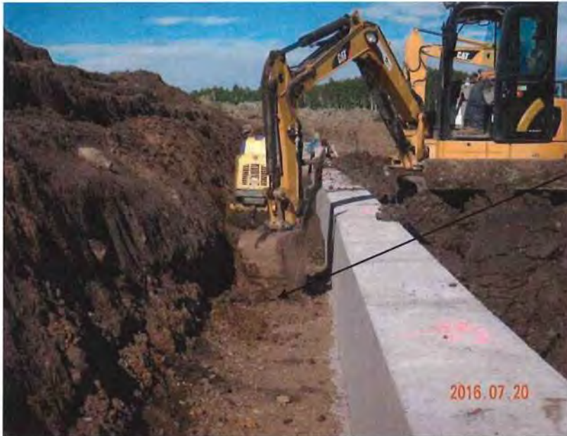
Photo 1 – Scarifying existing embankment before new fill placement.
