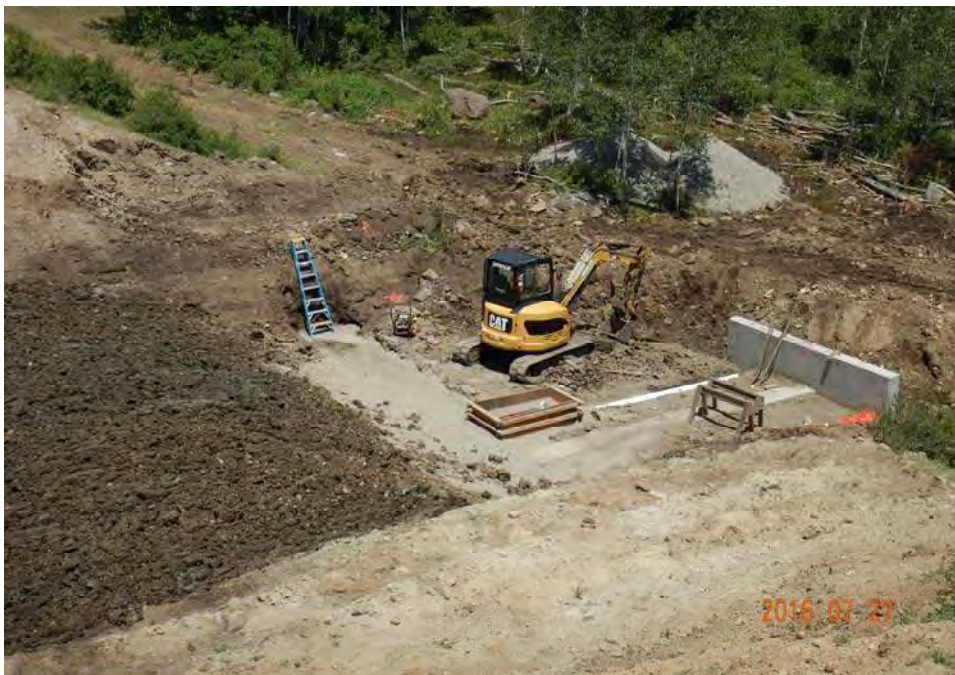
Photograph 20: General view of the filter collar.
