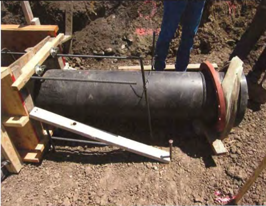
Upstream end of outlet pipe with flanged end for connection to intake structure. Concrete encasement of this section of pipe will occur at a later date.
