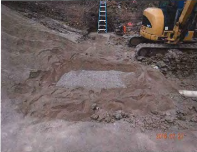
Photo 5 – Filter collar with forms removed.
