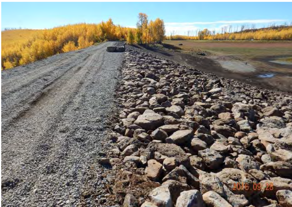
Photograph 48: Riprap on the upstream, slope from the left abutment.
