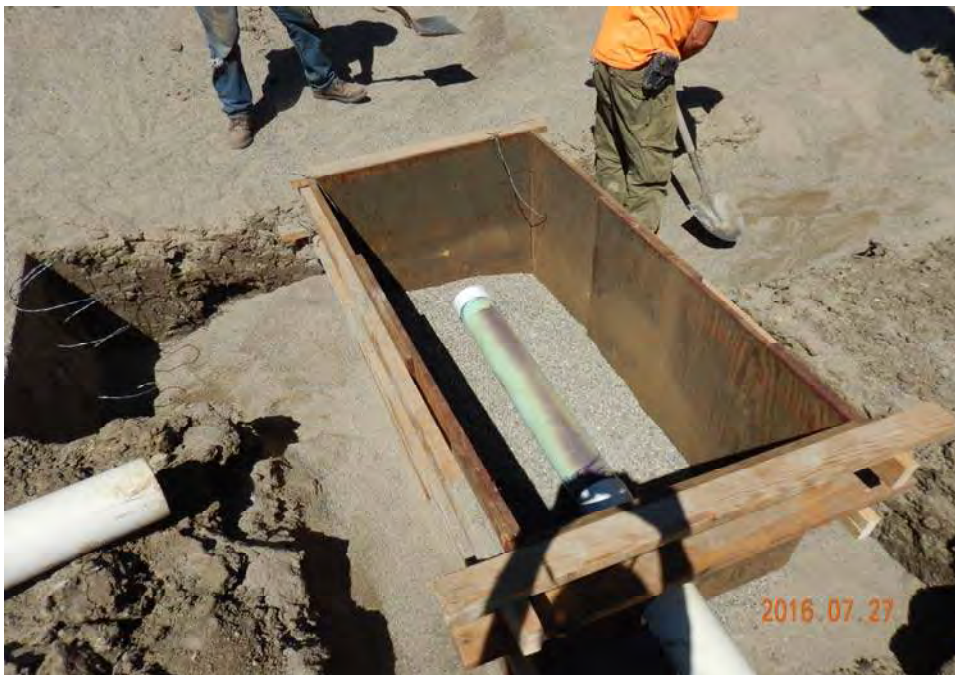
Photograph 18: Forms used to separate the filter sand and filter gravel for the filter collar drain pipe.
