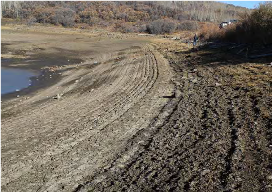
Photograph 1: Upstream slope prior to the start of excavation.
