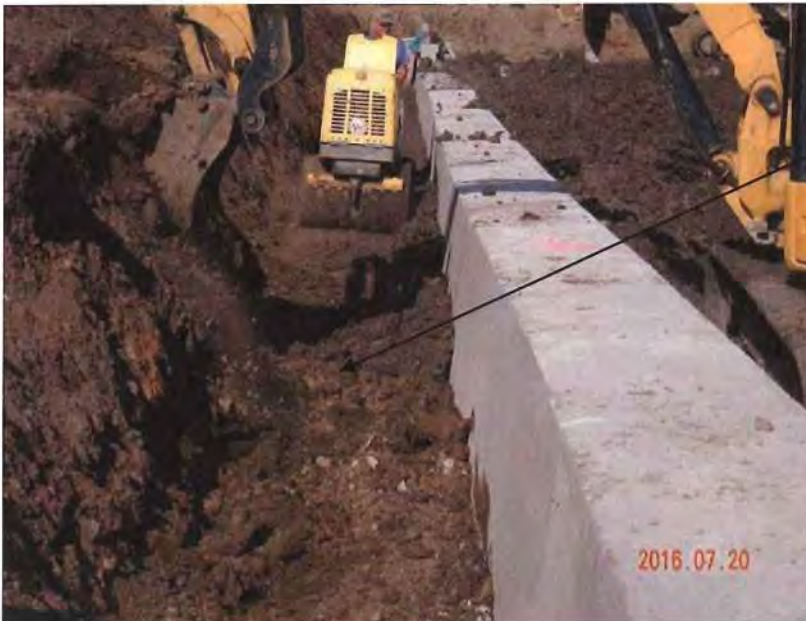
Photo 2 – Excavating existing embankment for use as backfill on the south side of the conduit encasement.
