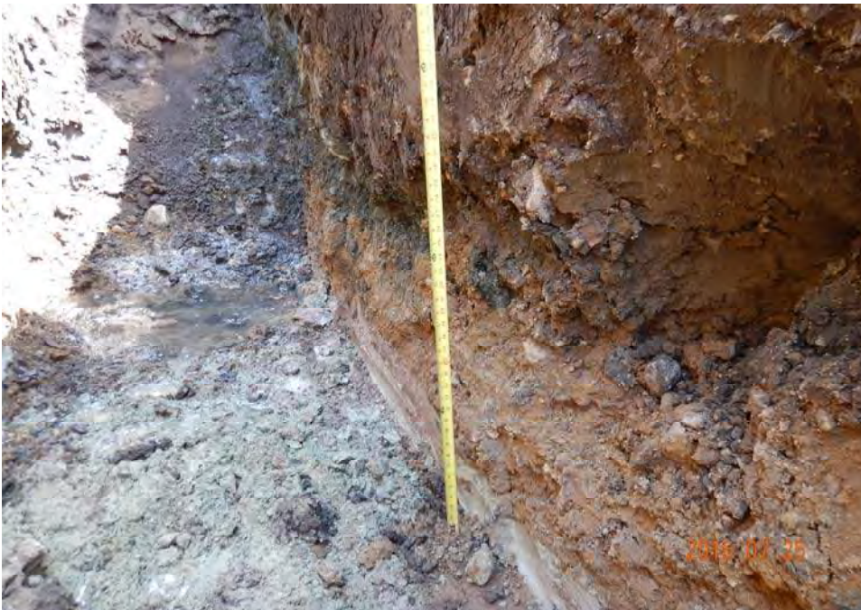
Photograph 16: Filter collar overlap between existing material and new fill.
