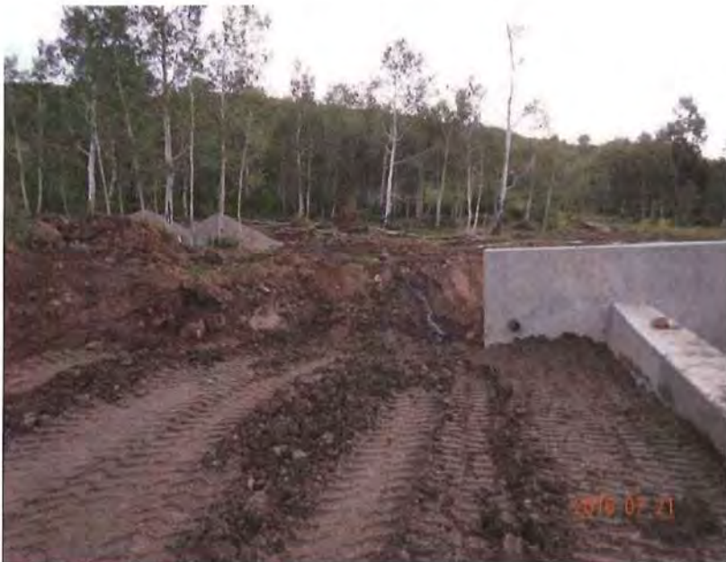
Photo 2 – Fill placement north side of headwall.
