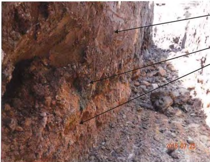
Photo 2 – Excavation for the filter collar.
