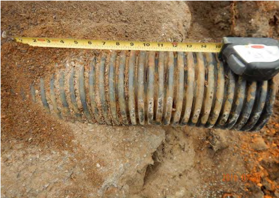
Photograph 21: Existing embankment toe drain pipe on the left side of the energy dissipation structure (not part of this construction).
