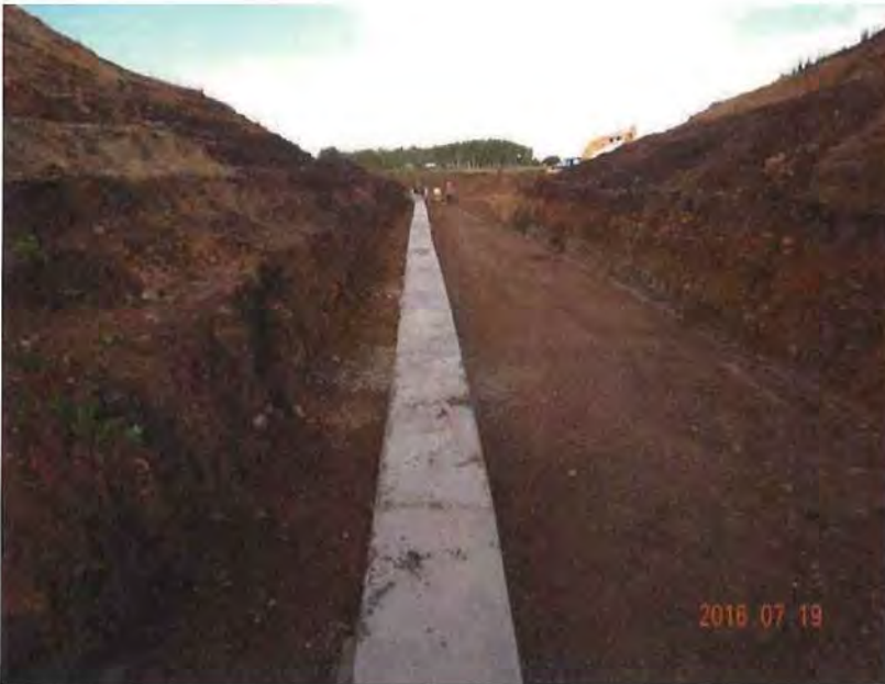
Photo 2 – Outlet works encasement and adjacent subgrade.
