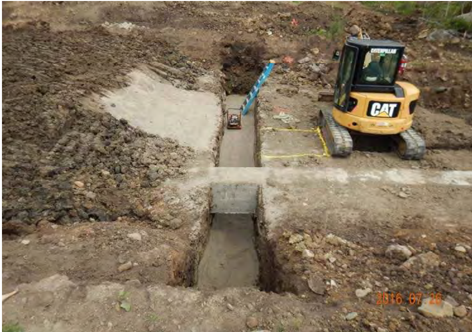
Photograph 17: Placing sand for the filter collar.
