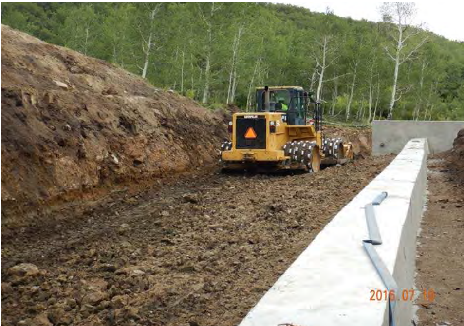
Photograph 8: CAT 815 compacting common fill for the embankment.
