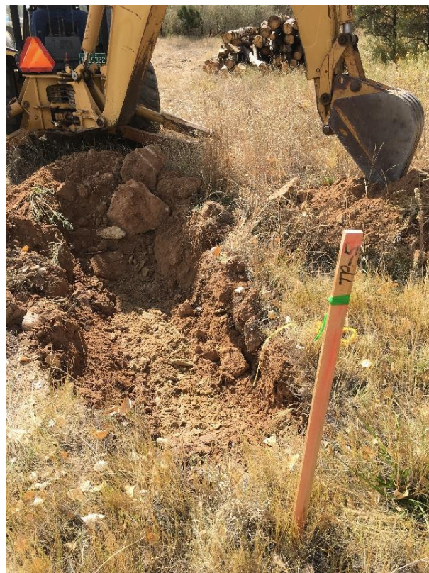
TP- 5: Test pit excavation.
