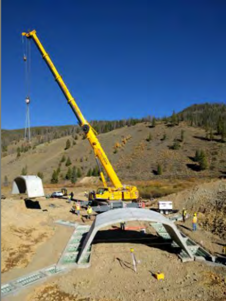
Installation of new crossing span segments
