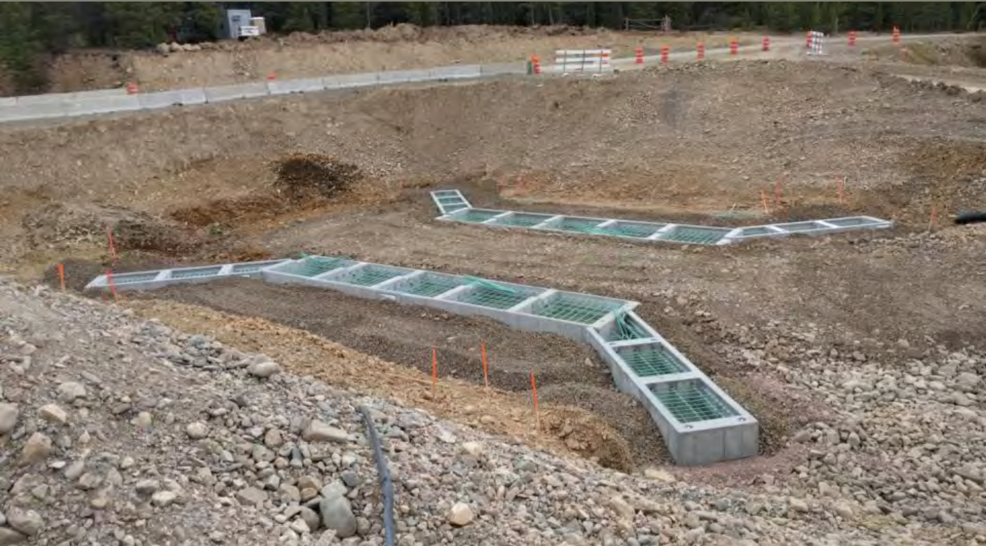
Footing installation for new stream crossing
