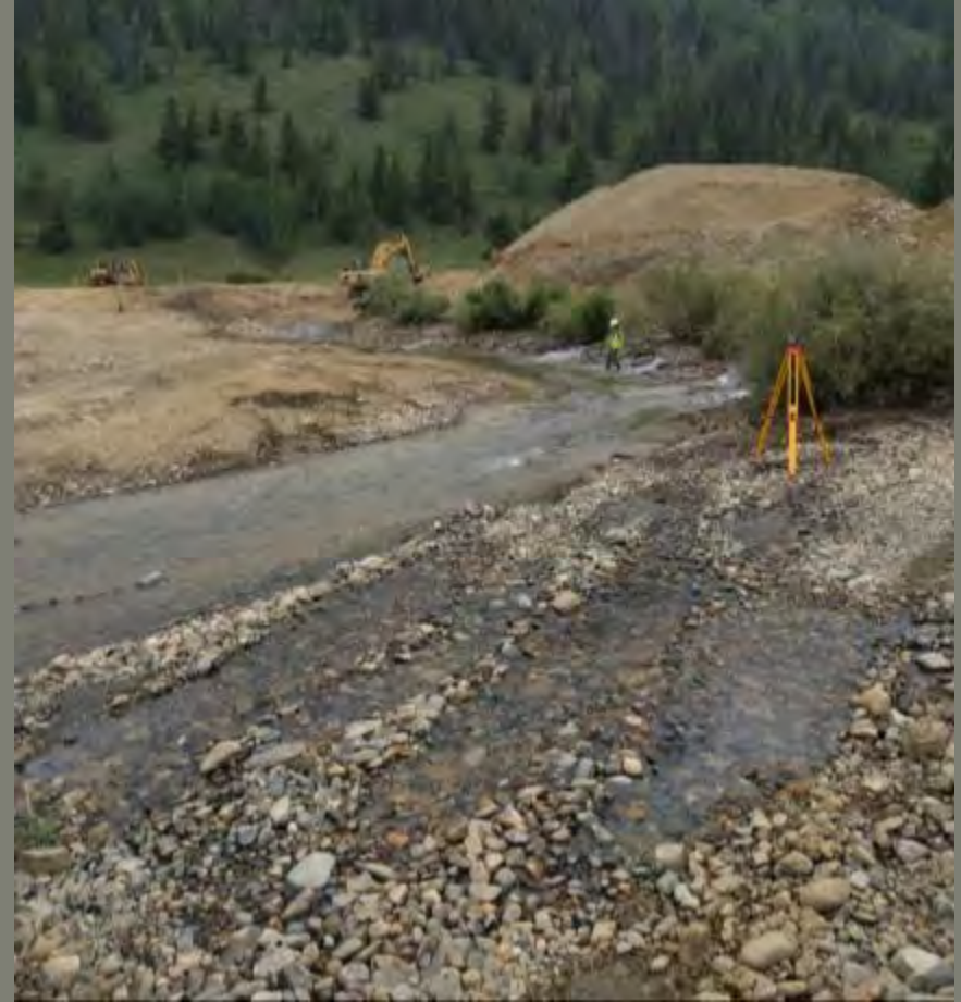
Channel and in-stream structure construction; willow transplants installed on new stream banks
