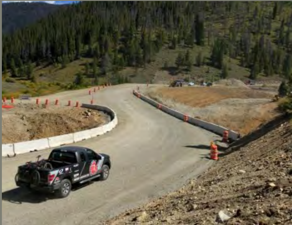
Detour installed in order to construct new stream crossing
