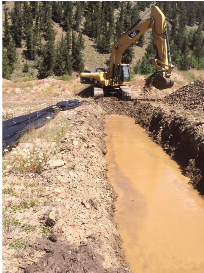
Photo 1 – Excavated Trench Prior to Deploying Geotextile
