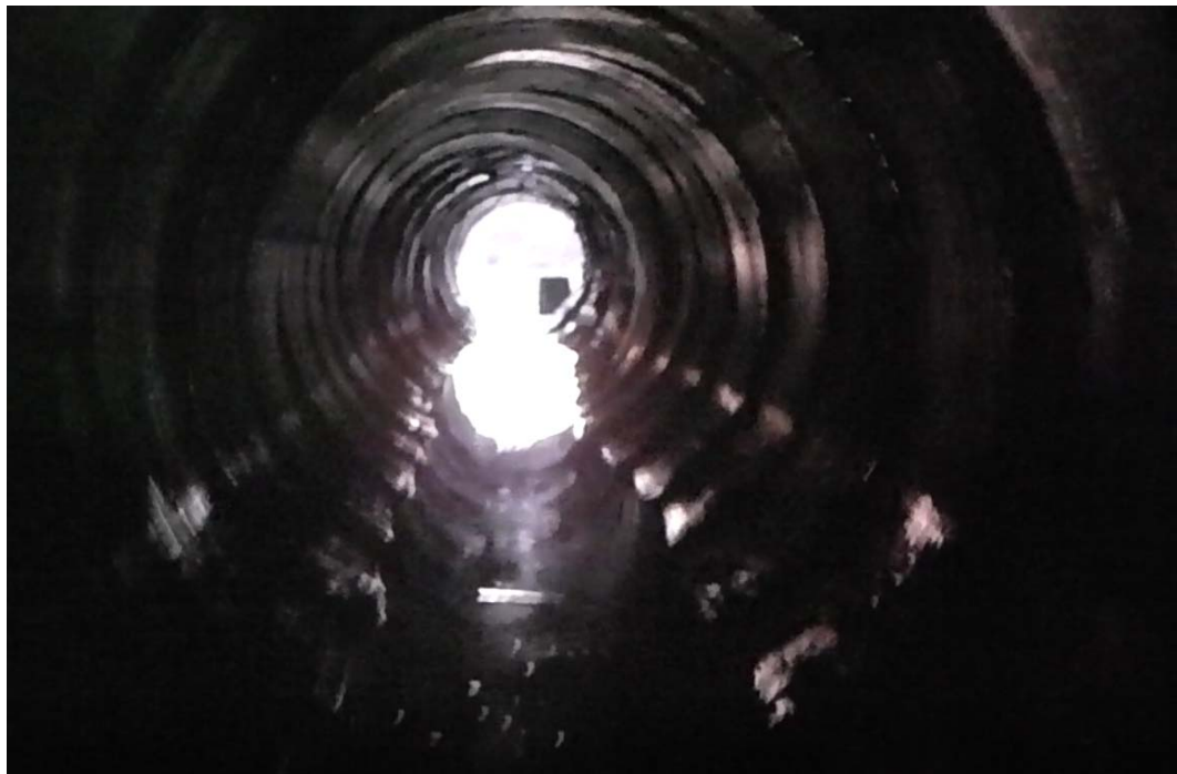
Screenshot 10: View looking downstream in Conduit No. 4 at Station 0+35 downstream of gate. View shows disjointedness and movement of pipe sections. November 9, 2016.
