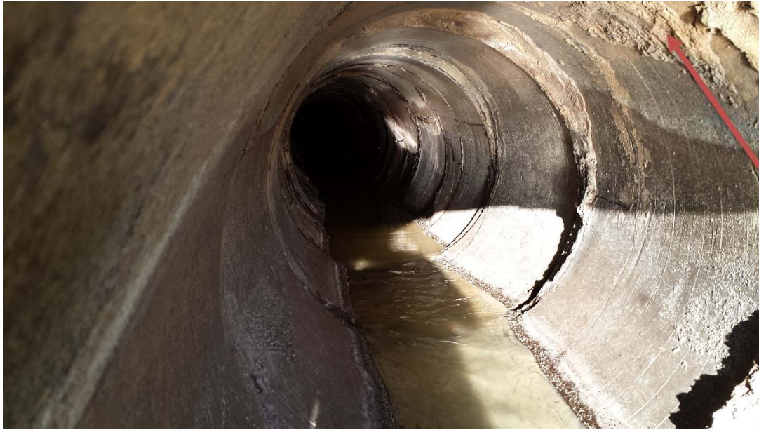
Photo 7: View of Conduit No. 3 taken from the discharge end looking upstream. Note lateral offset of joints and cracking in pipe. November 9, 2016.
