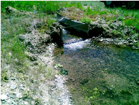
Photo 4: Unstable and inaccurate flume from lack of wingwalls and toewall.
