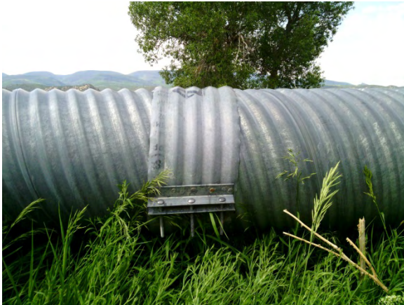
Photo 1: Leaking piped joints.
