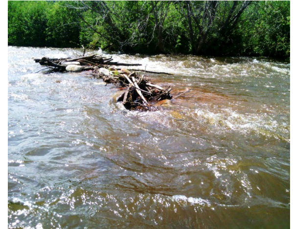
Photo 3: Ineffective diversion structure with hazardous tarps in creek .
