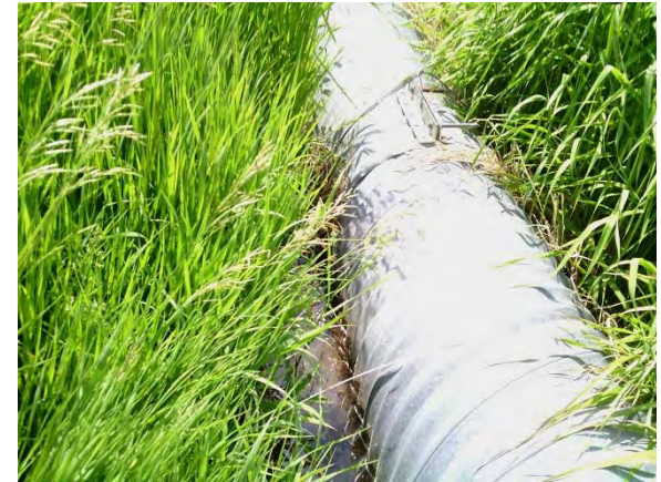
Photo 3: Rusty out and leaking culvert.
