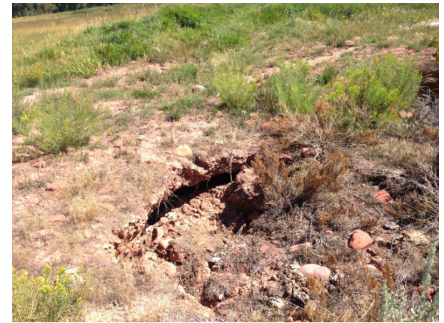
Photo 6: Sinkhole located above a ditch due to underlying salty soils.
