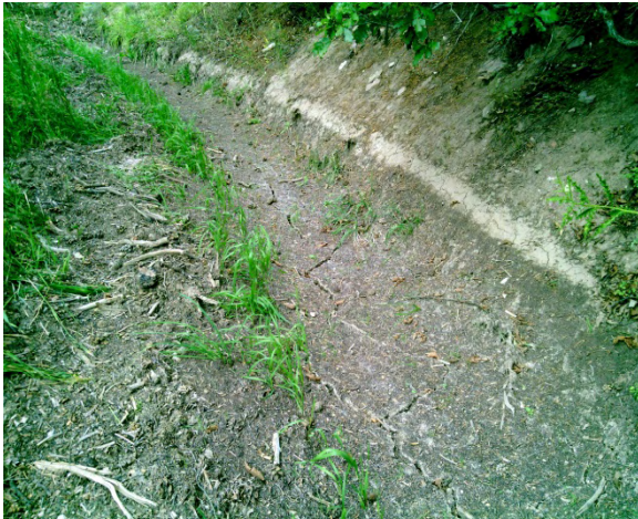
Photo 1: Sediment filled ditch from unstable upgradient watershed.
