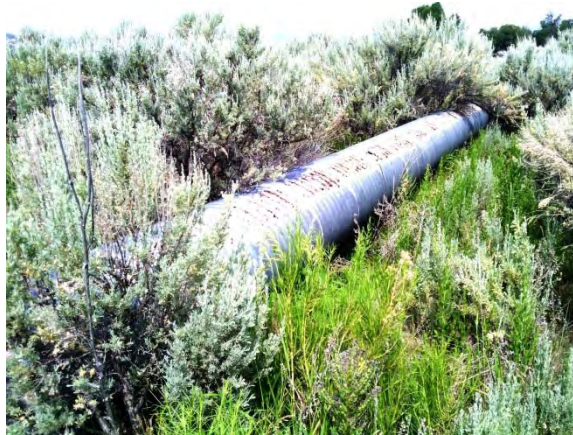
Photo 2: Rusty culverts being rotated to extend useful life.
