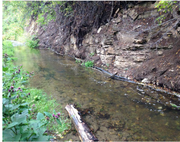
Photo 2: Approx. 2 cfs leak in ditch through liner damaged by rock fall.
