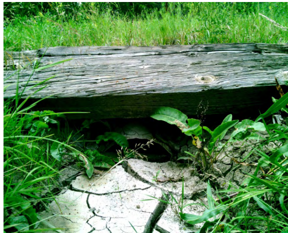
Photo 4: Sediment filled culvert from highly soils in watershed.
