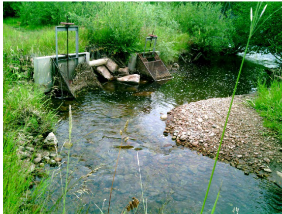
Photo 5: Unstable and unsafe headgates from erosion around structures.
