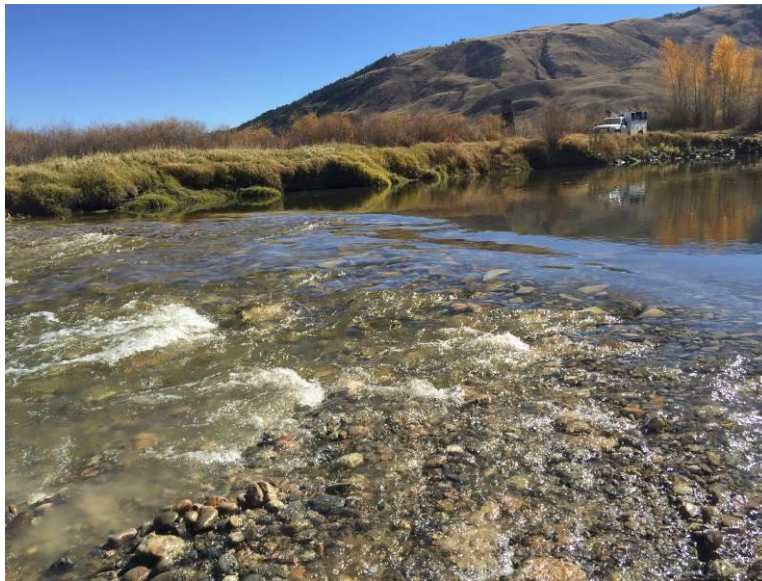
Figure 12. TA Engle Engineered Riffle Grade Control Structure
