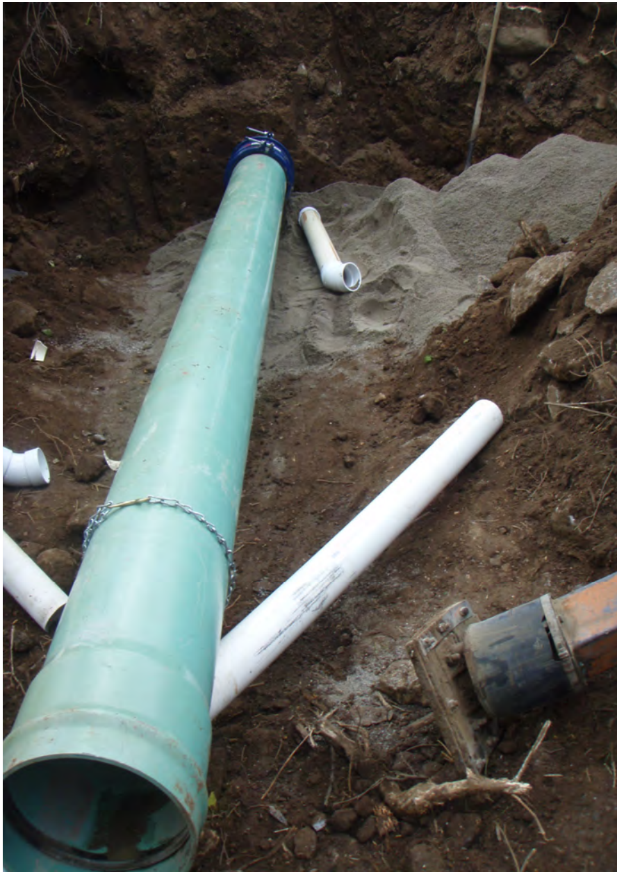
Downstream Pipe Extension
