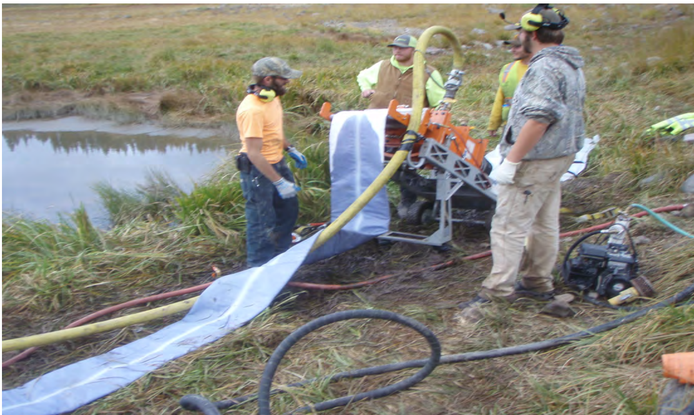
Liner Connected to Shooter
