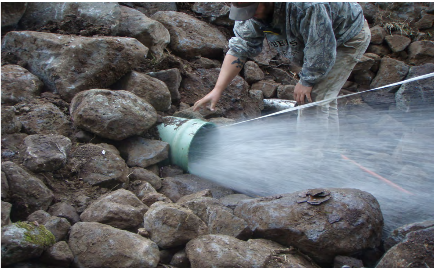
Cleaning Outlet Pipe Prior to Lining
