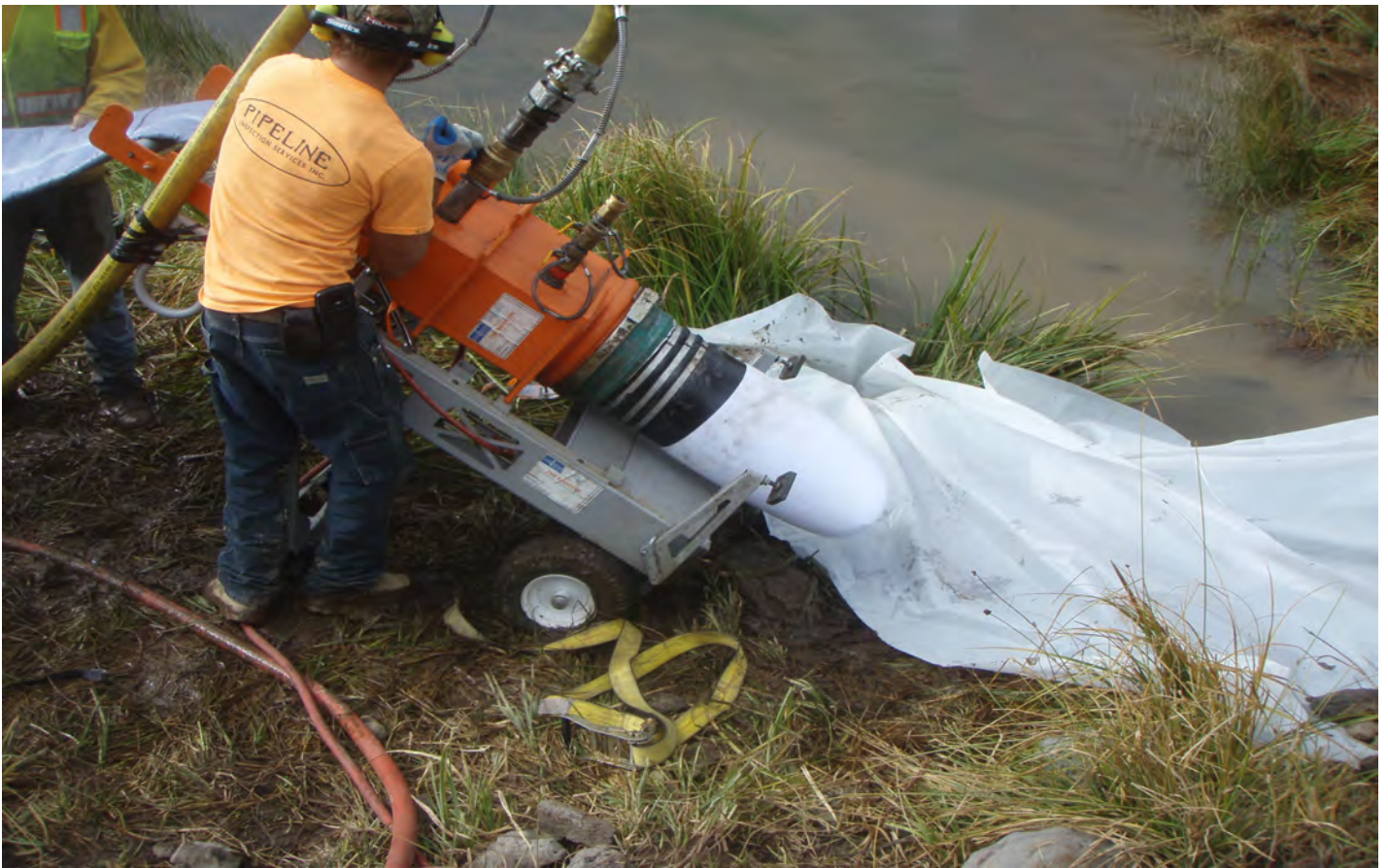
Liner Shooter Connected to Outlet Pipe
