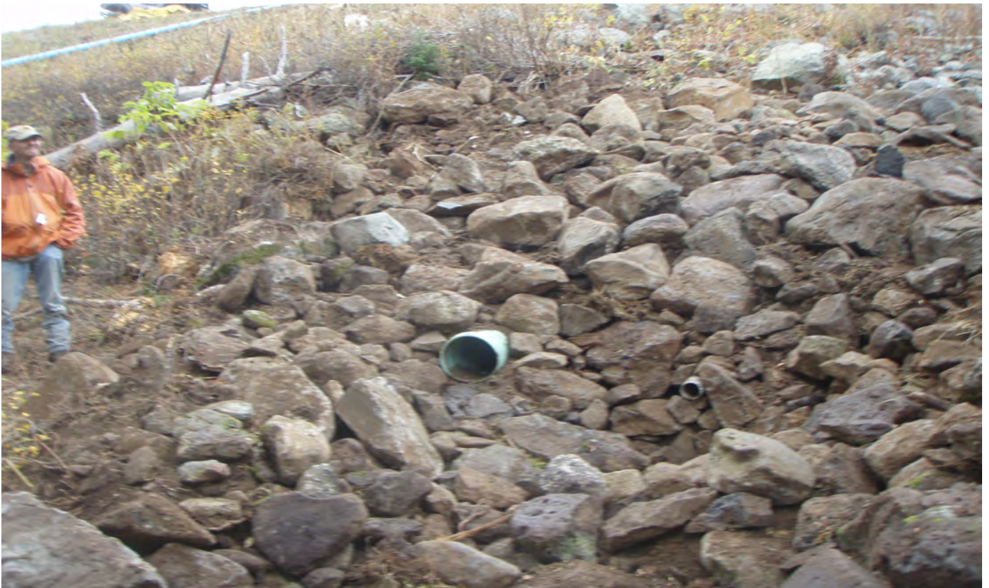
Completed Downstream Dam Embankment and Armoring Rip Rap
