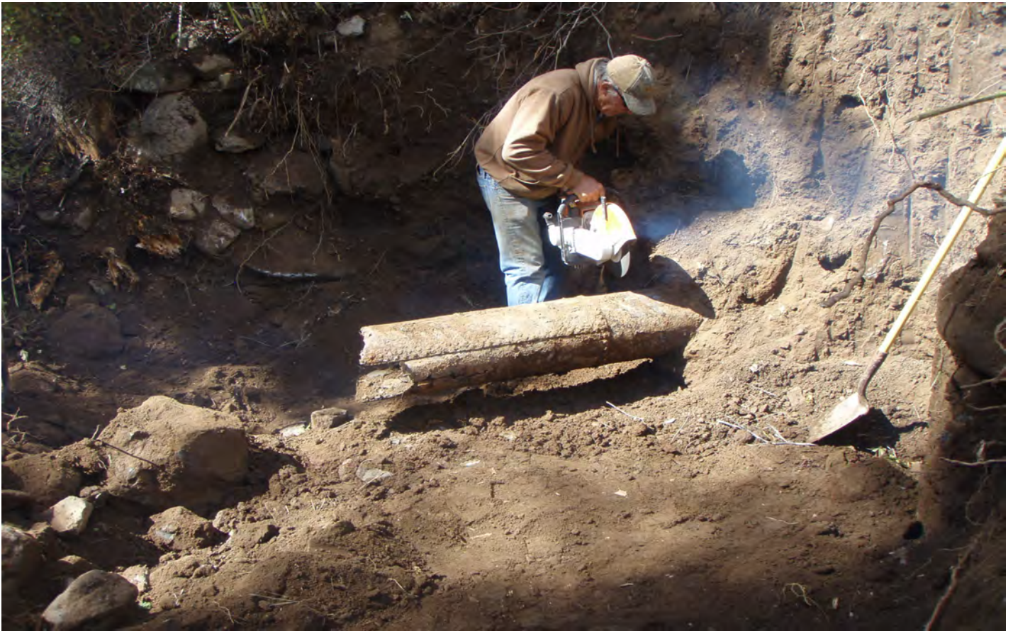
Cutting Downstream End of Original Outlet Pipe
