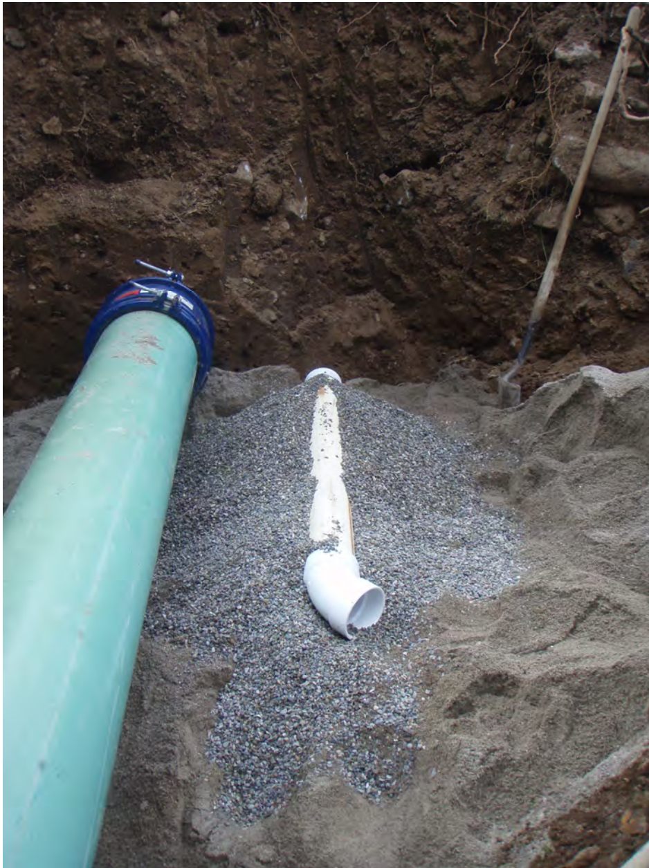
Diaphragm Filter Drain Slotted Pipe
