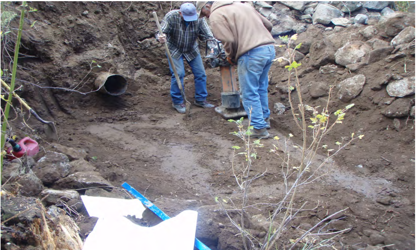
Compacting Downstream Outlet Excavation Subgrade
