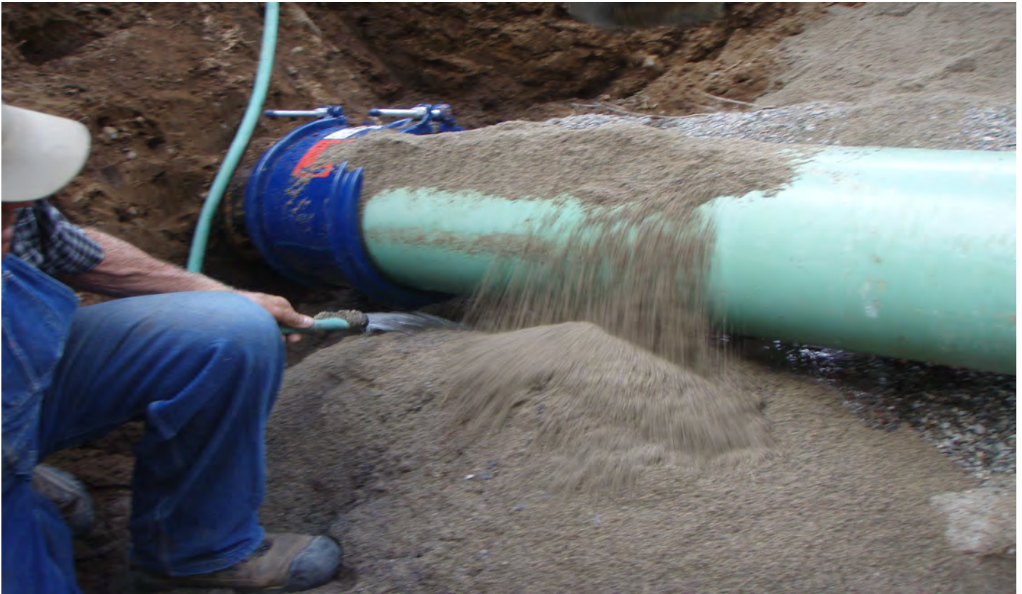
Wetting Diaphragm Filter Sand
