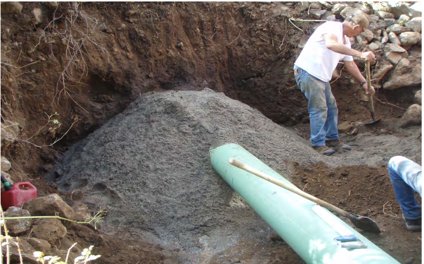
Completed Downstream Diaphragm Filter
