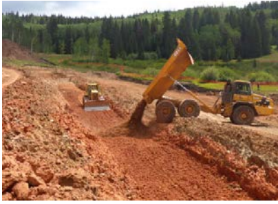
Figure 1 - Dam Embankment Construction
