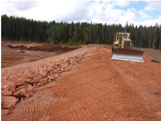
Figure 4 - Riprap Placement
