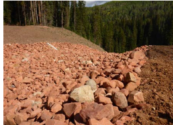
Figure 5 - Spillway Channel Riprap Armoring
